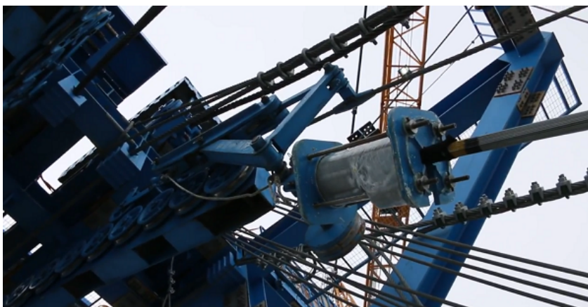
Video: Strand pulling over the saddle
