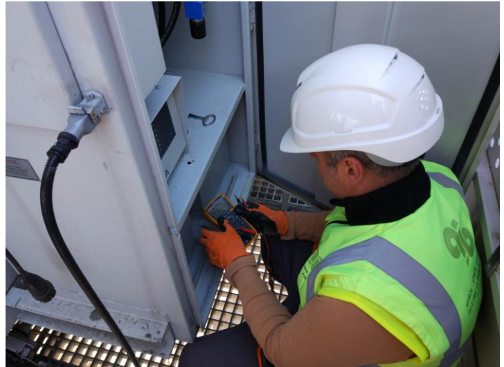
Figure 8: Routine inspection of accumulator of deck gantry man lift
