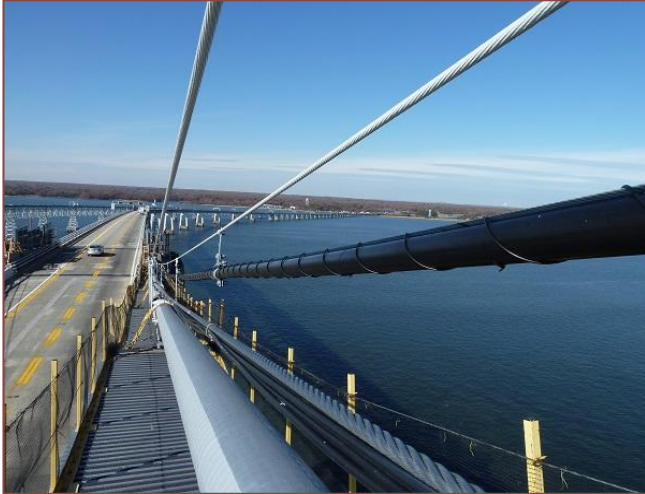
Figure 22. HDPE dry air supply pipework
