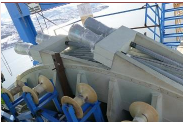
Figure 21: Anchorage of back strands at the tower saddle
