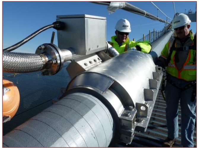
Figure 24. Cable injection sleeve (note sensor box on top)
