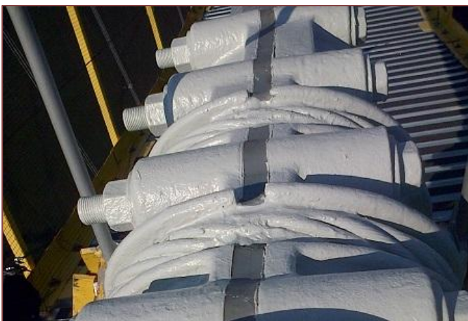
Figure 14 ←: Westbound Bridge cable band longitudinal gap with new caulk sealant
