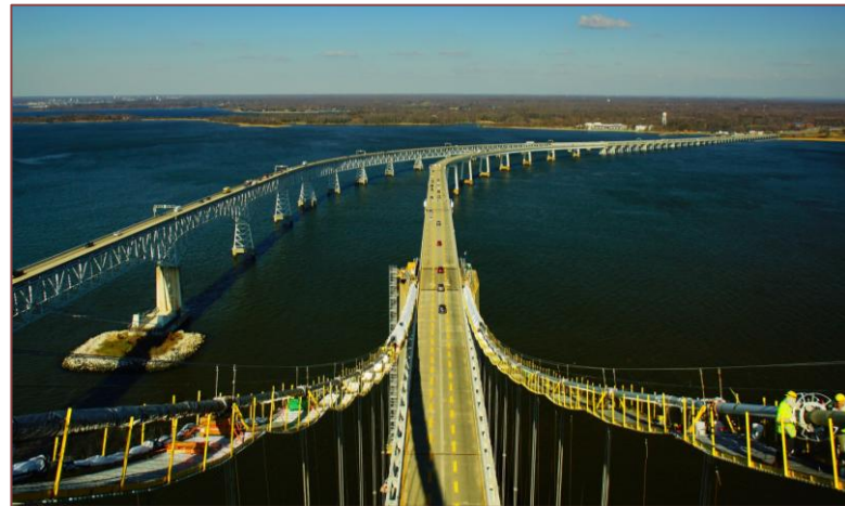
Figure 27: Main cable access platform; Westbound Bridge shown, Eastbound Similar (Photo Credit: Christian Christodoulou, AECOM)
