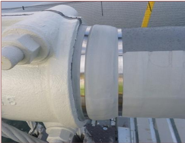
Figure 13: Finishing strip at cable band interface
