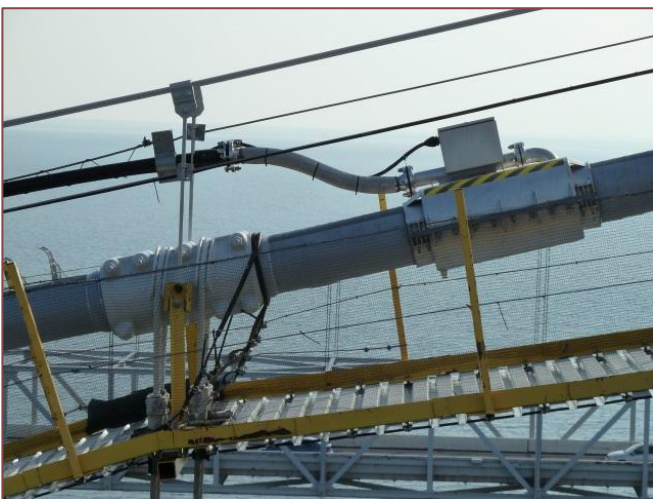
Figure 23. Flexible stainless steel pipe transition to injection sleeve
