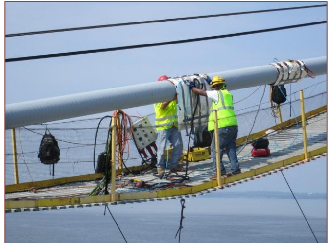
Figure 11: Inflatable heating blankets used to seal the cable wrapping
