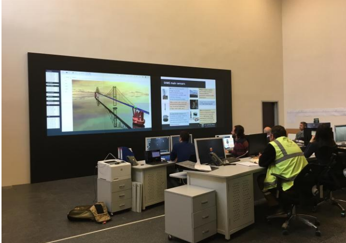
Figure 17: Bridge Control Center Scada Wall
