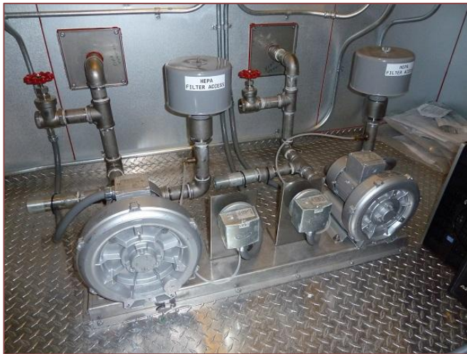
Figure 20: Injection fans with HEPA filters
