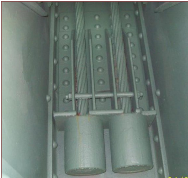
Figure 5: Typical suspender socket detail on a US suspension bridge
