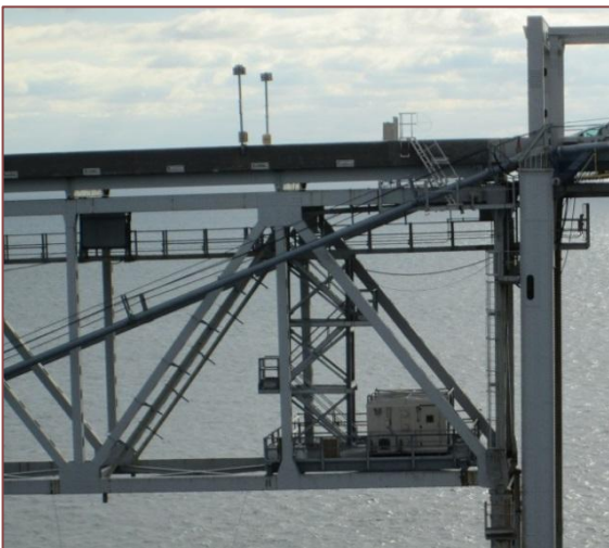
Figure 7: Eastbound plant room on platform; backstay and approach span on left, suspension span on right
