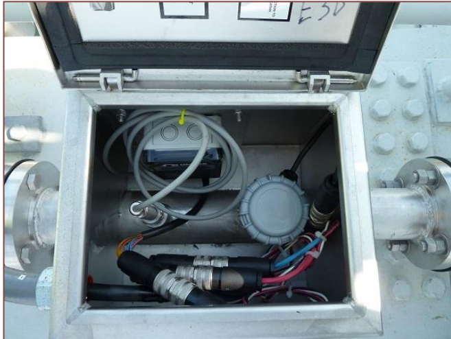
Figure 25: Sensors in NEMA 4X sensor box
