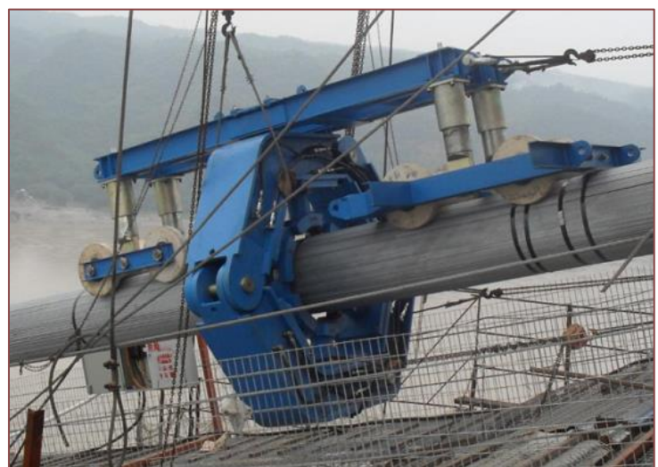
Figure 22: Compacting of the main cable
