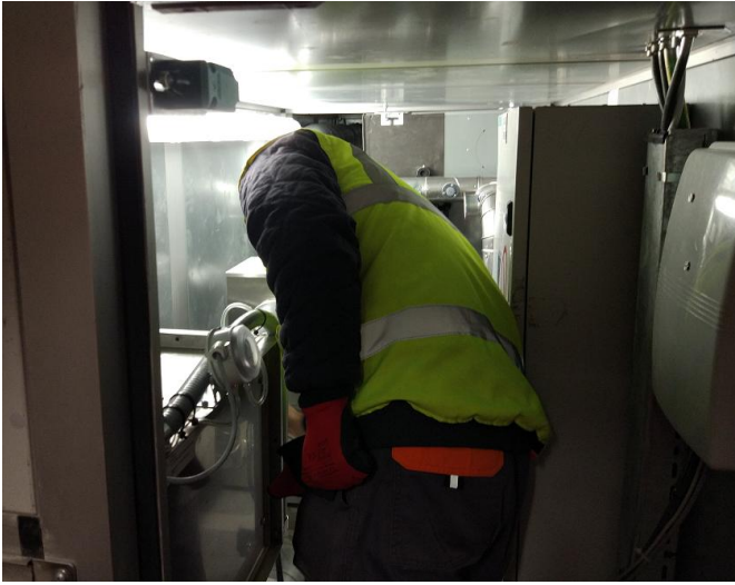
Figures 11 + 12: Routine inspection of dehumidification pipes at South Anchorage Block Back Chamber East
