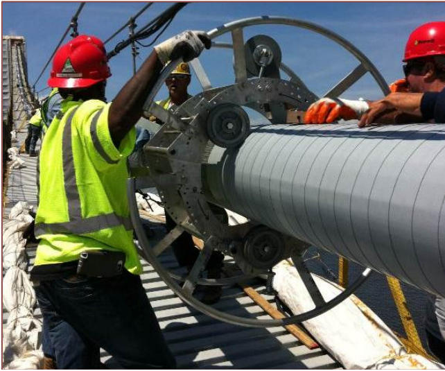
Figure 9: Cable wrap being spirally wound using a wrapping device (Skewmaster™)
