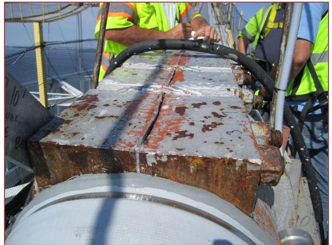
Figure 15: Eastbound cable band gap filled with lead sealant
