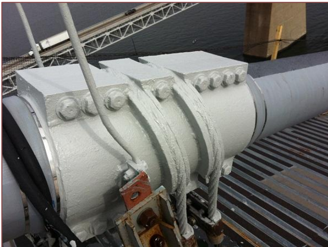
Figure 17: Eastbound cable band with new elastomeric acrylic coating system
