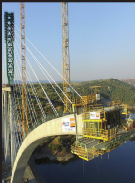
VIADUCT OVER TAJO RIVER (HSR - SPAIN) Pair of tri-hinged formwork travellers for compressive arch construction (324 m free span)
