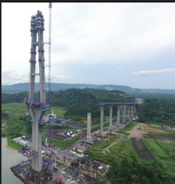
ATLANTIC BRIDGE (PANAMA) 4 No. R-1900 series form travellers for the construction of a cable stayed bridge -Assembly stage-
