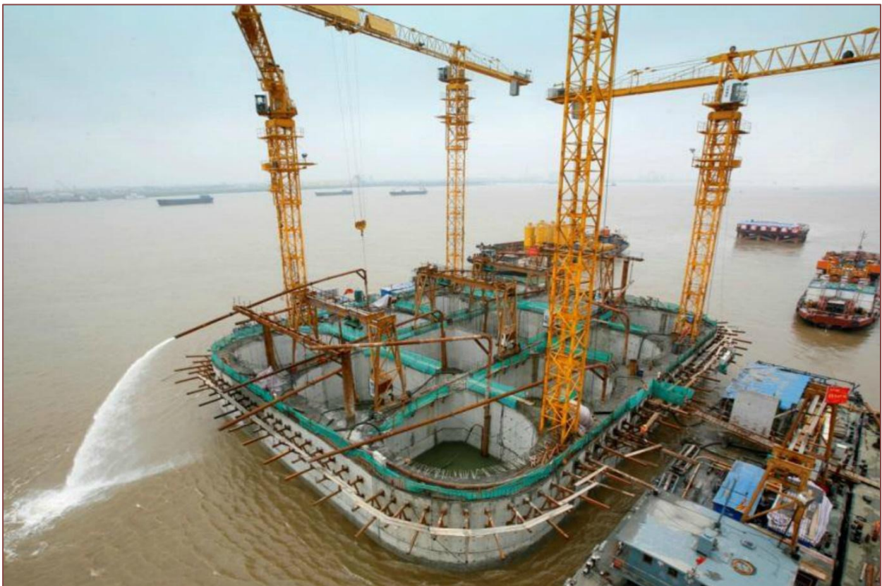
Figure 12: River caisson for the Taizhou Bridge 3
