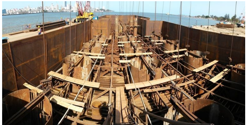
Piles of the South Pylon
