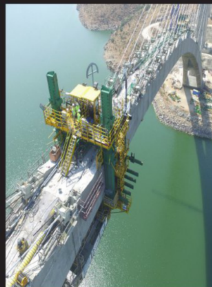
RAILWAY ARCH BRIDGE OVER ALMONTE RIVER (HSR - SPAIN) Special equipments (4 formwork travellers) for the execution of the arch bridge (384 m free span)
