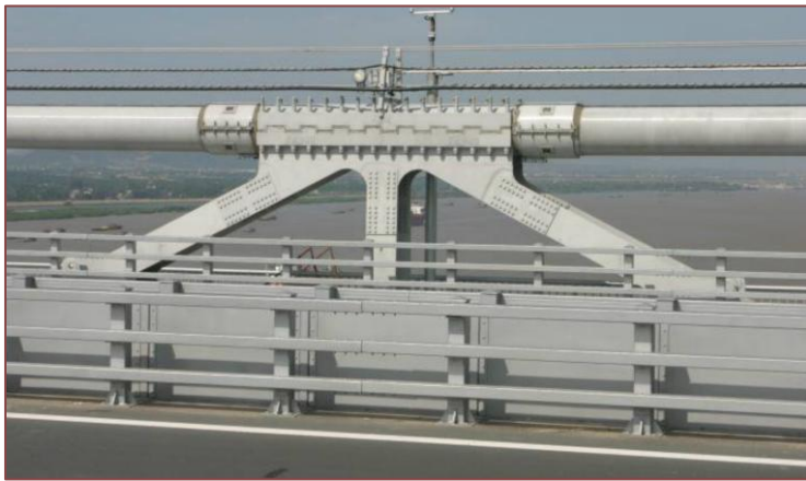
Figure 9: Cable clamp on the Runyang Yantze Bridge 3
