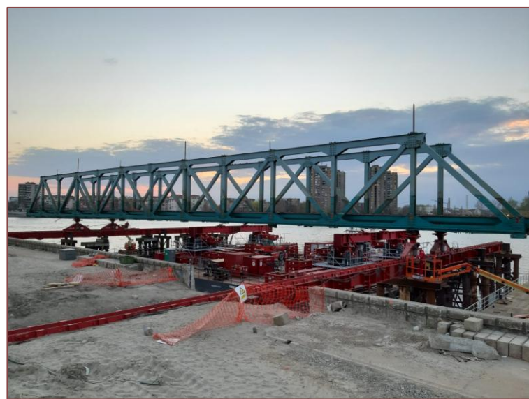
Figure 11: Span in the skidding process to land
