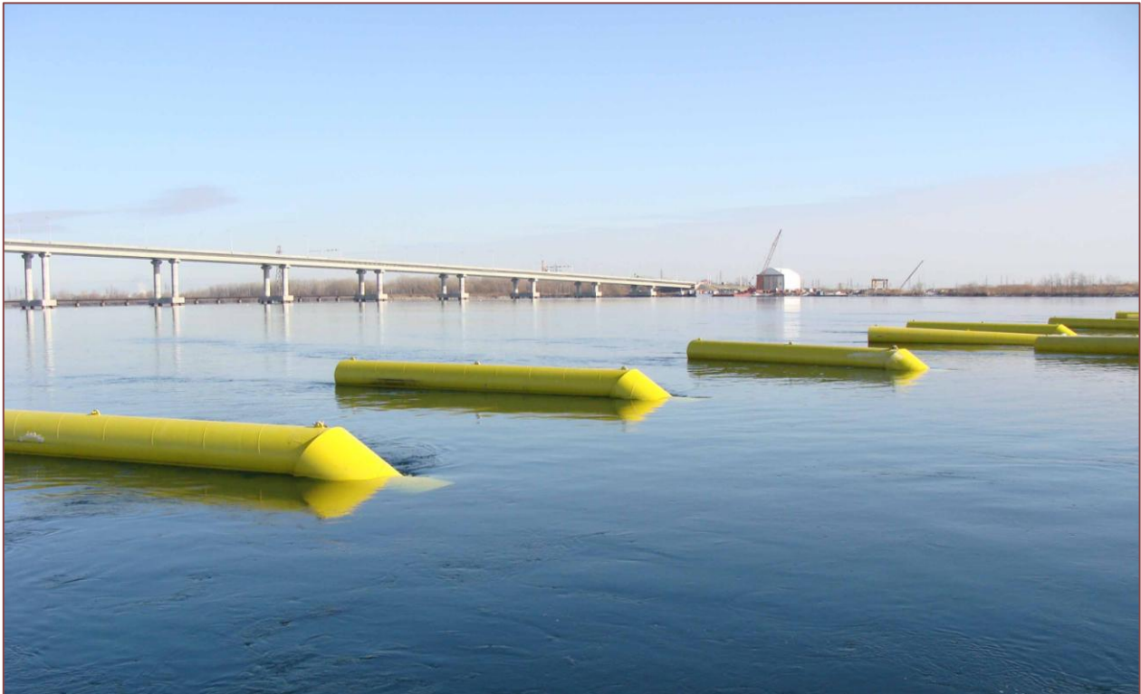
Figure 1: Ship Arrest Boom pontoons just upstream of the A30 Bridge
