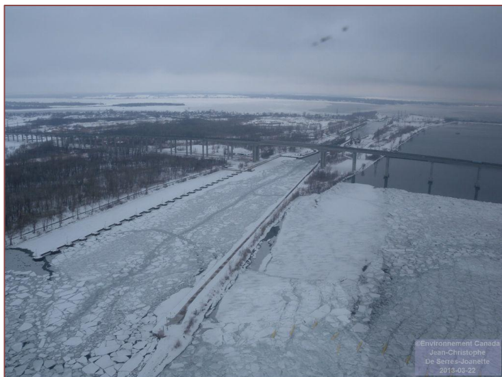
Figure 4: The Ship Arrest Boom allowing the ice to pass and collect on the Ice Boom downstream
