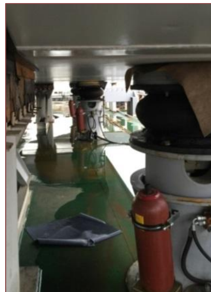
Figure 10: A buffering system was designed and used during lifting operations at site in order to avoid undesired movements and damage to either the transportation vessel or the deck segment
