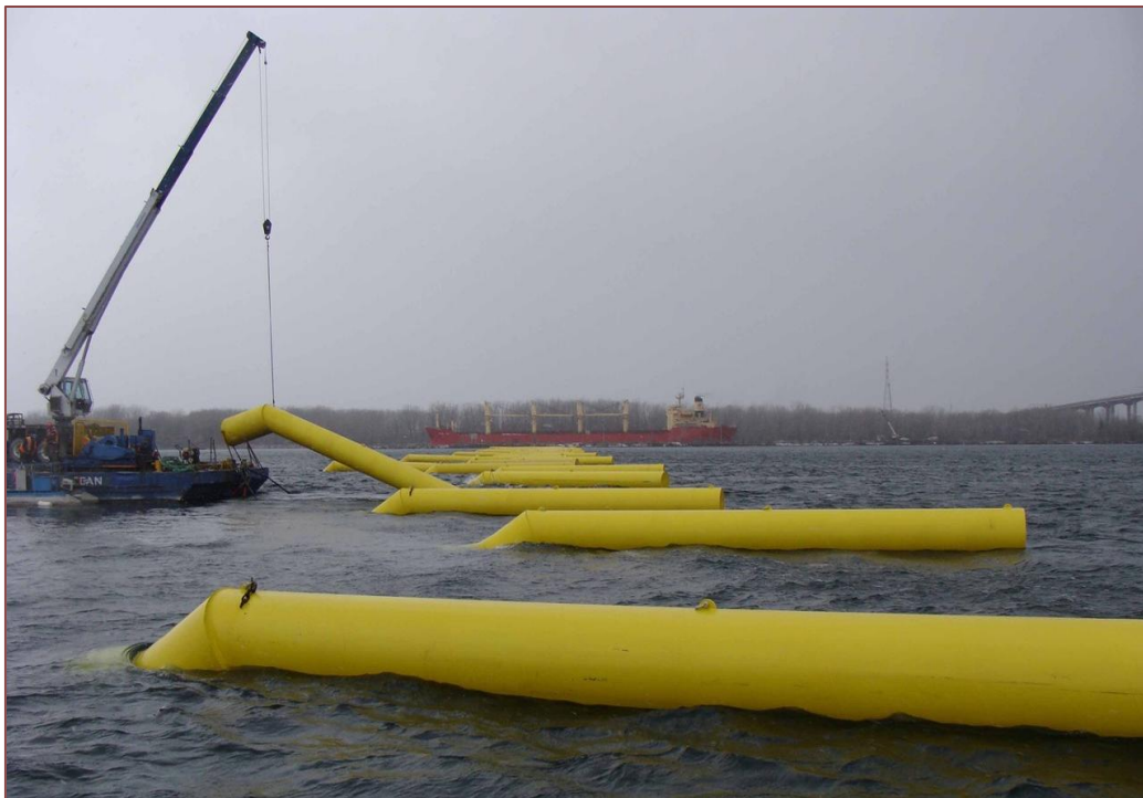
Figure 3: The final pontoon of the Ship Arrest Boom being installed as a ship passes by through the canal
