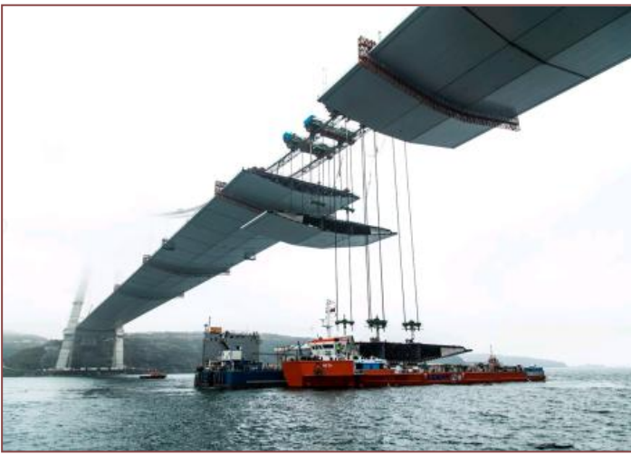
Figures 11 – 14: Positioning of the additional non-propelled barge by M/V Neta using the tension controlled hydraulic mooring system, and delivery of two deck segments simultaneously
