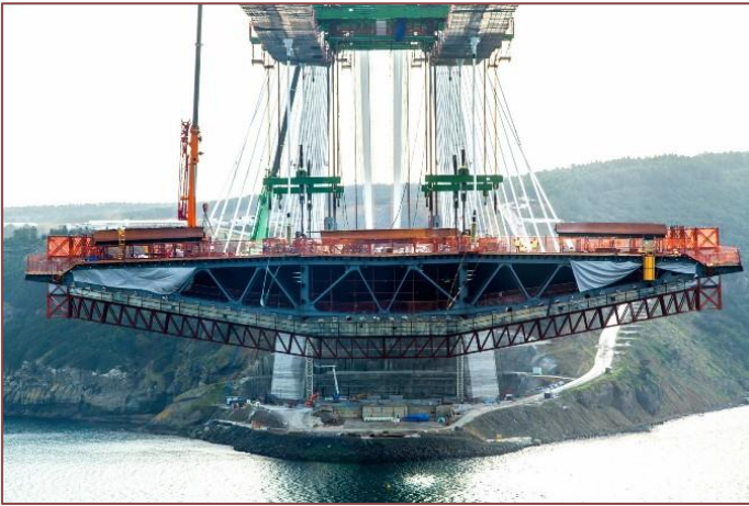
Figures 15 – 18: Deck segments transportation and lifting
