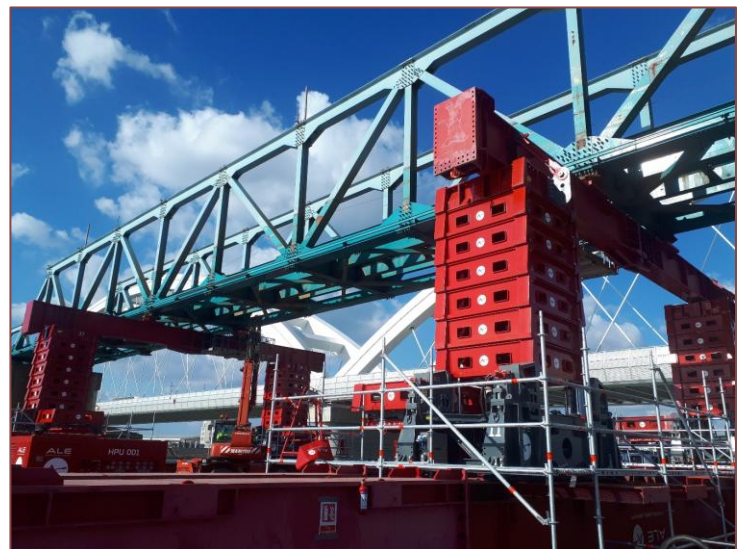
Figure 7: Taking the load with the ballasting and the jacking towers
