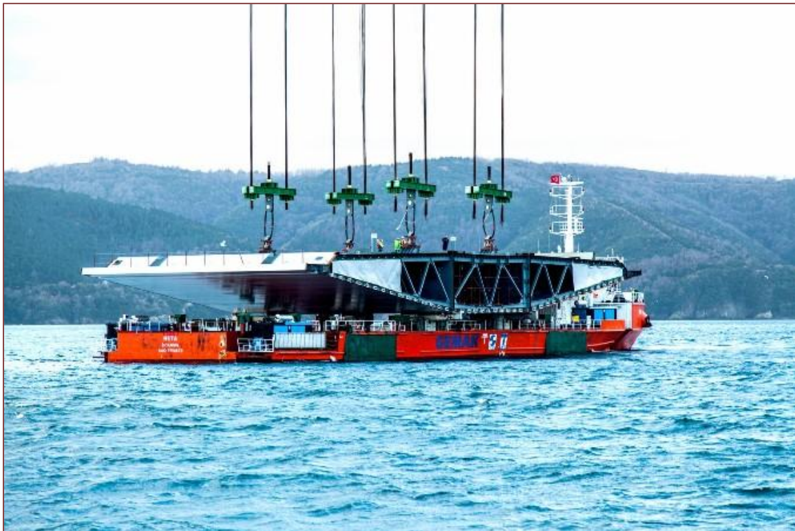
Figure 1: Transport and positioning of deck segments have been executed by DP vessel "M/V Neta"
