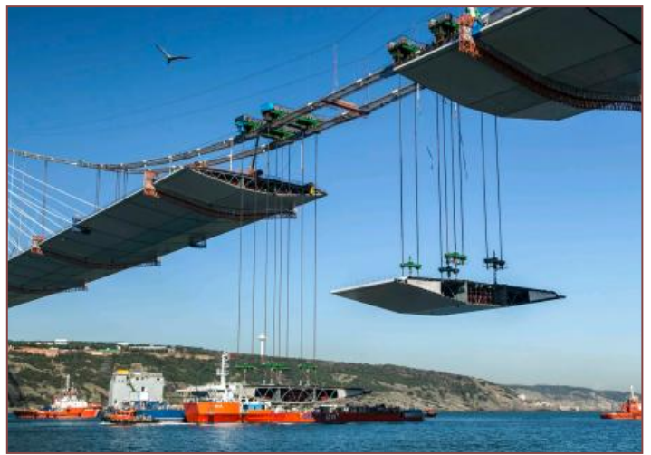
Figures 11 – 14: Positioning of the additional non-propelled barge by M/V Neta using the tension controlled hydraulic mooring system, and delivery of two deck segments simultaneously
