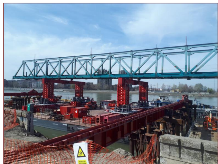
Figure 10: Span at the jetty to be downloaded
