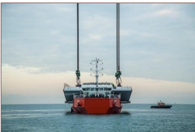
Figure 9: Lifting instant of deck segment from M/V Neta
