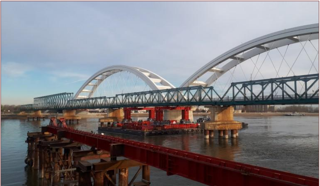
Figure 1: Civil bridge removal, Mega Jack 800 in Serbia
