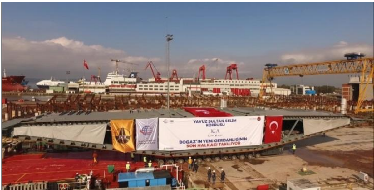
Figure 5: Load out of last deck segment (key segment) at Gemak Altinova Factory
