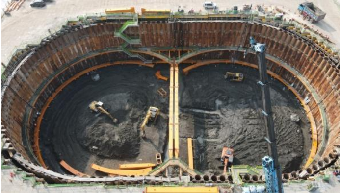
Figures 13 and 14: The cofferdam under construction (left) and upon completion (right)
