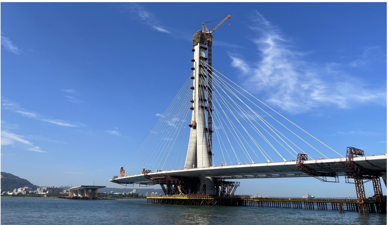
Figure 1: Pylon erection
