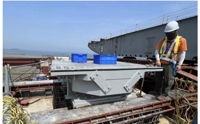
Figure 8: Pendulum bearing at the construction site - preparation before installation
