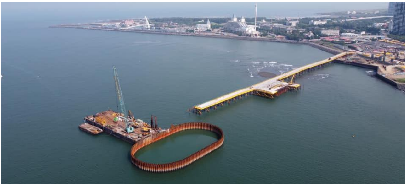
Figure 1: View of the cofferdam during construction
