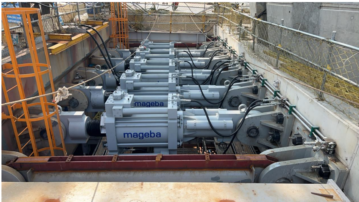
Figure 16: Installed hydraulic fuse restrainers
