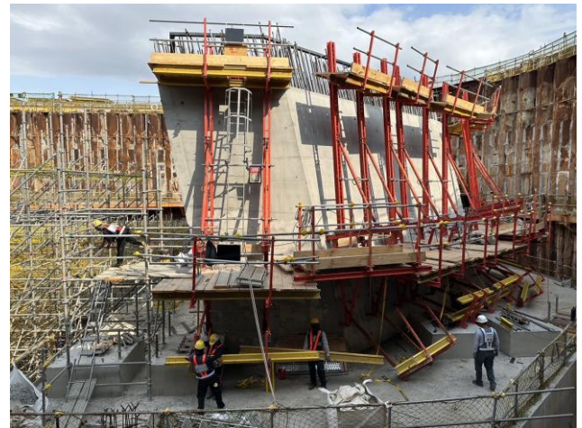
Figure 4: The SCS Climbing System ensures safety by providing horizontal working areas on inclined walls
