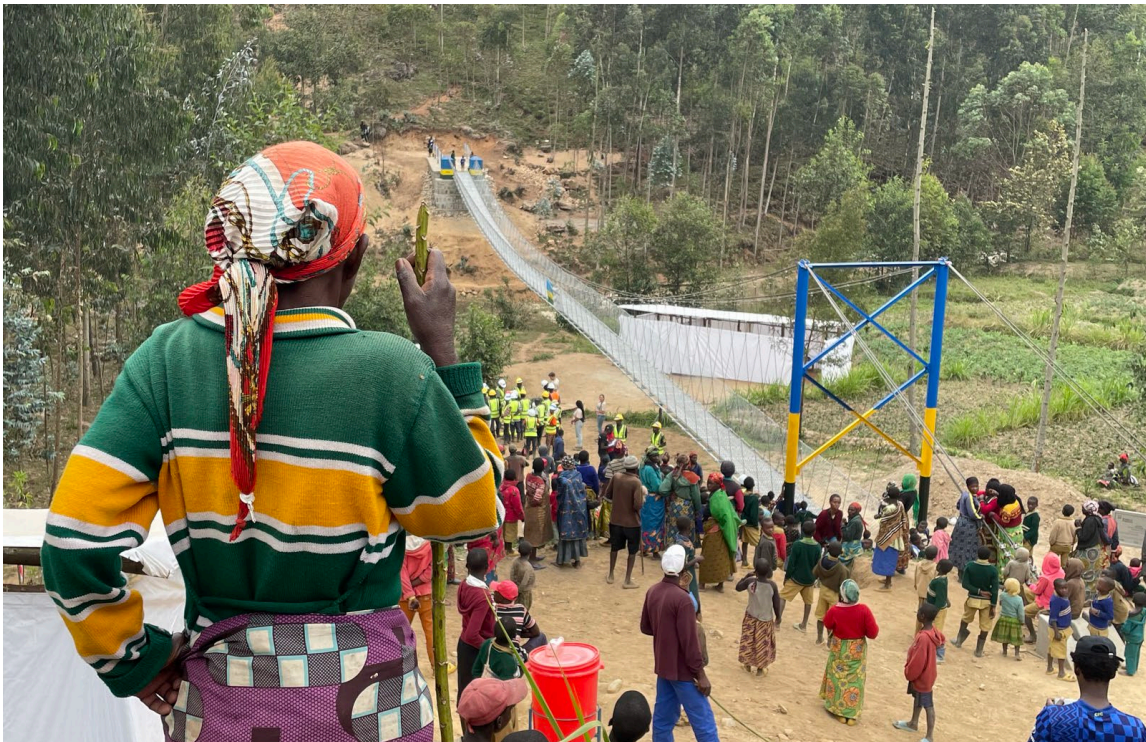
Figure 1: Construction of the Bishenge-Masuma bridge above the Gasumo River
