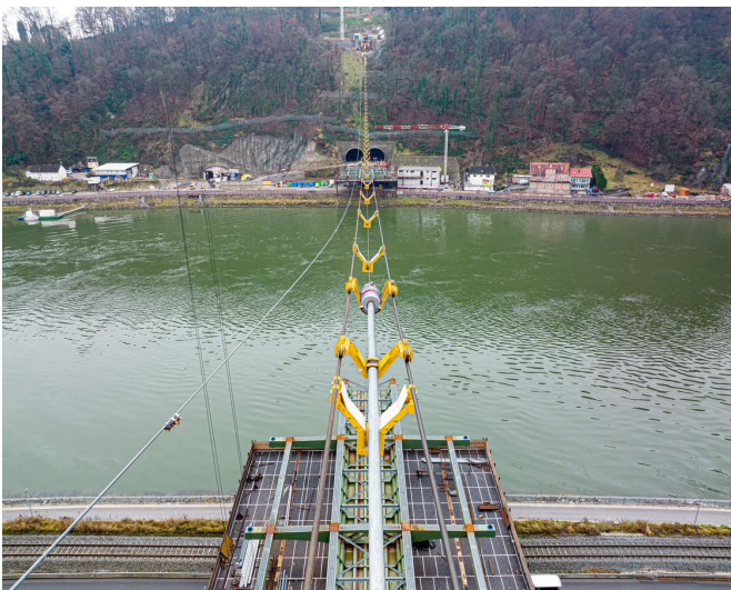
Figure 15: Auxiliary cableway suspension cable installation ASFINAG
