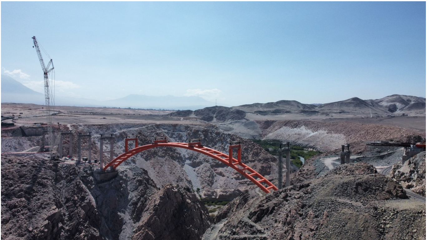
Figure 1: View of the construction site with part of the arch completed
