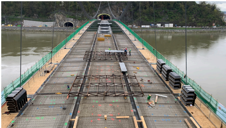
Figure 30: Installation of Precast Slabs
