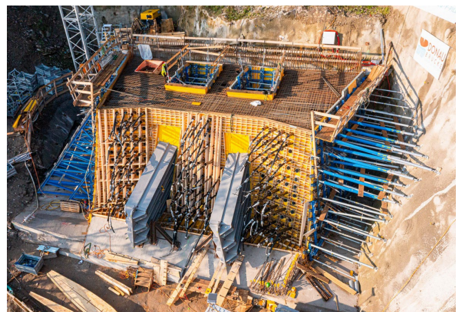
Figure 14: Anchor Block south before concreting / ASFINAG
