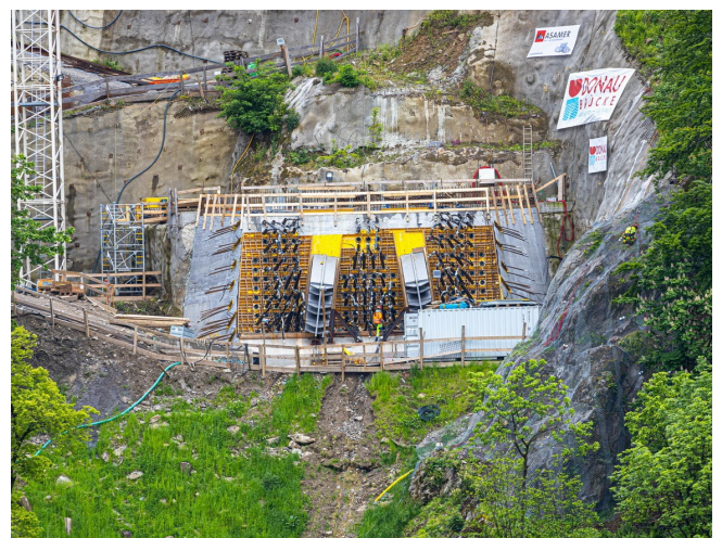
Figure 13: Anchor Block South / ASFINAG
