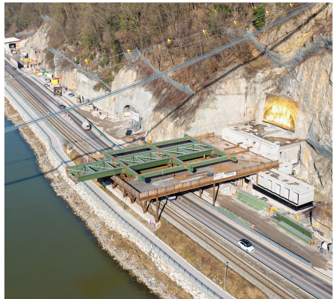
Figures 23 and 24: Pre-assembled deck segments 1 and 9 (South / North) ASFINAG
