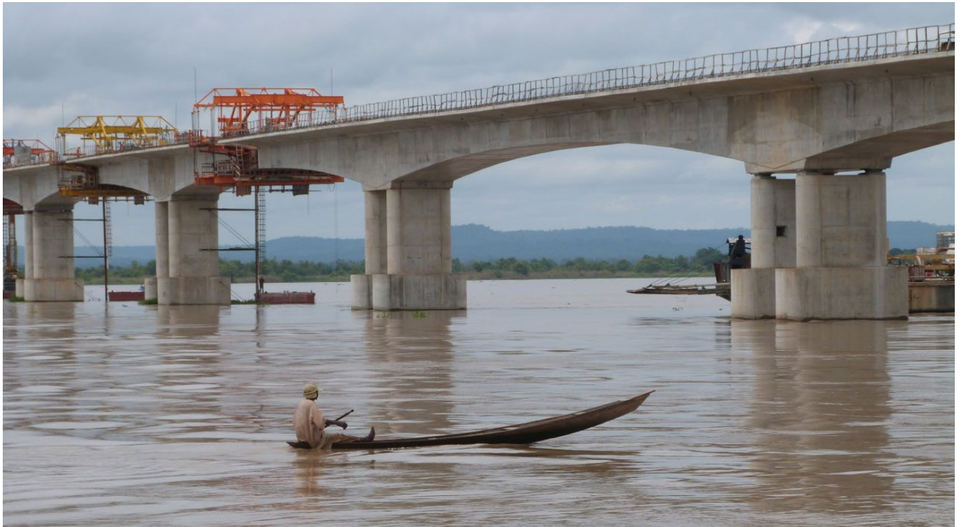
Figure 8: River and Bridge - the typical span length is 85 m
