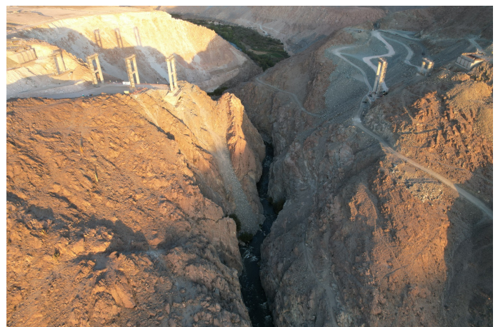
Figure 5: View of the construction site before installation of the bridge
