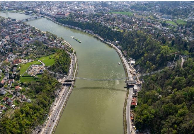
Figure 17: First installed suspension cable schlaich bergemann partner
