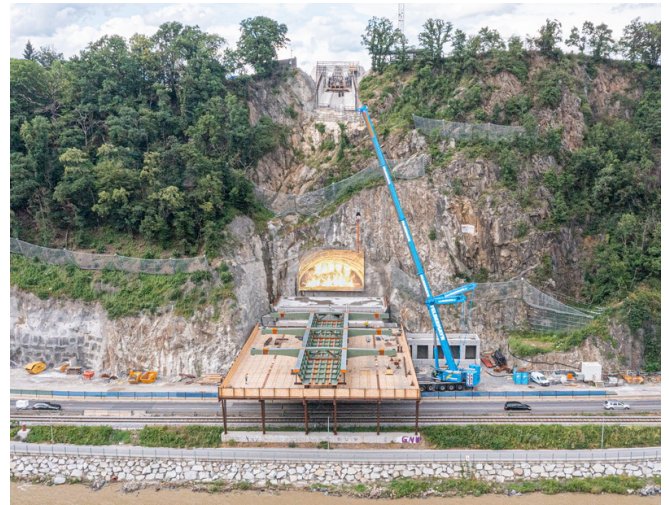
Figure 11: Abutment & tunnel portal south / ASFINAG
