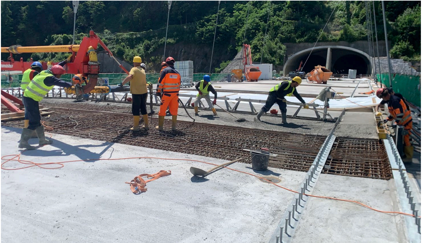
Figure 32: In-situ concreting of deck slab / schlaich bergemann partner
