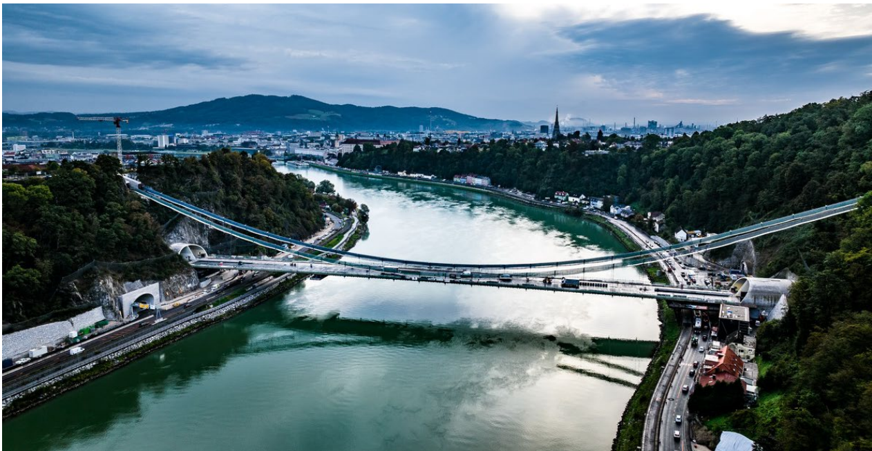
Figure 1: Bridge View / ASFINAG
