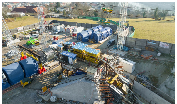
Figure 16: Cable drums / uncoiling wheel, cable tensioning unit/anchor block north ASFINAG
