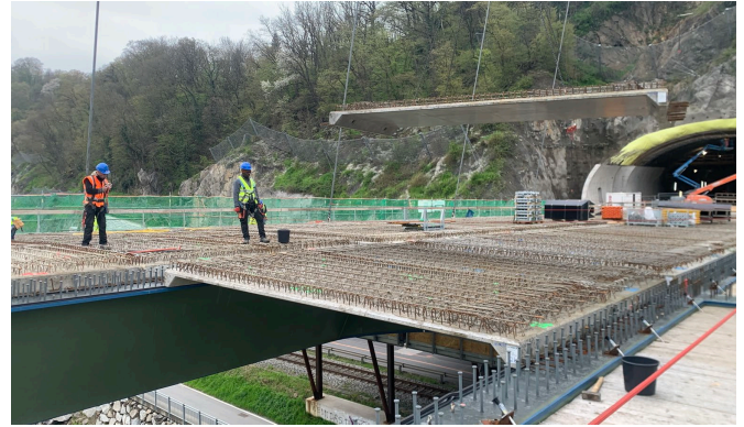
Figure 6: Installation of semi-prefabricated composite slabs schlaich bergemann partner
