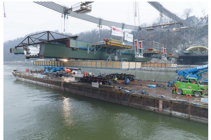
Figure 25: Lifting of the first deck-segement / ASFINAG
