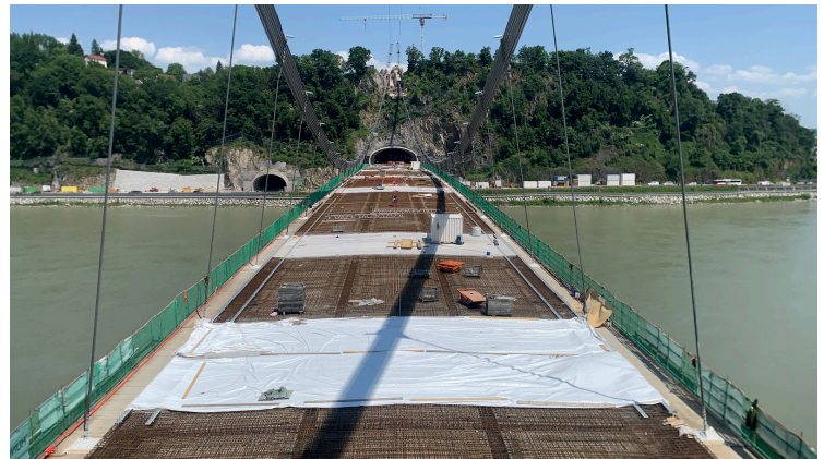
Figure 31: Stage-wise Concreting of the Deck Slab
