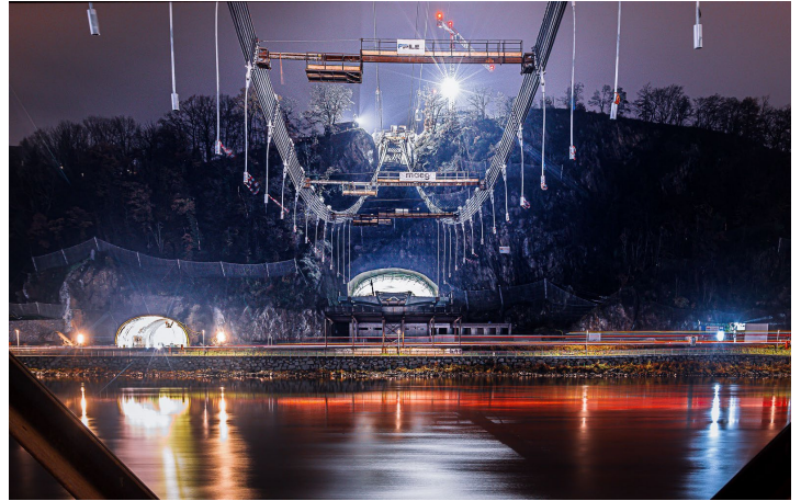
Figure 22: Completion of the cable structure ASFINAG
