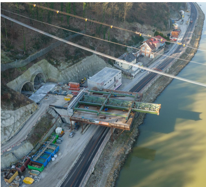
Figures 23 and 24: Pre-assembled deck segments 1 and 9 (South / North) ASFINAG
