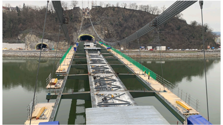
Figure 29: Steel Deck Completion
