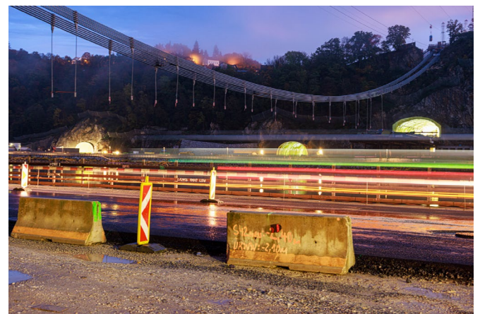
Figure 19: Completion of cable clamp and hanger cable installation ASFINAG
