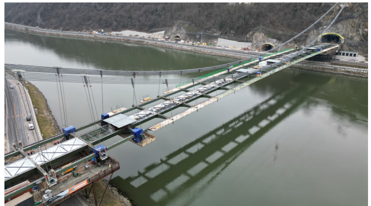
Figure 27: Steel deck installation completed schlaich bergemann partner
