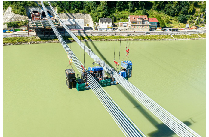
Figure 18: Moveable installation platform for clamp and hanger cable installation / ASFINAG
