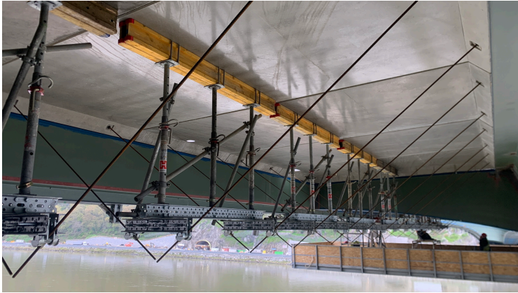
Figure 28: Temporary precast slab supporting schlaich bergemann partner
