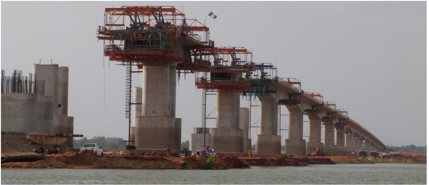
Figure 14: Work during river low level. The column shows the upper water level mark
