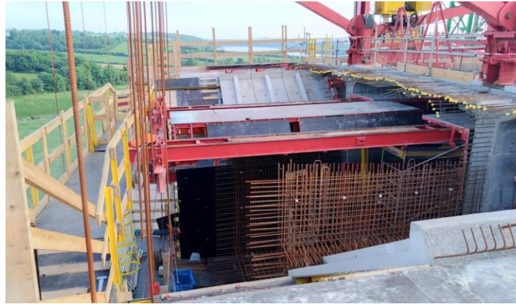
Figure 7: Inner form view from external form
