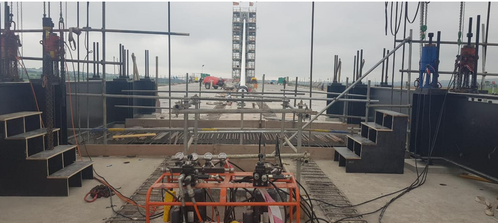
Figure 14: Locking System
