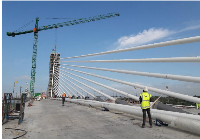
Figure 10: Stay pipe hoisting on P4
