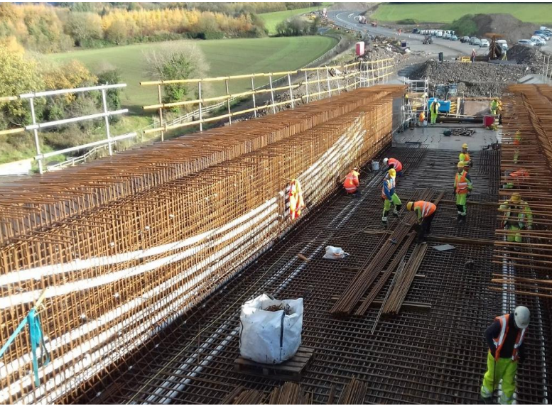
Figure 7: PT works on a typical access span
