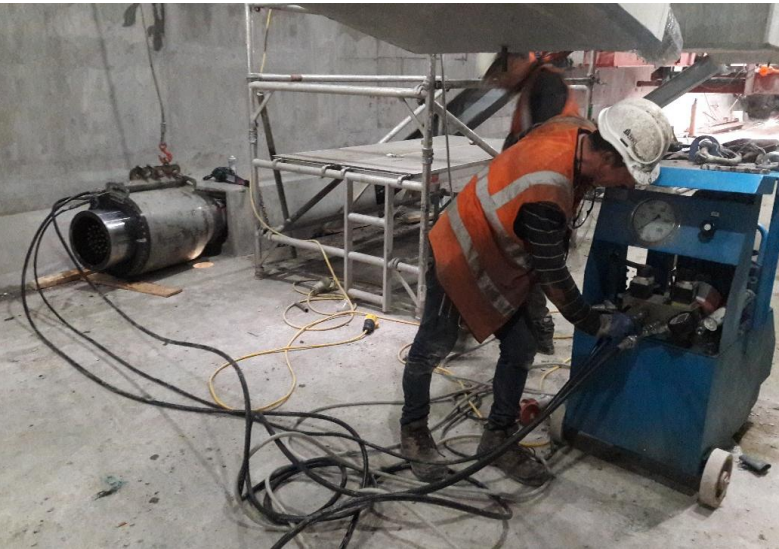
Figure 11: Stressing of a continuity tendon
