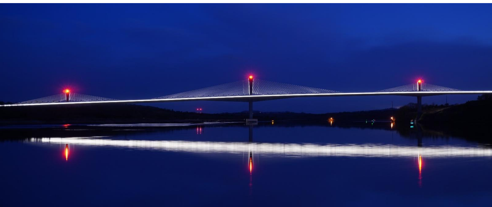
Figure 24: Architectural & Aviation Lighting
