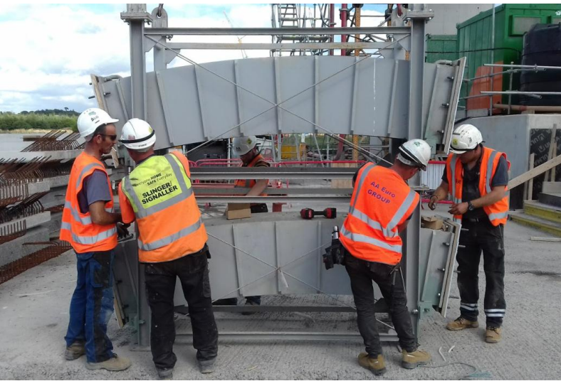
Figures 2 and 3: Multi-tube saddles assembly for lifting and installation
