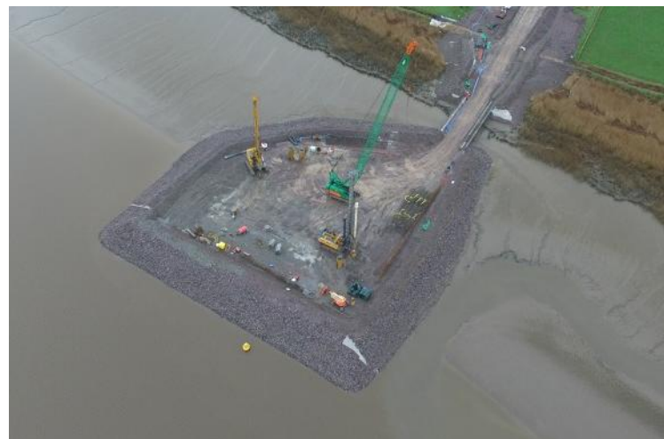
Figure 11: Piling Works on the Platform
