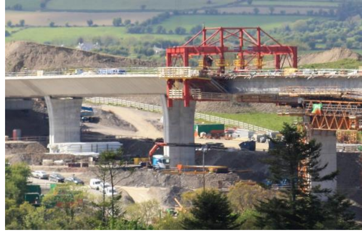
Figure 20: Approach spans construction of precast slabs and cantilevers using a wing traveller
