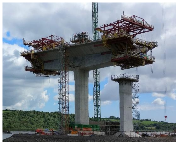
Figure 22: Balance cantilever method deployed at P4 prior to connection to the Push Pull prop
