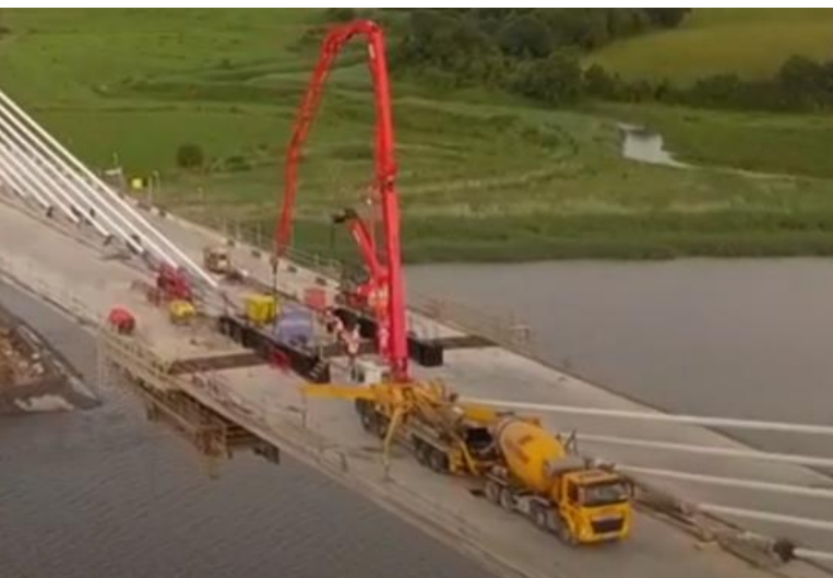
Figure 26: Cantilever blocking beams during the pouring of the closing segment
