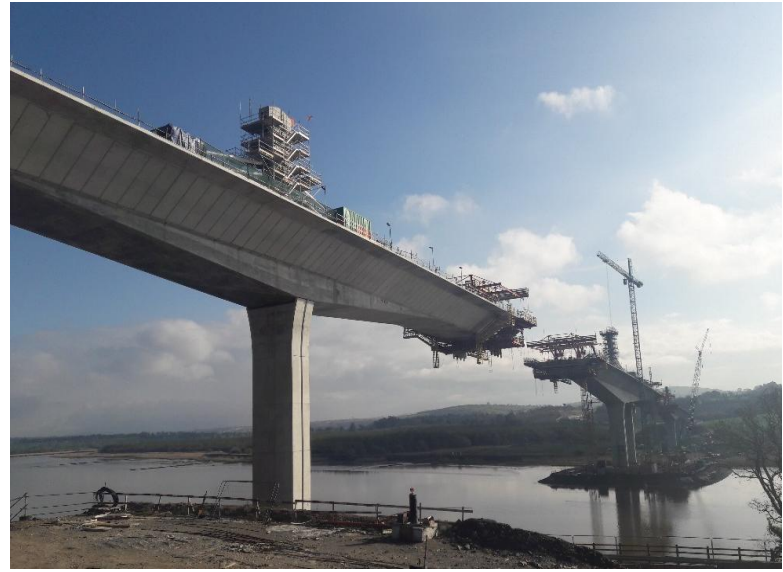
Figure 8: A view of RFK Bridge under construction during cantilever working phases on P3 and P4
