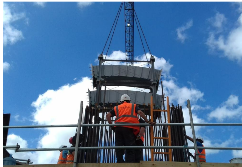
Figures 2 and 3: Multi-tube saddles assembly for lifting and installation
