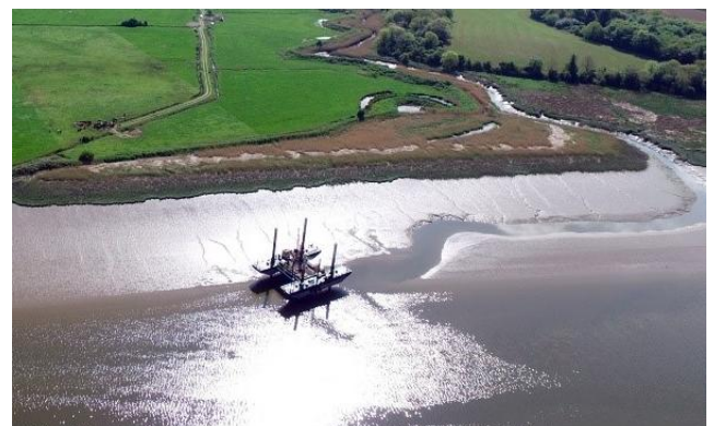
Figure 9: Jack-up Barge for GI Works
