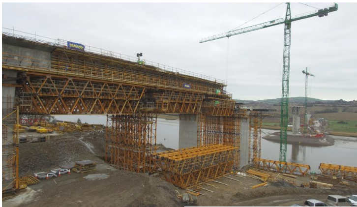
Figure 5: Falsework in Span 2
