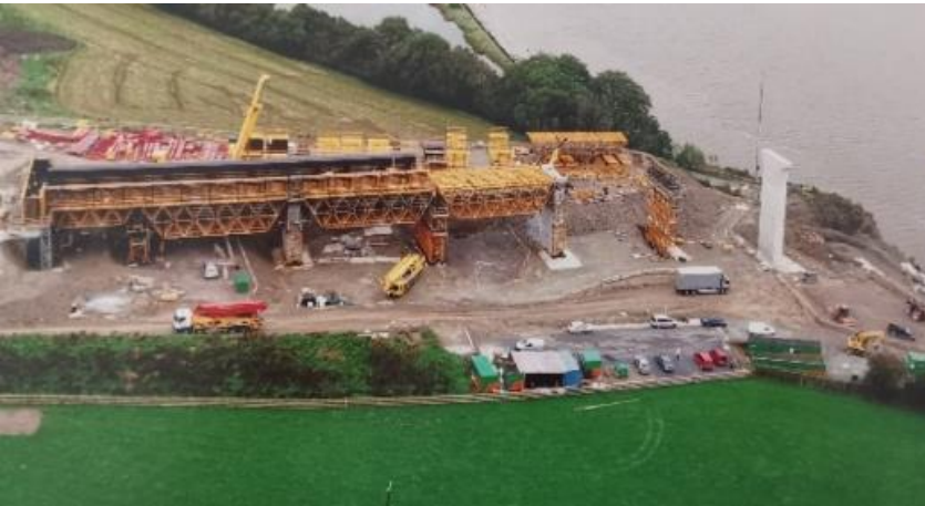
Figure 19: Construction of central box at Spans 1 and 2 in the west area of bridge using scaffold to the ground
