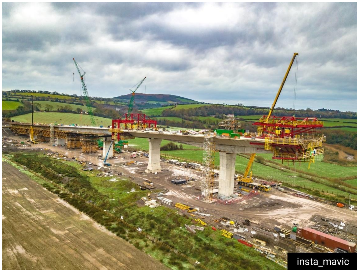
Figure 2: Traveller in P5 side during construction
