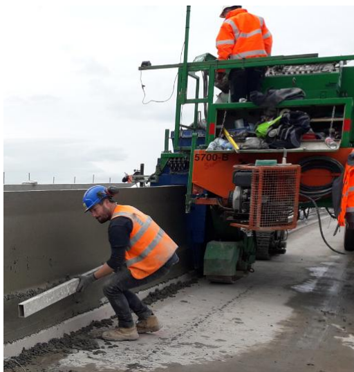
Figure 21: Barrier Slip-forming Operation
