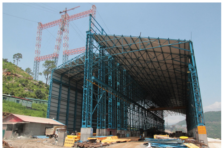
Figure 4: Steel frame construction for the arch workshop
