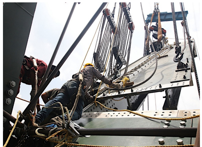
Figure 27: Installation of top chord
