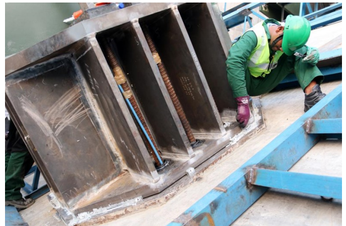
Figure 23: Installed injection holes for filling the gap
