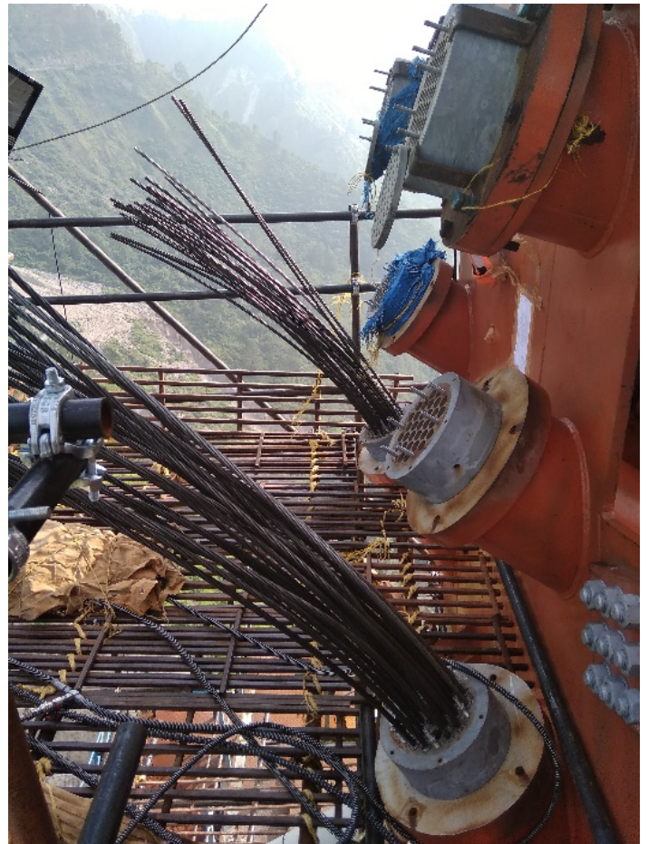
Figure 3: Stressing anchors at the temporary towers
