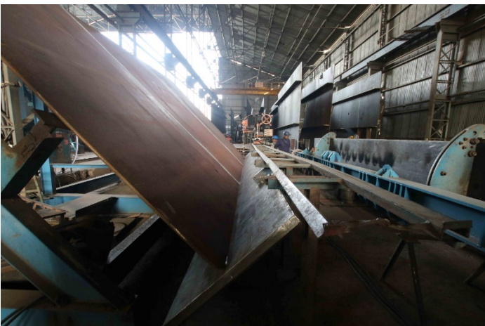
Figure 28: Welding bottom flange – web plate after rotation
