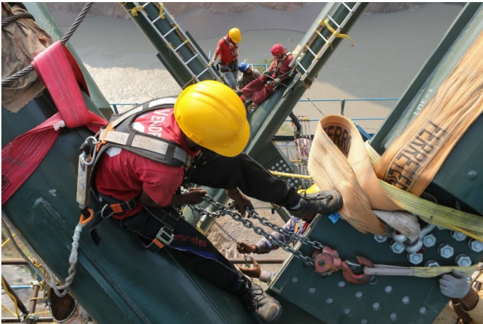
Figure 32: Matching the drilling holes for the bolting joints in height
