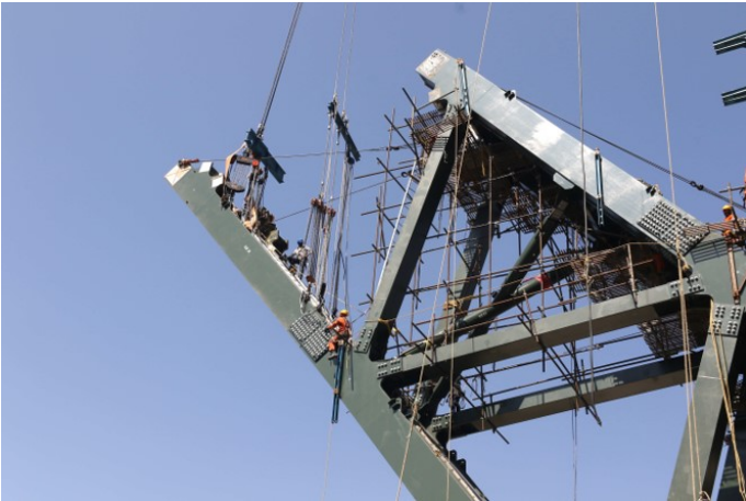
Figure 24: Installation of the bottom chord
