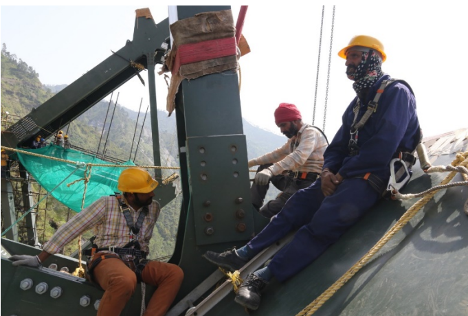
Figure 26: Installation of the diagonal
