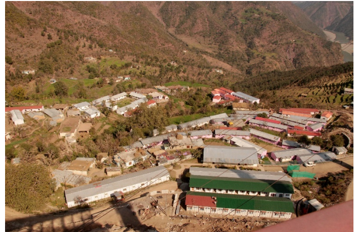
Figure 2: Camp on site for engineers and workers
