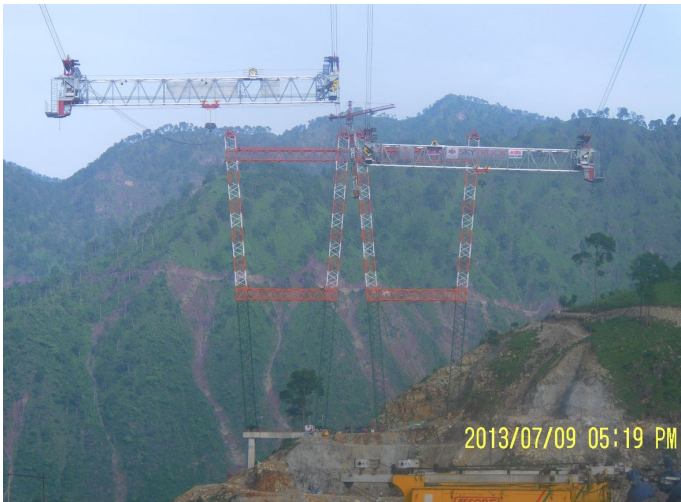
Figure 4: Skytruck 200 in operation
