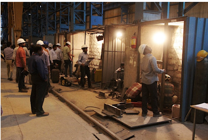
Figure 18: Welder qualification according to DIN EN 281-1
