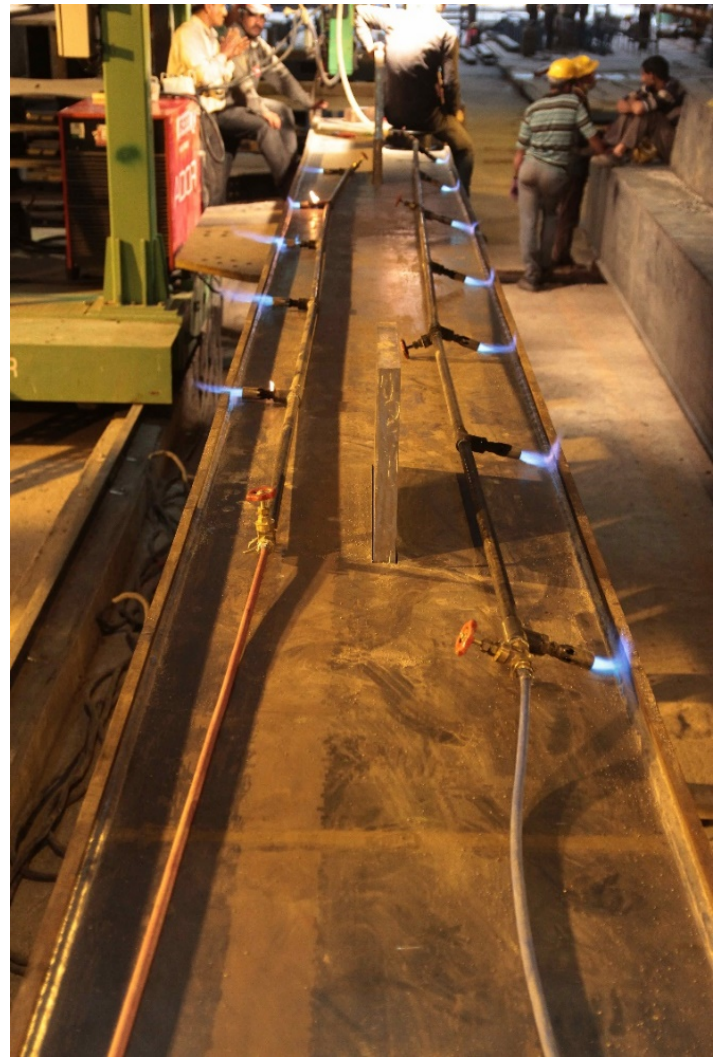
Figure 35: Heating during welding with gas
