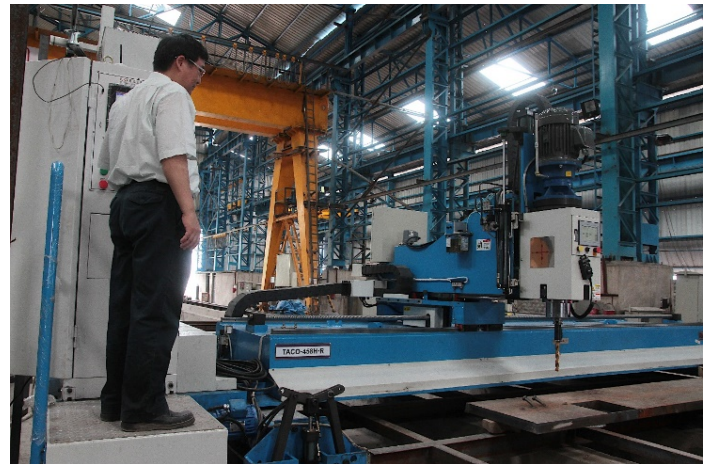
Figure 16: Installed drilling machine in arch workshop
