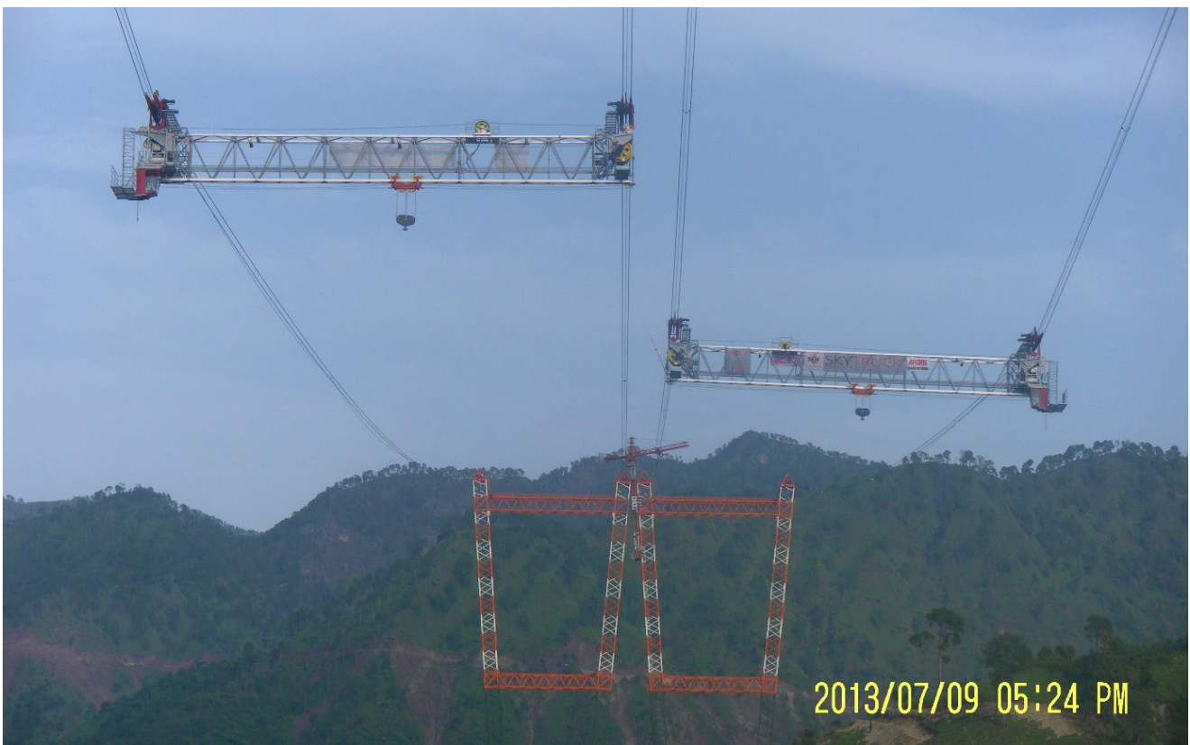
Figure 1: Skytruck working at Chenab Bridge construction
