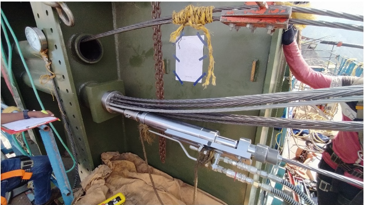
Figure 9: Stressing of horizontal ties
