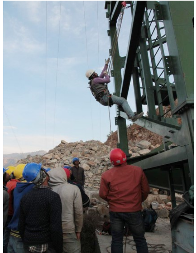
Figure 12: Training in climbing on site
