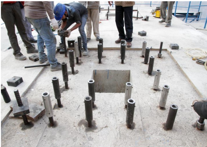
Figure 4: Plates for correct installation of the base segment
