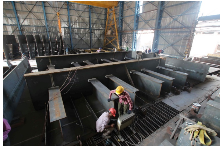
Figure 24: Tacking of cross girder and LT beams
