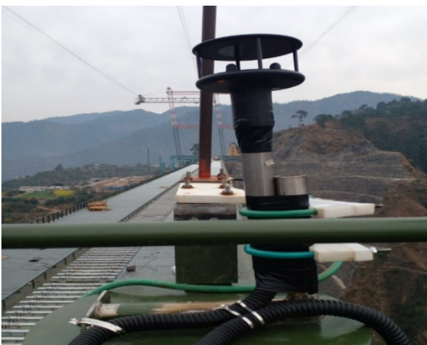
Figure 5: Anemometer installed on the mast
