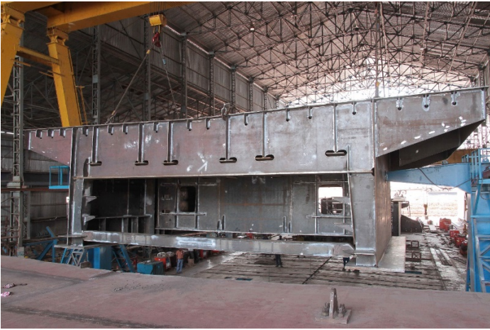
Figure 32: Final position for finishing welds on deck plate
