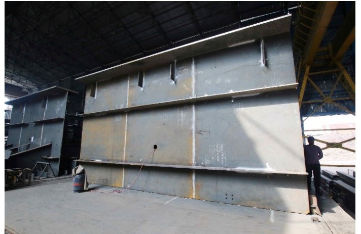
Figure 29: Tacking web on deckplate
