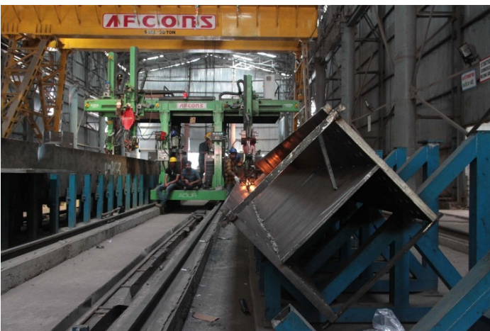
Figure 34: Welding of part 1 for the hollow section with welding gantry
