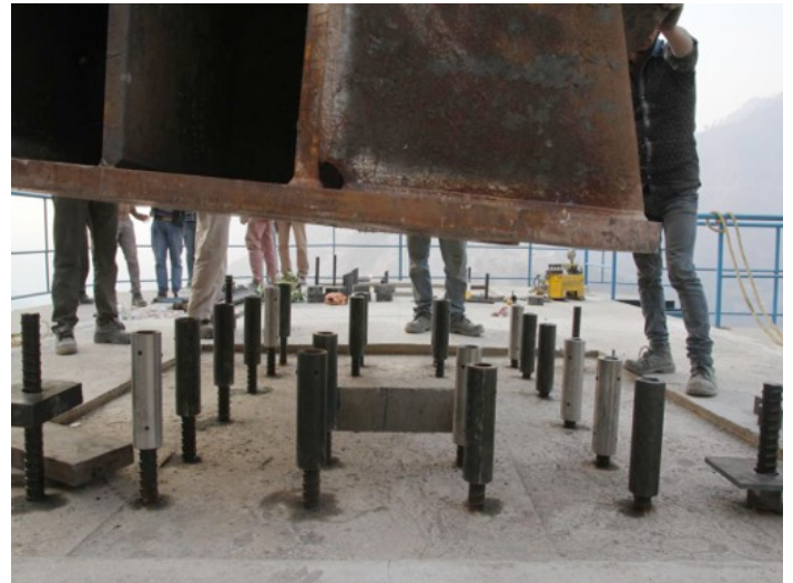
Figure 6: Leading the base segment to match the drilling holes
