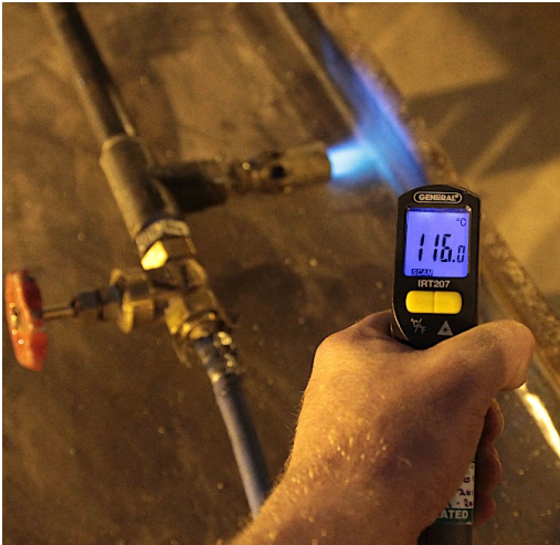
Figure 37: Checking heating temperature during welding
