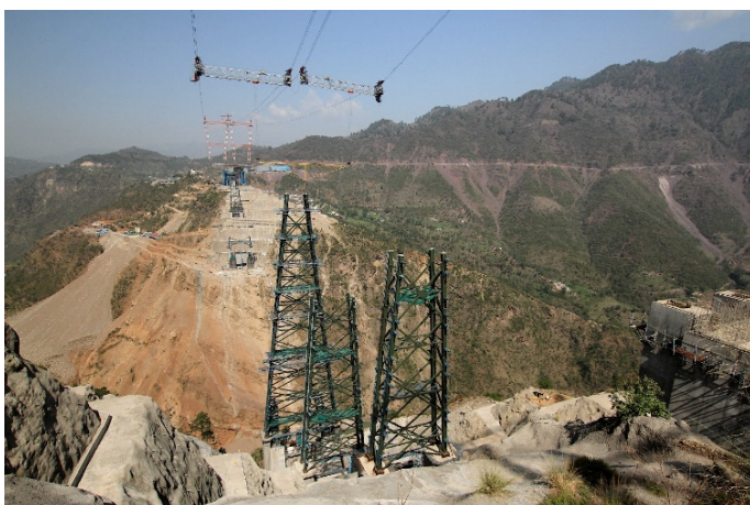
Figure 17: Pier assembly in progress
