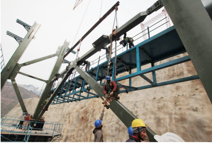
Figure 14: Vertical cross-bracing installation
