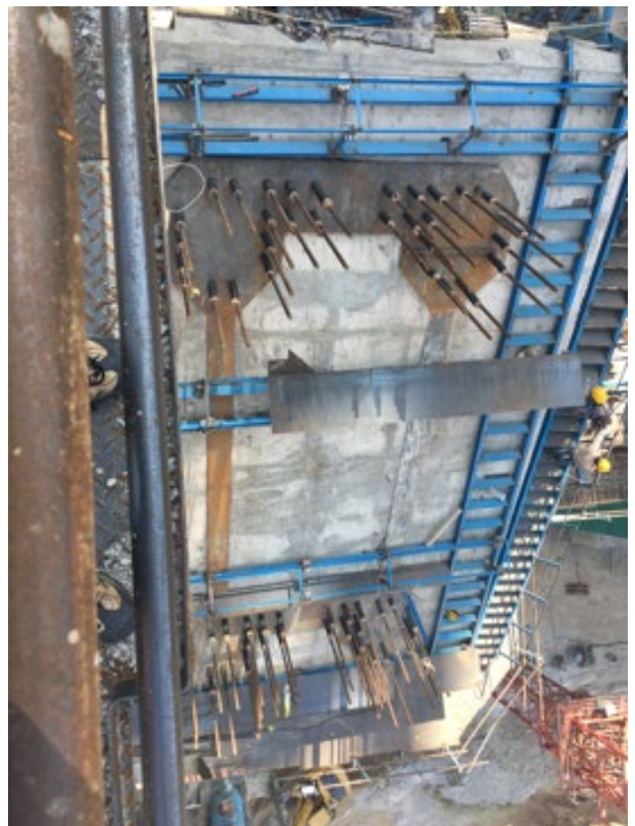
Figure 2: Arch base plate with Dywidag bars
