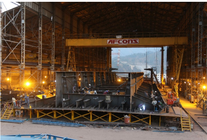
Figure 33: View in the workshop with at least five fabrication trolleys in parallel
