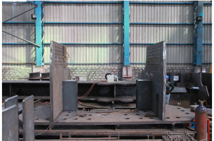
Figure 38: Tacking of web plates for the arch base segment
