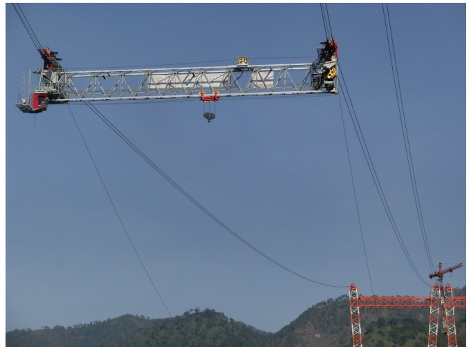
Figure 2: Skytruck 200 in operation
