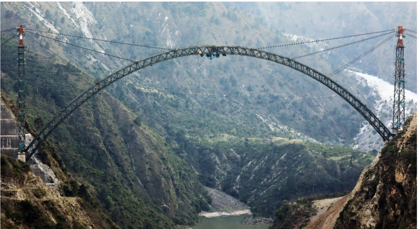
Figure 5: Arch after closure
