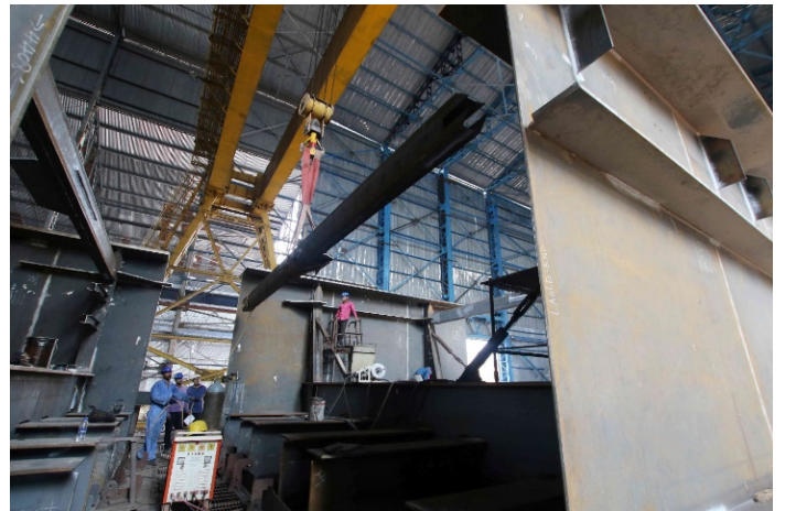
Figure 30: Installation of bracing in the bottom flange level
