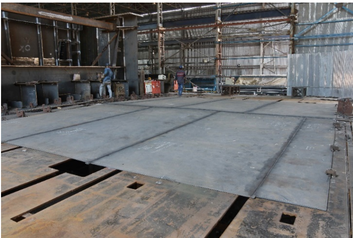
Figure 22: Welding deck plate
