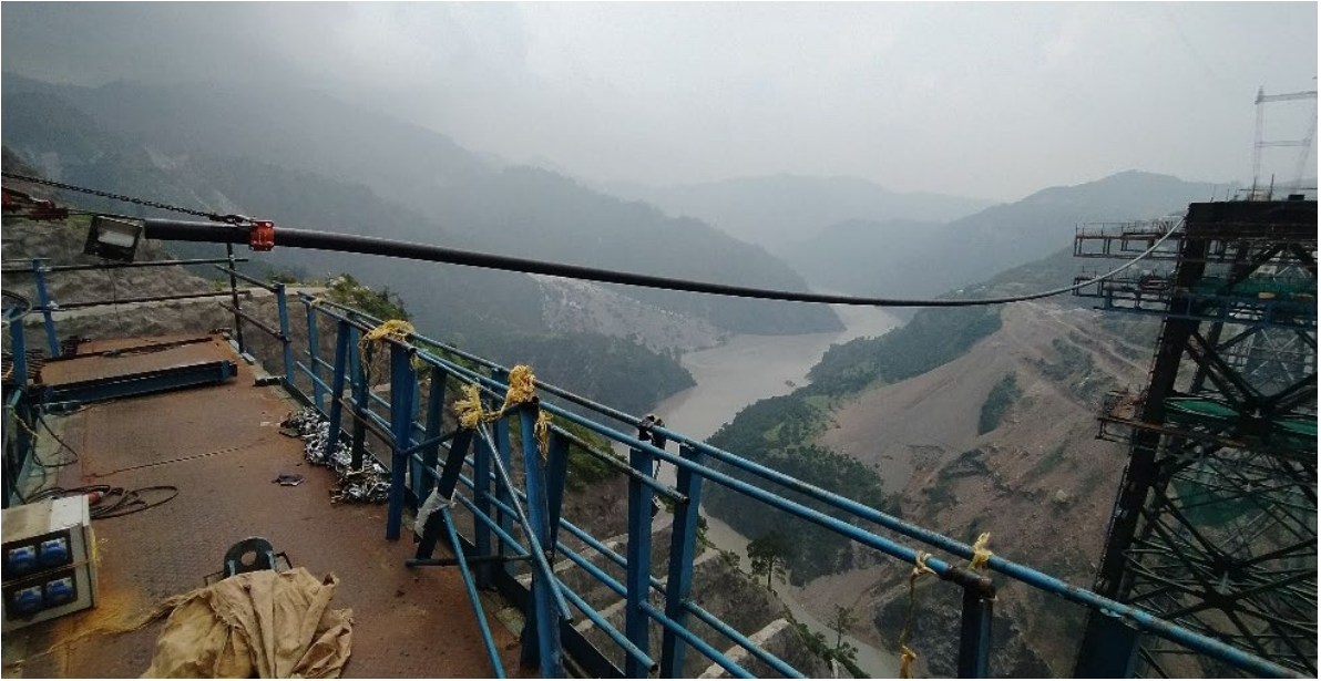
Figure 8: Horizontal ties during installation
