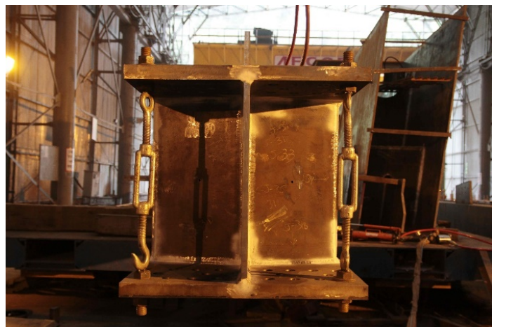
Figure 36: Temporary fittings for reducing distortion from welding
