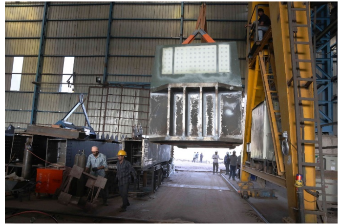
Figure 43: Lifting of the base segment
