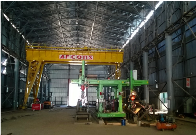
Figure 15: Welding gantry in a workshop for piers
