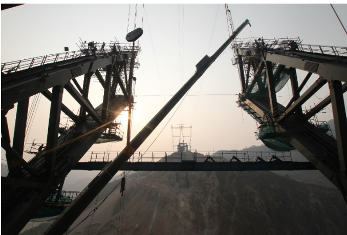
Figure 30: Installation of the first 60m diagonal
