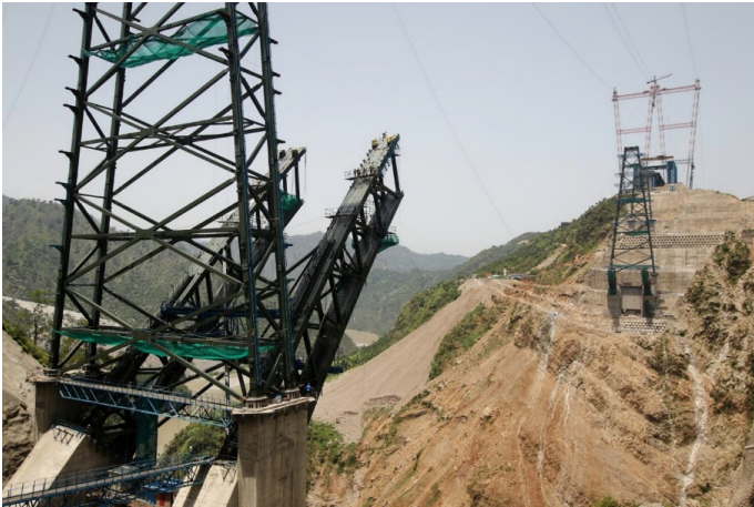
Figure 28: Step by step the triangles of the arch were installed
