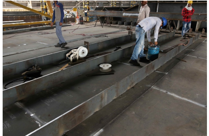
Figure 23: Welding ribs on deck plate
