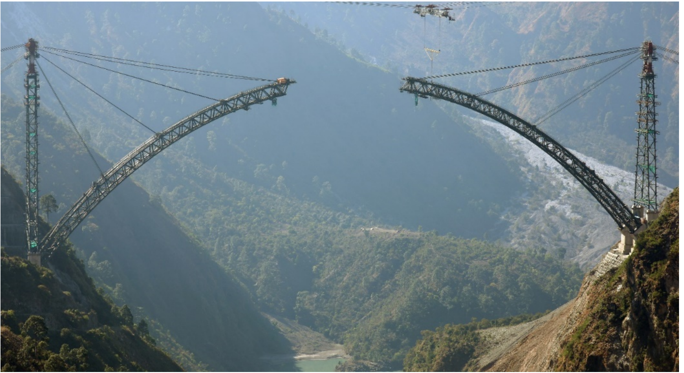
Figure 4: Arch before closure; shortest forestays already dismantled
