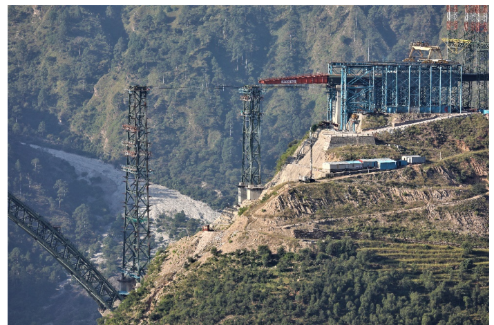
Figure 7: Horizontal ties partly in place
