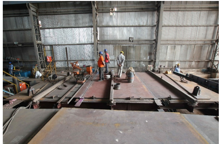
Figure 25: Welding of web plate
