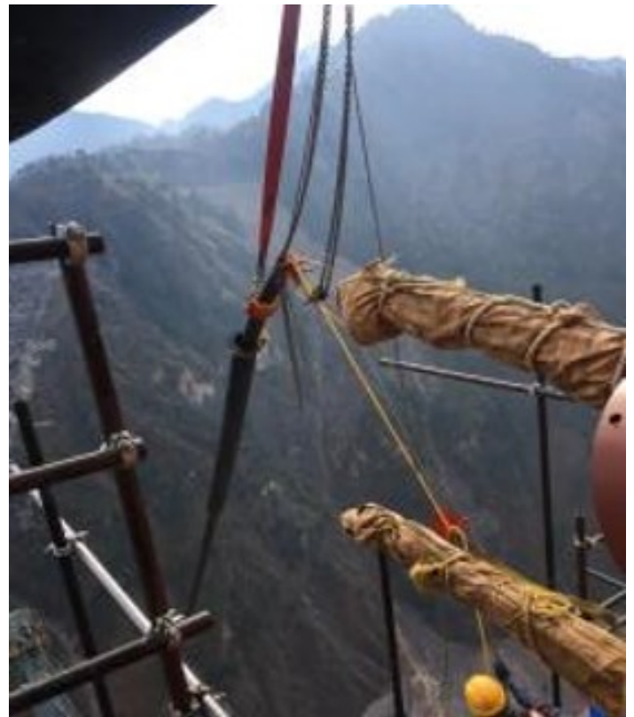
Figure 6: Stay pipe removal
