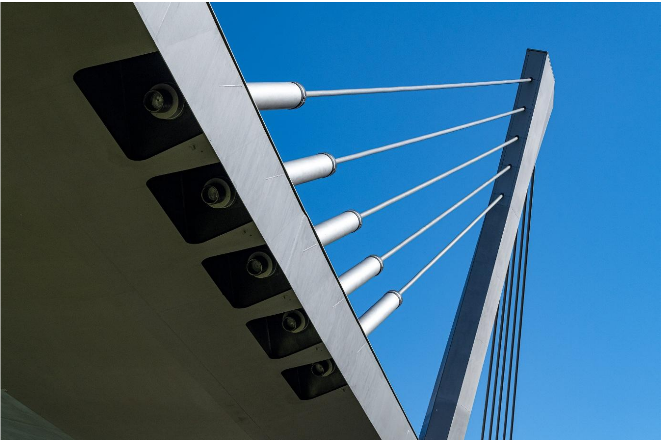
Figure 11: Pylon and Cables
