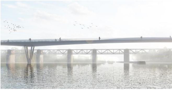
Figure 8: View of the bridge with existing weir and weir bridge in the background
