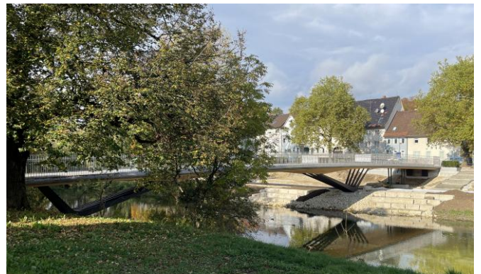
Figure 6: Hybrid structure of Rathausbrücke Tuttlingen Credit: sbp
