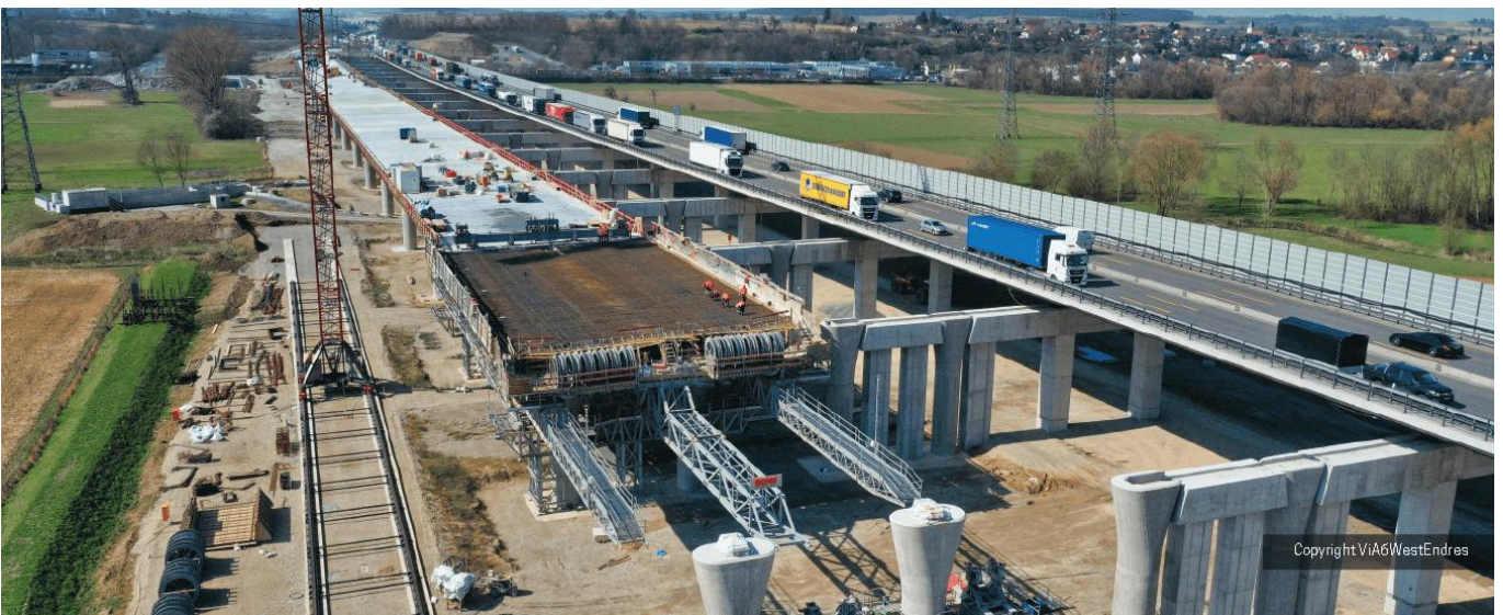
Figure 3: The deck construction
