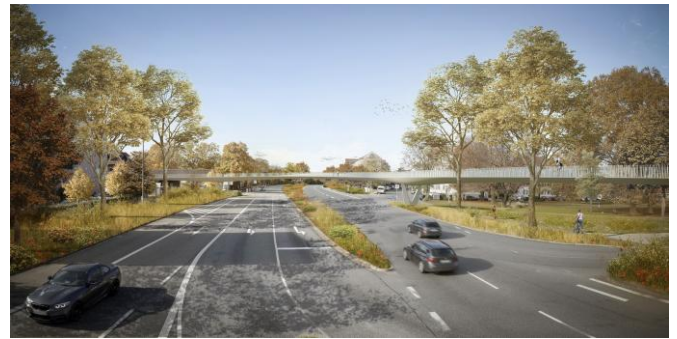
Figure 11: Support-free overpass over the B37 and continuing into Gneisenau Park (right)
