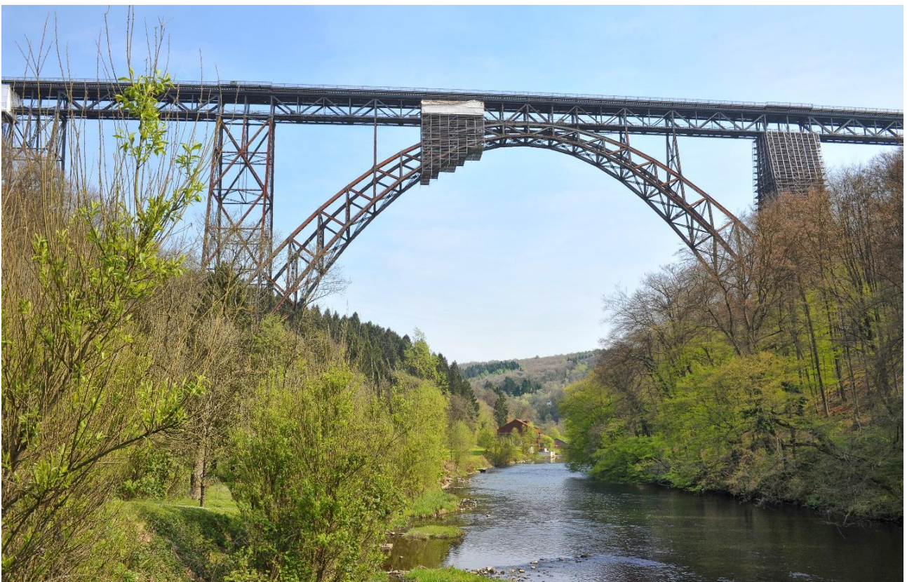
Figure 1: The Müngsten Bridge is the highest steel railway bridge in Germany with a height of 107 m
