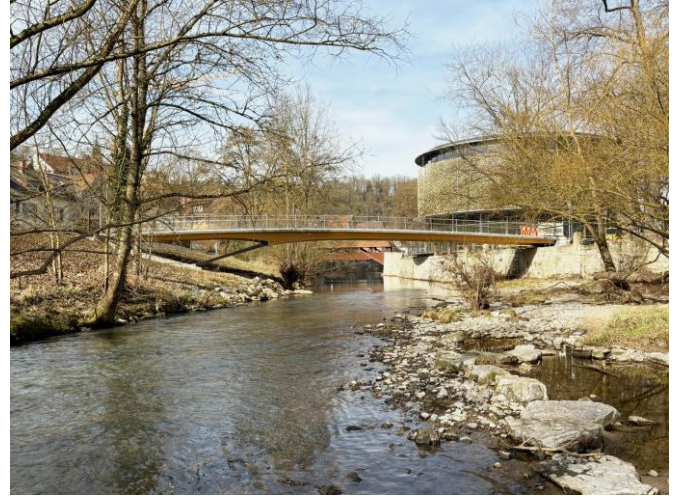
Figures 20 and 21: Inclined central support designed as trapezoidal hollow steel box (left) / bridge view with theatre in the background (right)
