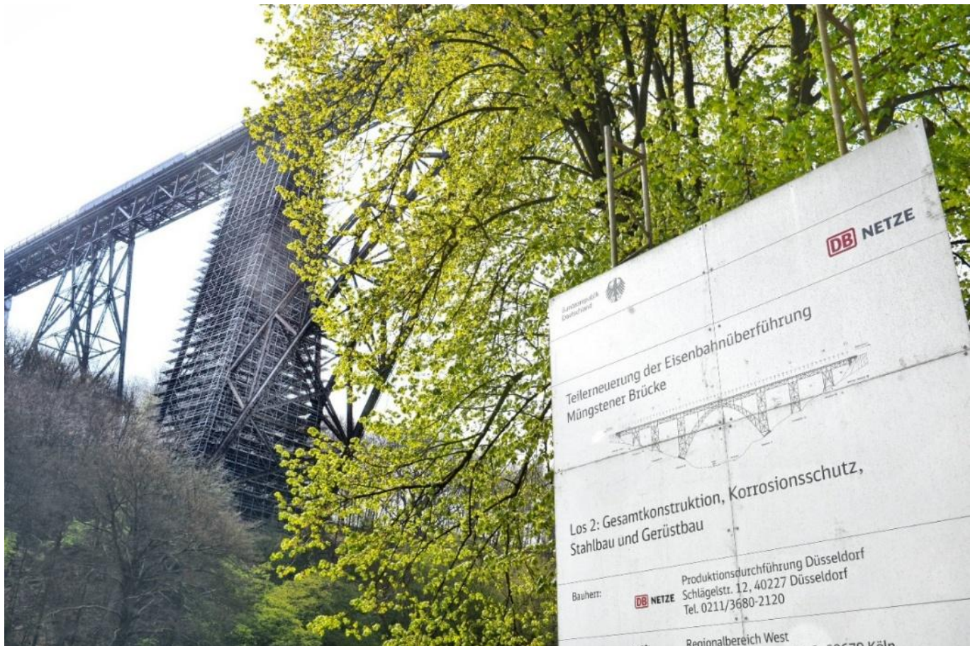
Figure 3: The refurbishment work began in 2013
