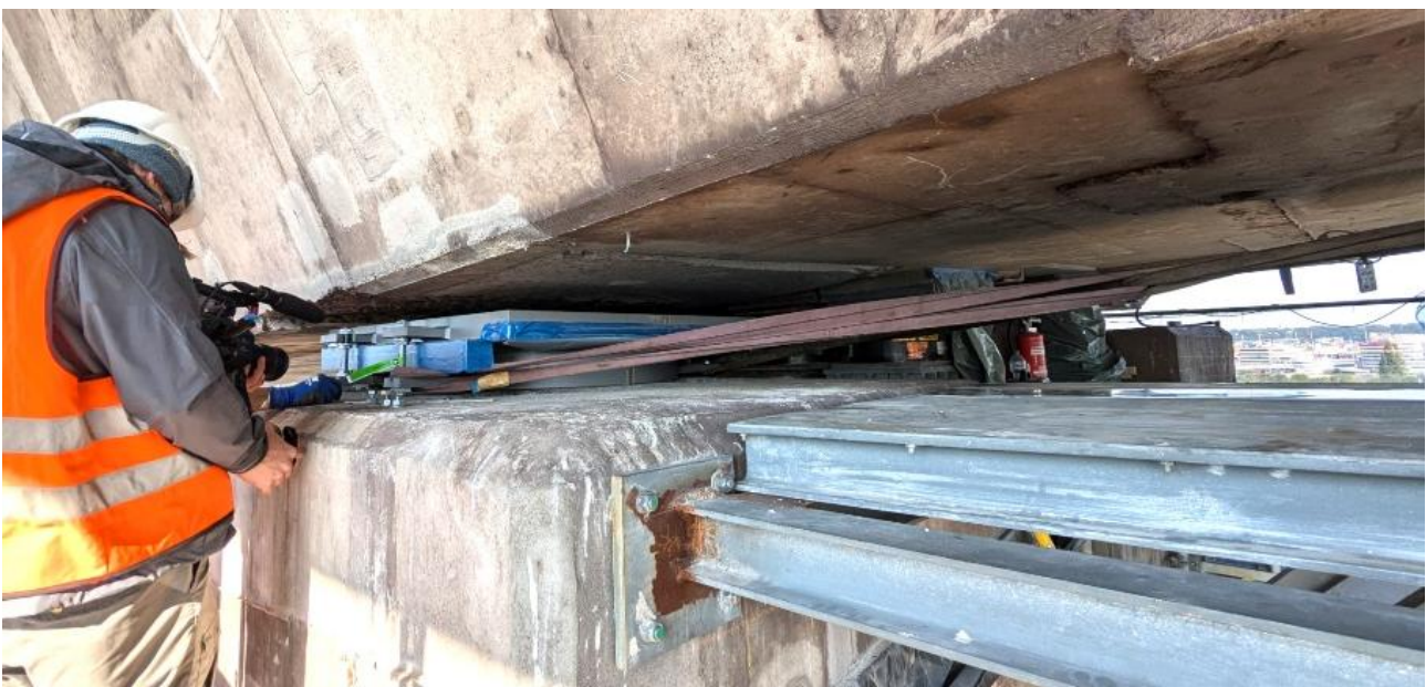
Figure 3: Taking away the old bearing
