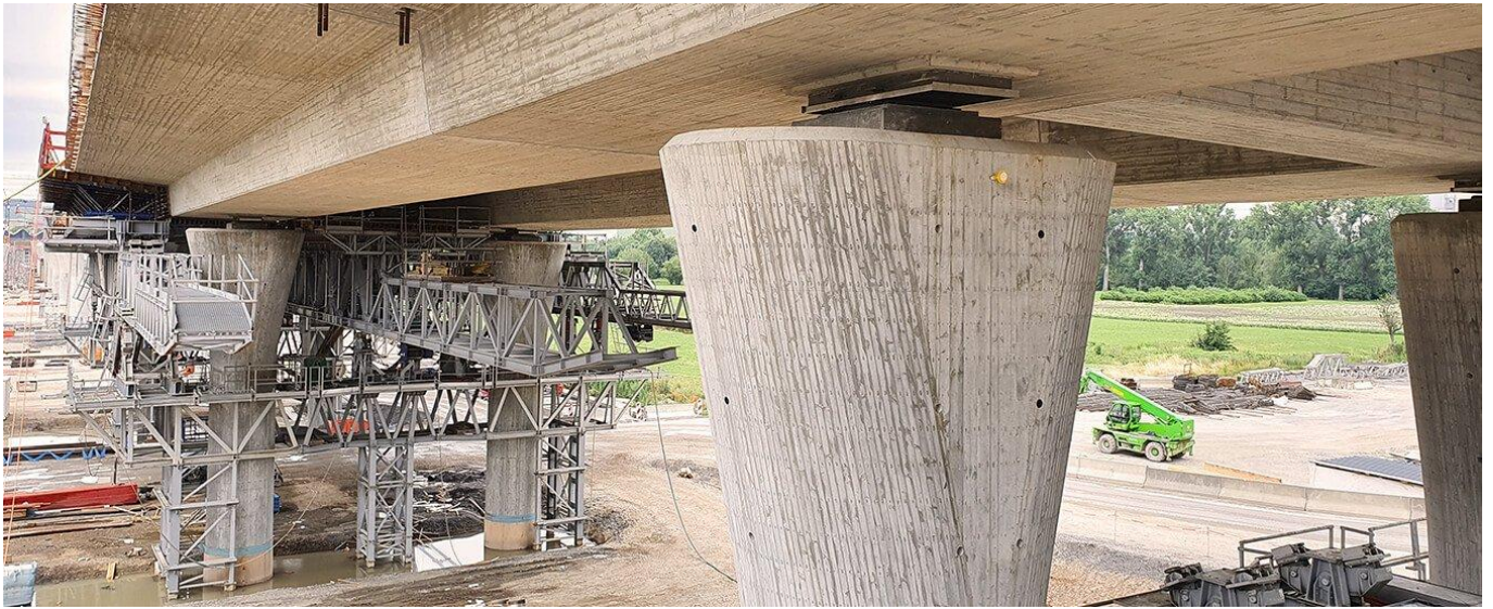
Figure 6: The MSS operating under the deck
