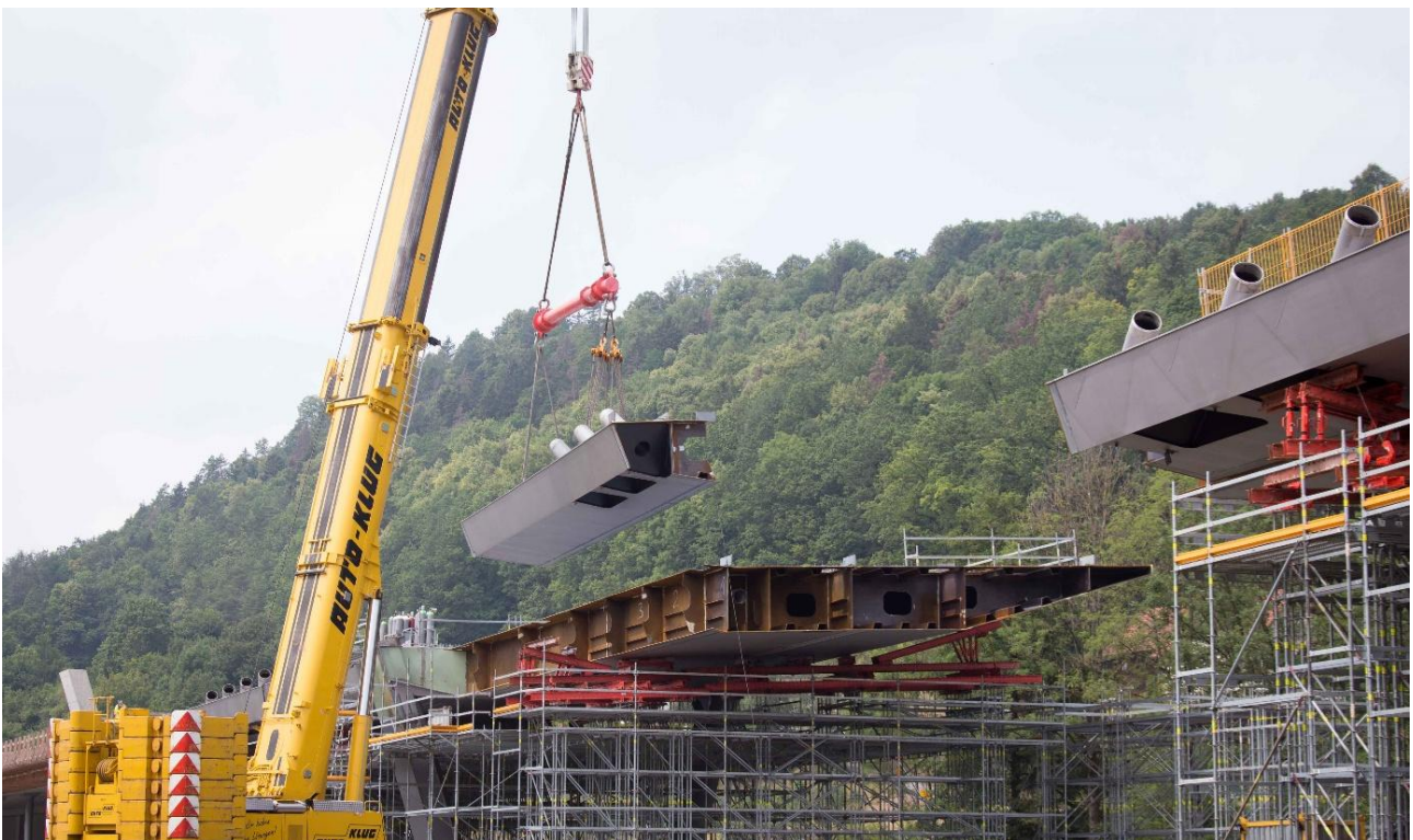
Figure 7: Steel Works Erection
