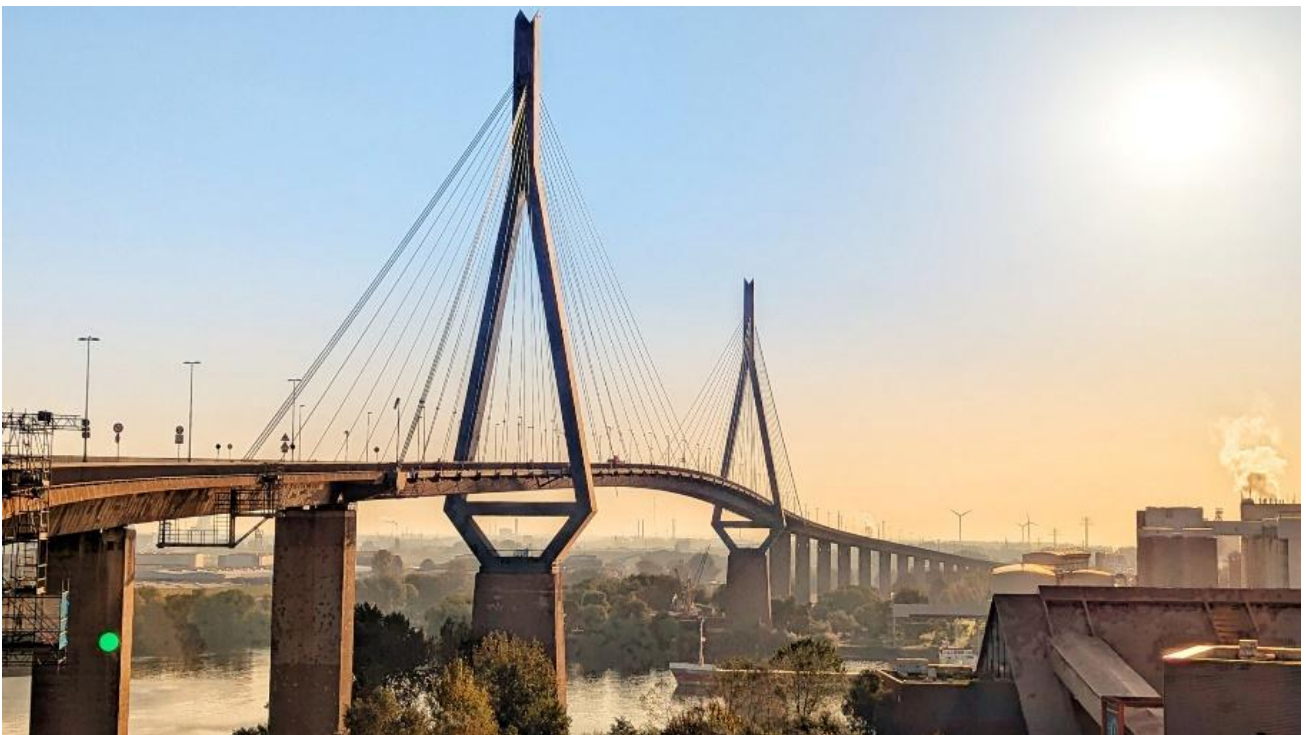
Figure 1: The Köhlbrand Bridge in Hamburg
