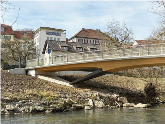
Figures 20 and 21: Inclined central support designed as trapezoidal hollow steel box (left) / bridge view with theatre in the background (right)
