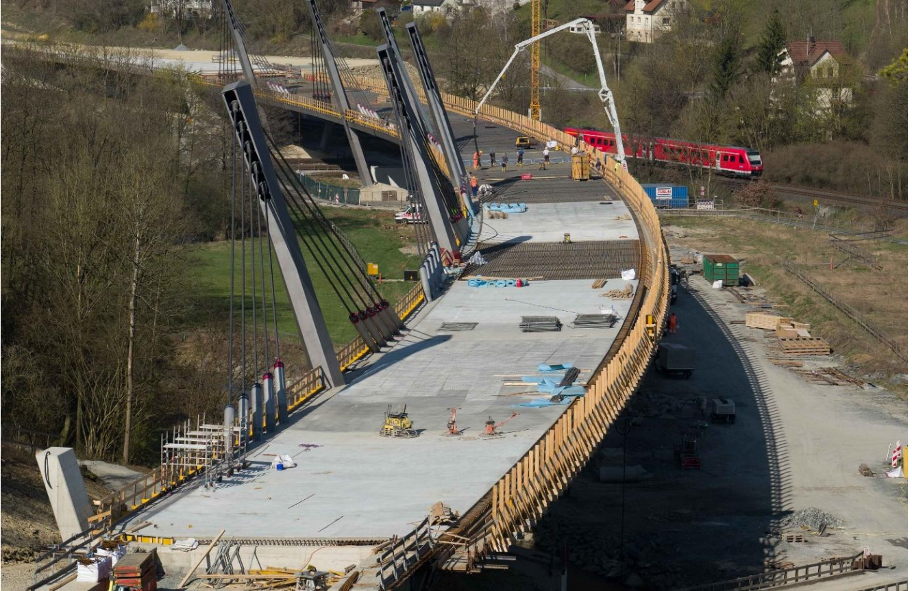
Figure 8: Concreting Deck
