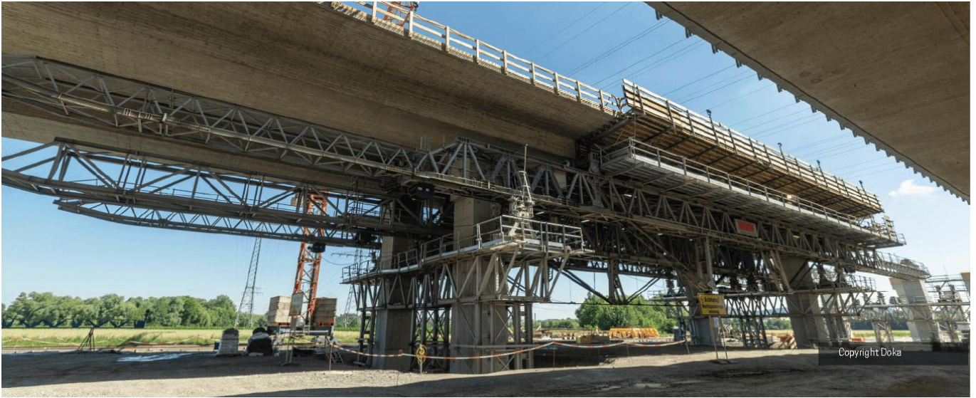
Figure 2: Underslung movable scaffolding system M38-I
