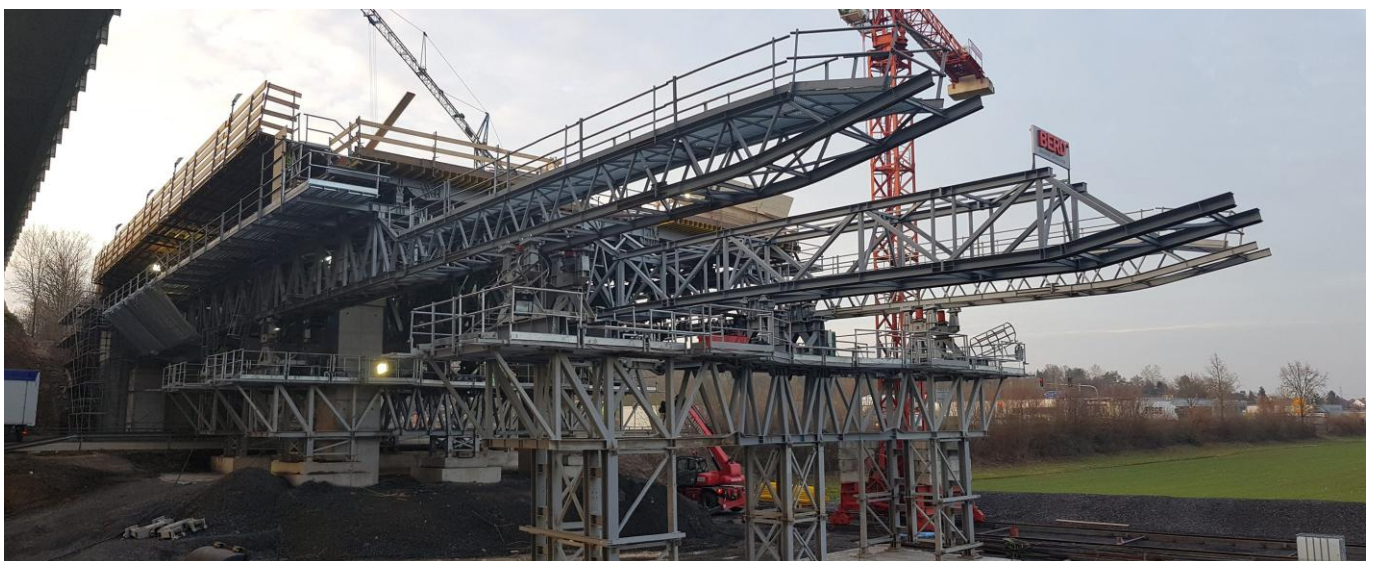
Figure 8: The MSS ensured fast construction within cycles of nine days
