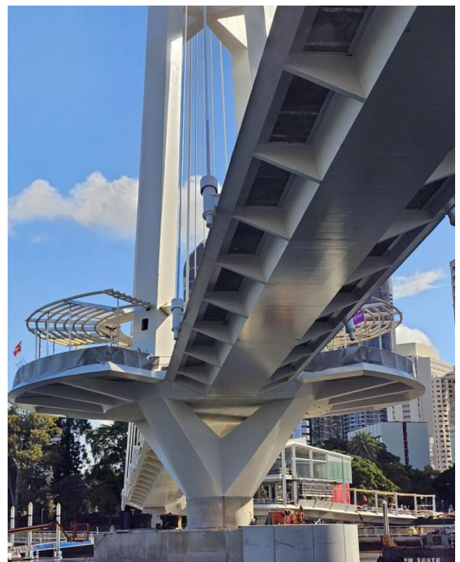
Figure 2: View of the deck and the Bridge from water
