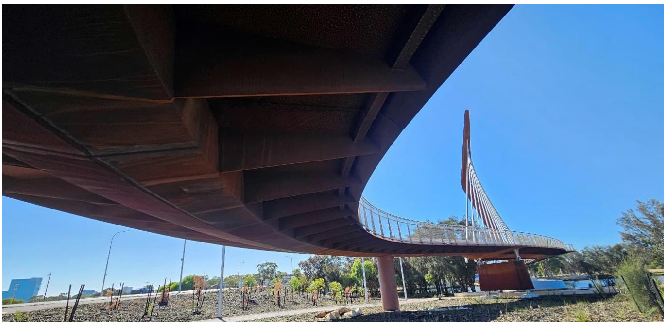
Figure 14: The approach spans and the deck transition at Pier 3
