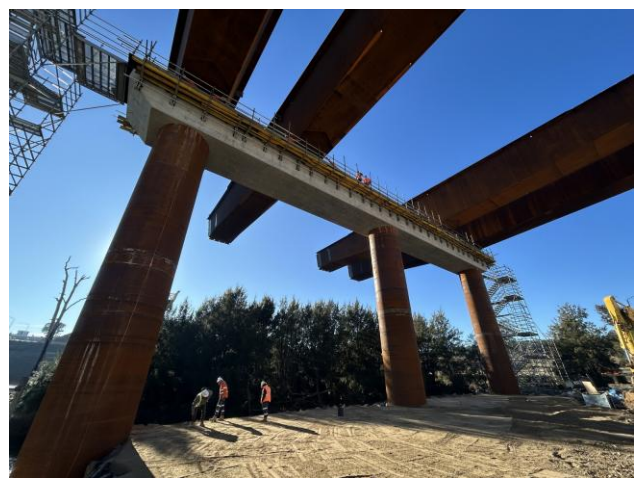
Figure 5: View from below
