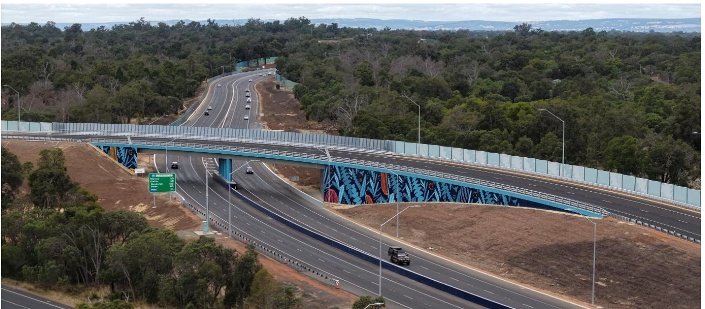
Figure 8: Wilman Wadandi Highway southern entry – Bridge 1907
