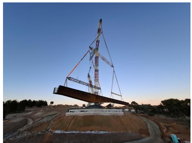
Figure 3: Heavy lifting operation
