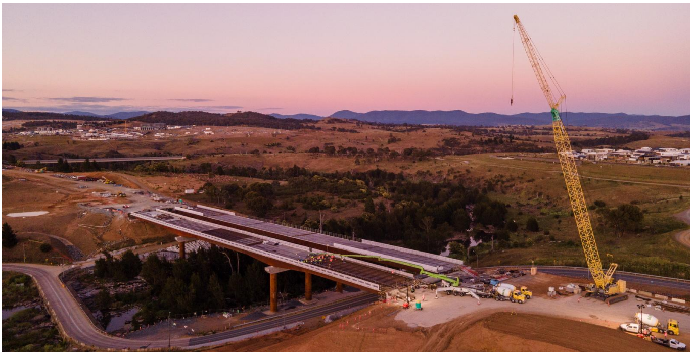
Figure 1: Construction of the Molonglo River Bridge
