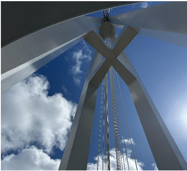
Figure 10: The steel box legs of the mast are kept slender with the help of a cruciform bracing part way up
