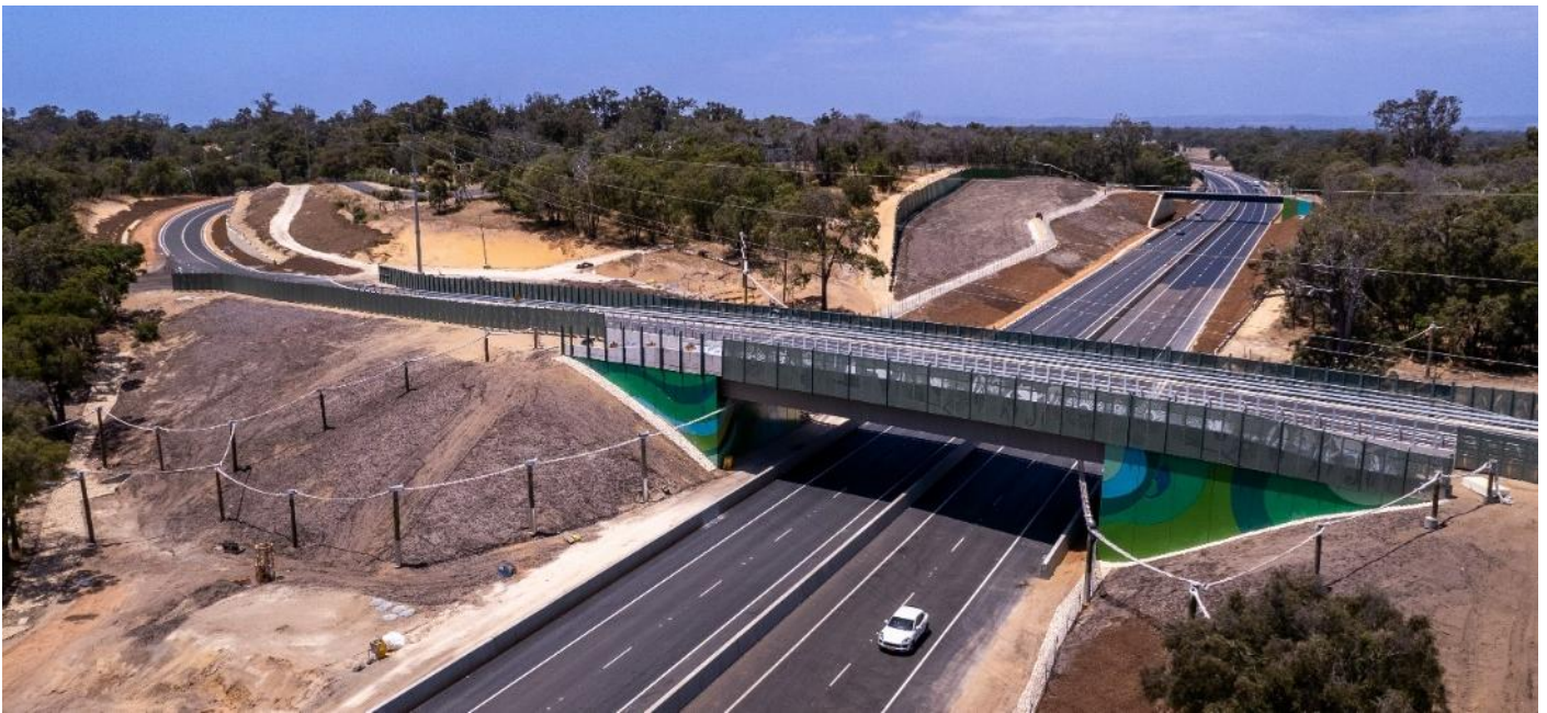
Figure 1: Yalinda Drive Bridge and connections to Fauna rope Structures
