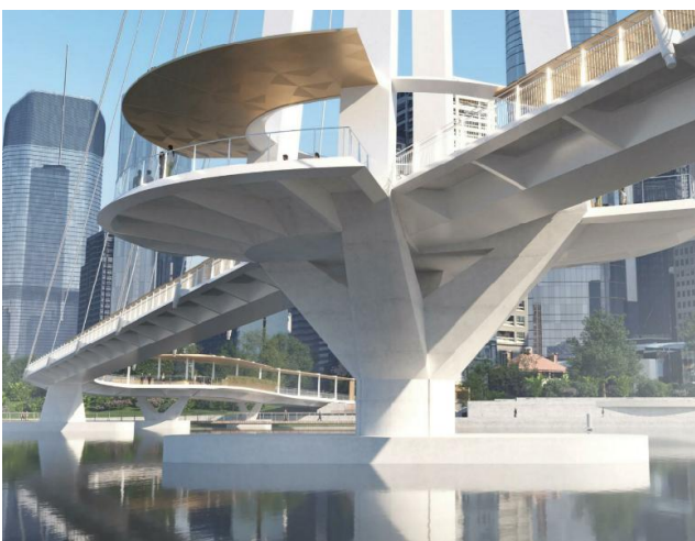
Figure 8: River Pier (Pier 4) arrangement; Architect's Rendering (left), Structural Digital Model (right)
