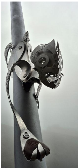
Figure 16: Toanga (treasure) sculpture attached to mast to welcome visitors onto bridge (left); FEA model to confirm the sculpture performance in high winds (right)
