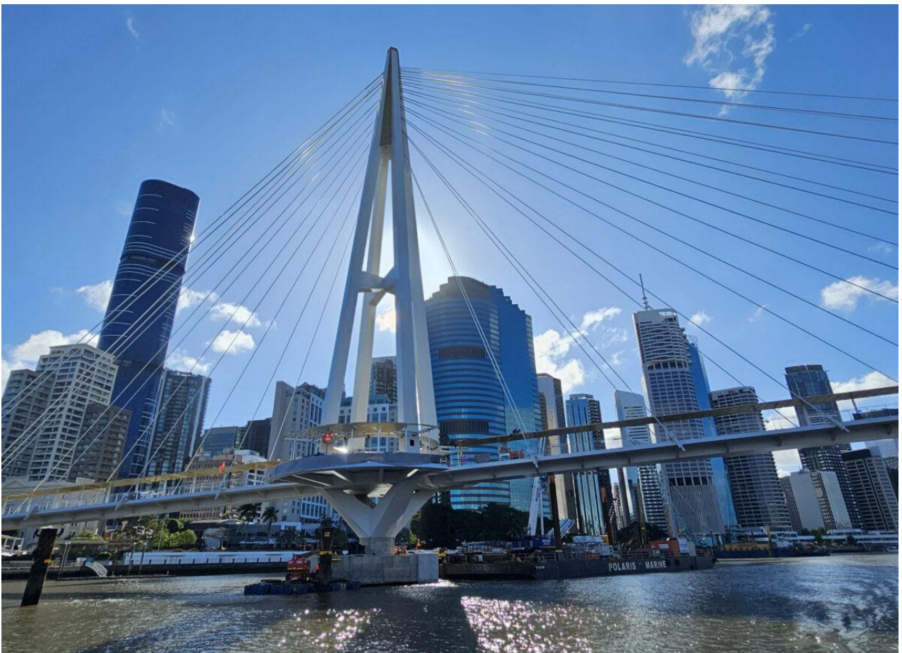
Figure 3: View of the complete Kangaroo Point Bridge
