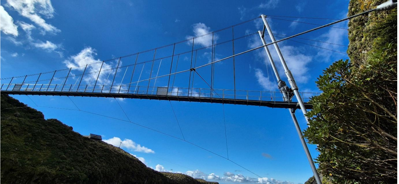
Figure 10: South mast following erection
