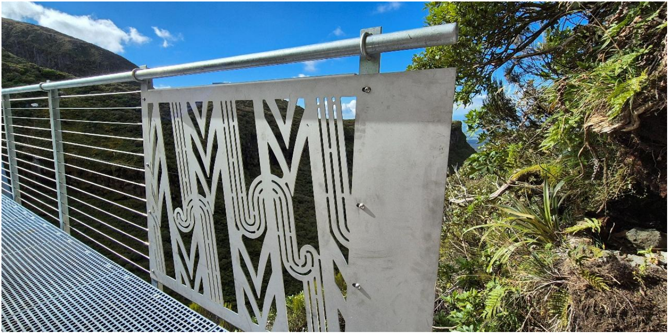
Figure 15: Architectural laser-cut balustrade infill panels
