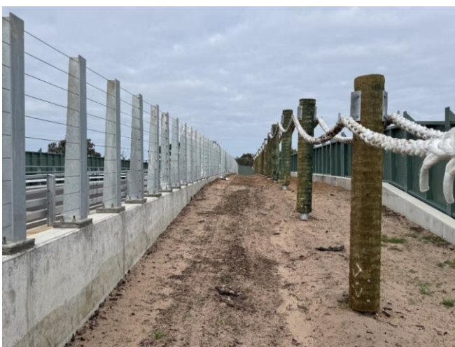
Figure 4: Possum rope crossing design
