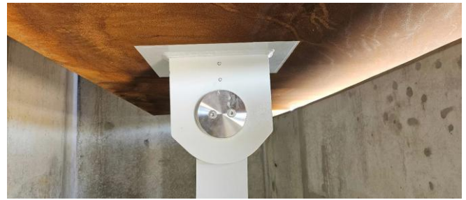
Figure 13: Pendulum anchor to steel diaphragm connection
