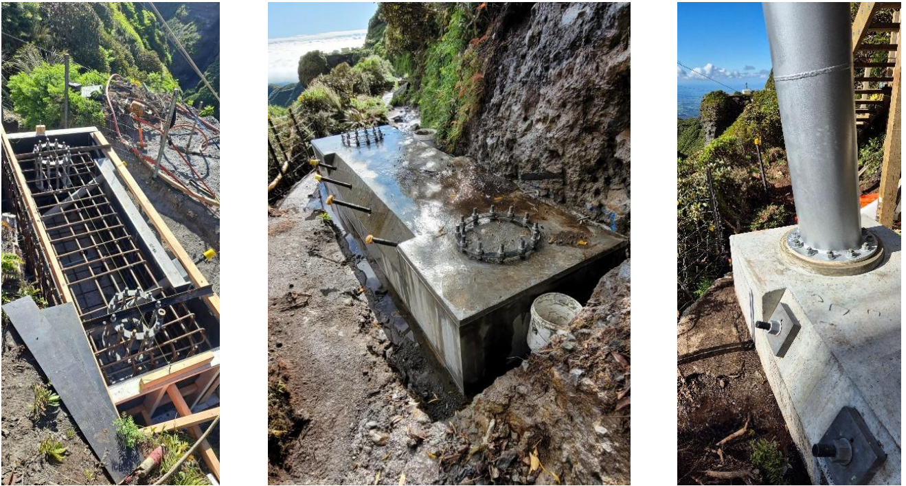
Figure 5: Mast base construction at various phases of construction
