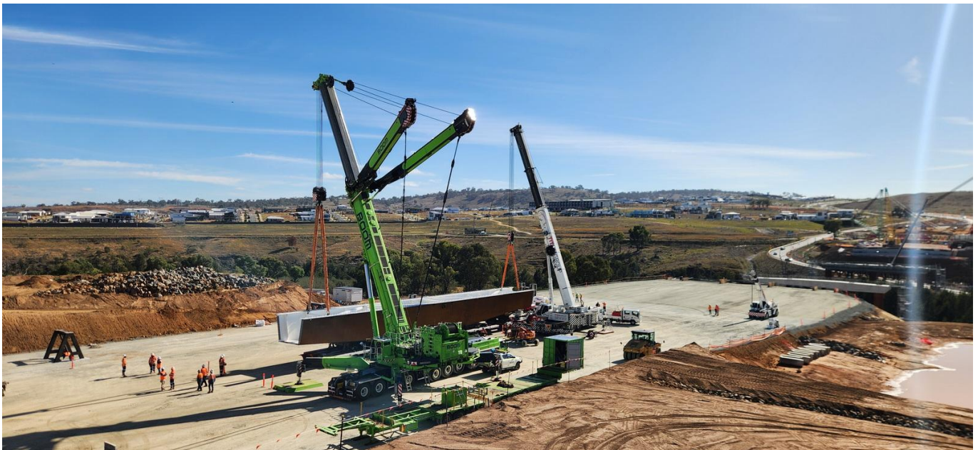
Figure 1: Lifting of a girder
