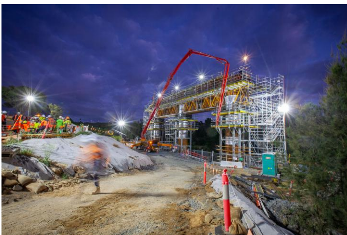
Figure 2: Pouring concrete
