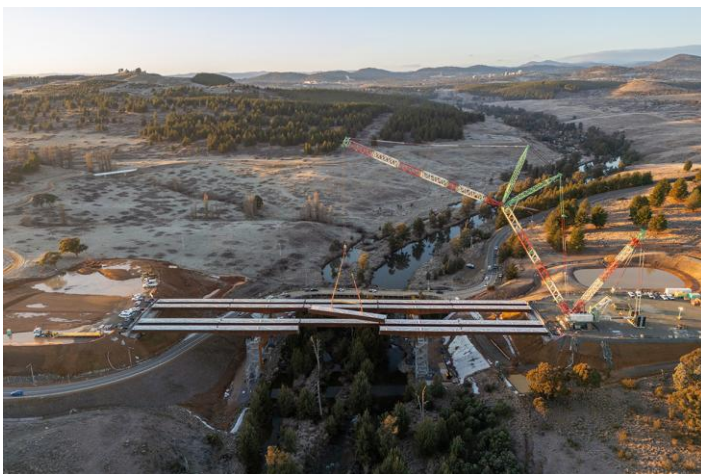
Figures 8 and 9: Installation of the midspan girder and the deck panels
