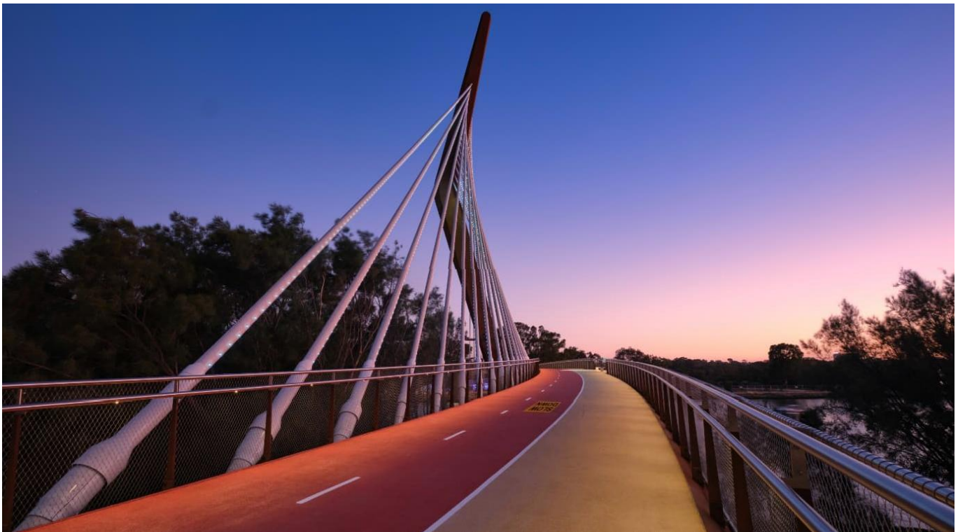
Figure 12: Bridge barriers with integrated lighting and integrated stay cable lighting system
