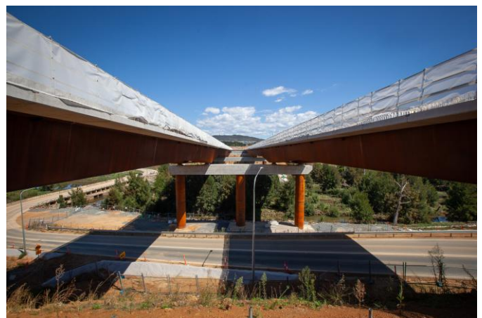
Figure 7: View of complete bridge
