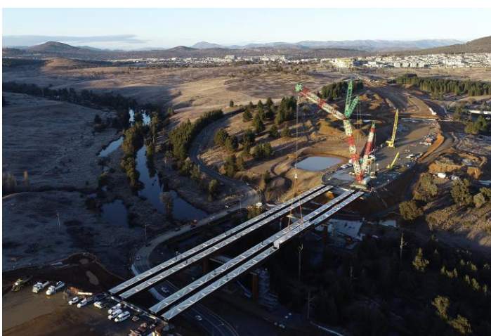
Figure 4: Installation of the last girder
