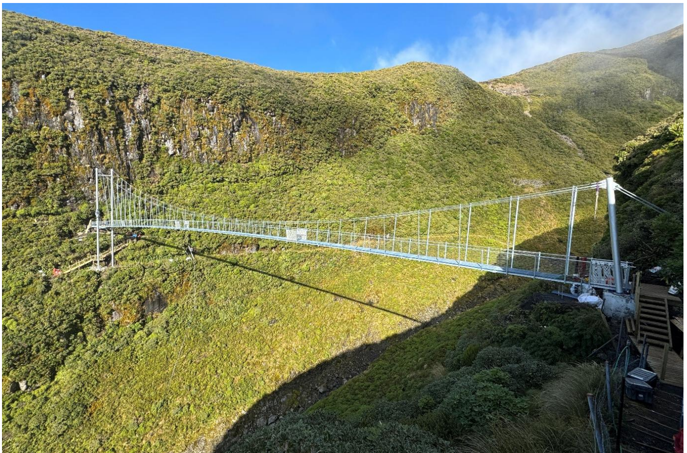
Figure 14: Completion of superstructure
