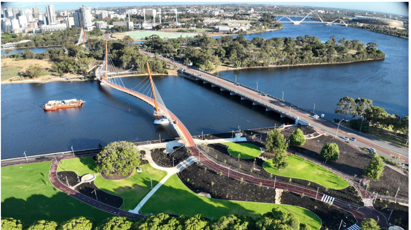
Figure 4: Aerial View of the complete Boorloo Bridge with the Matagarup Bridge
