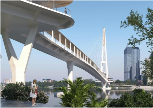
Figure 7: Typical forked pier arrangement; Architect's Rendering (left), Structural Digital Model (right)
