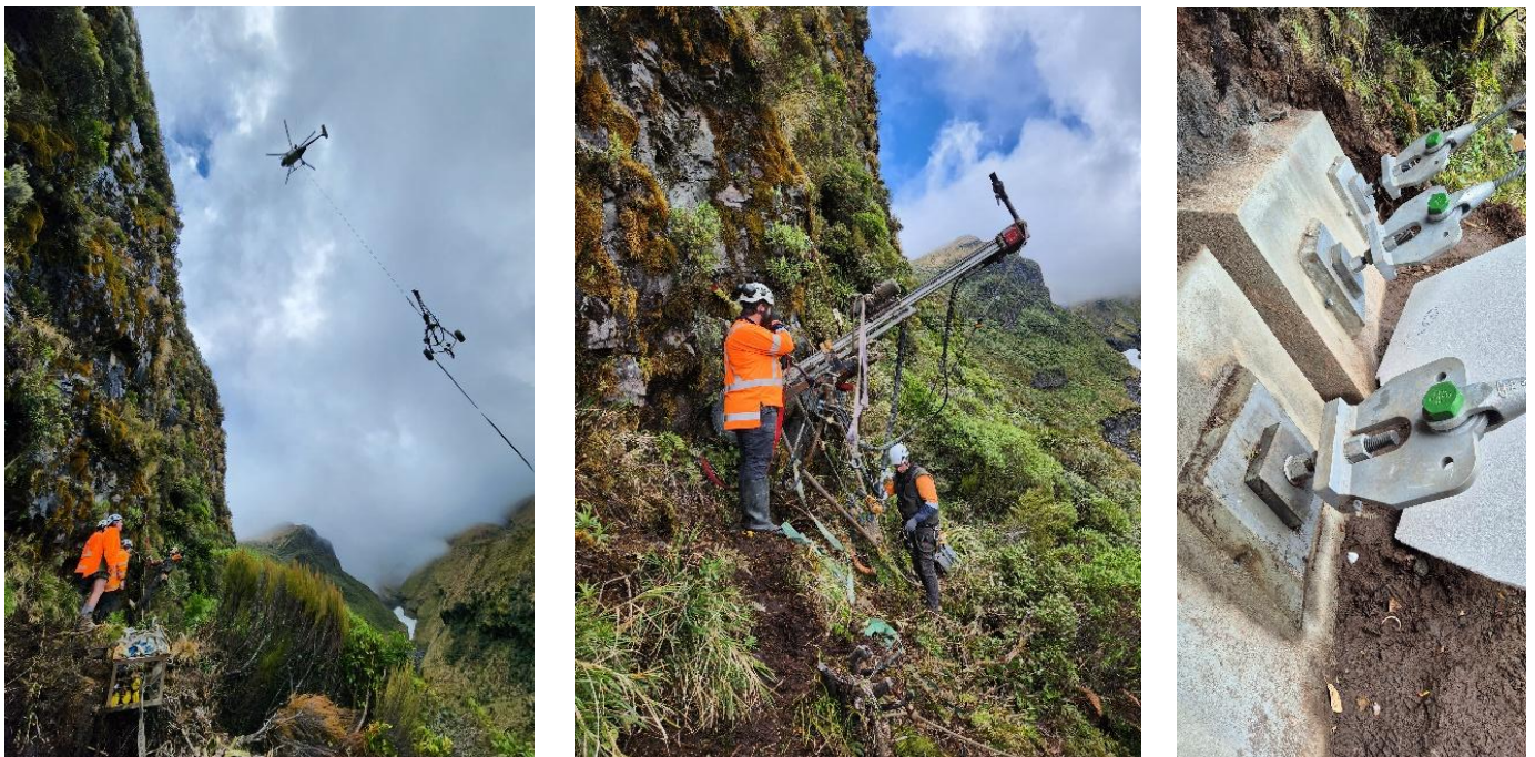
Figure 6: Helicopter delivery of the anchoring equipment, anchoring, and final outcome
