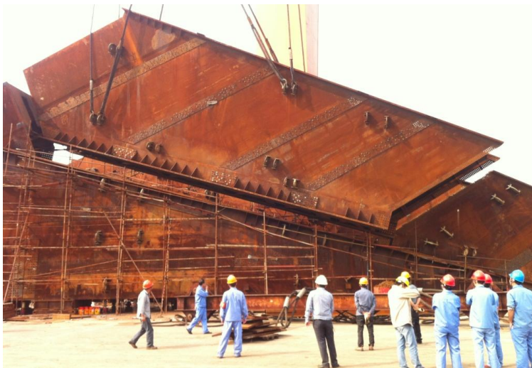
Figure 28: Fabrication and assembly of Pylon main body
