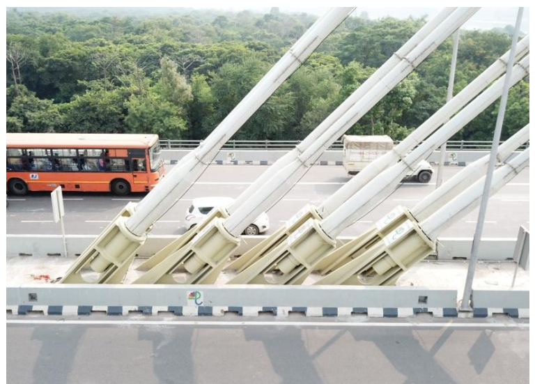
Figures 7 and 8: The main span is supported by two cable planes and the backstays are anchored in the centre of the deck
