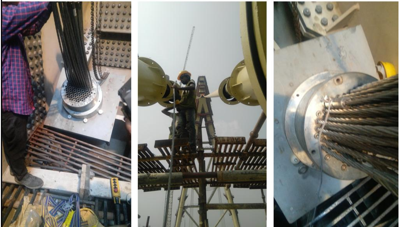
Figures 44: Cable installation & tensioning
