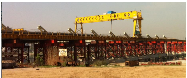
Figures 36 and 37: Erection of Deck girder using Goliath gantry
