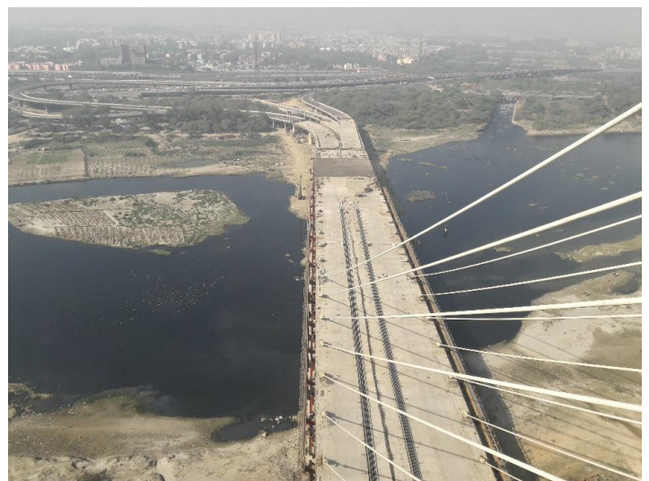
Figure 10: Signature Bridge deck and stay cables during erection
