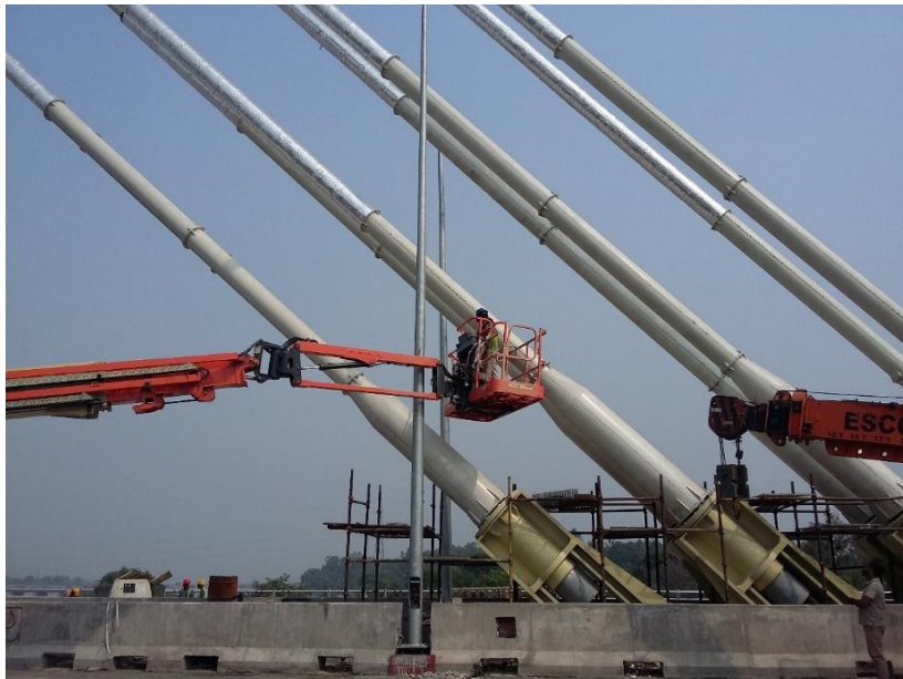
Figure 11: Fire protection over backstays
