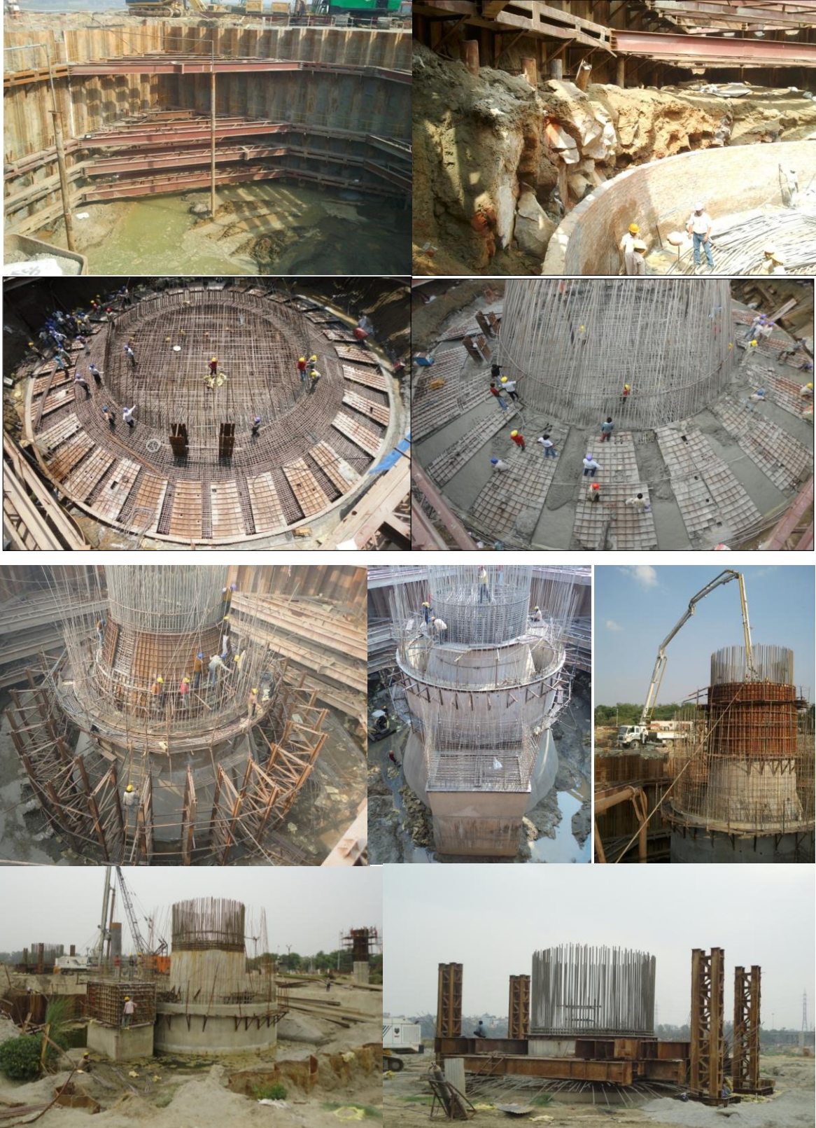
Construction of Open foundation under Pylon – P19
