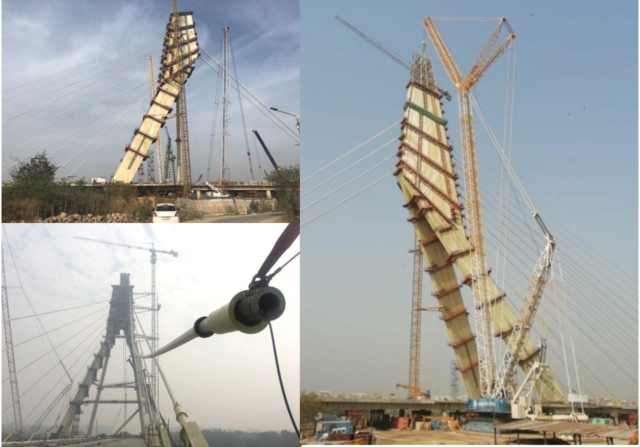
Erection of final pylon segment and Pylon Head
