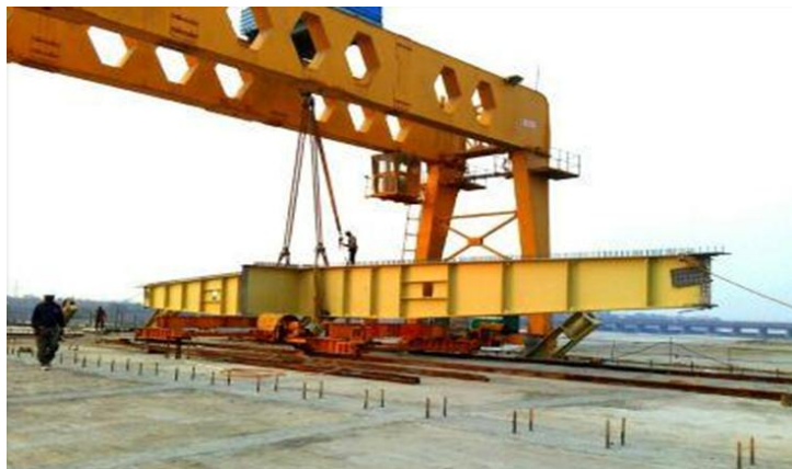
Figures 36 and 37: Erection of Deck girder using Goliath gantry
