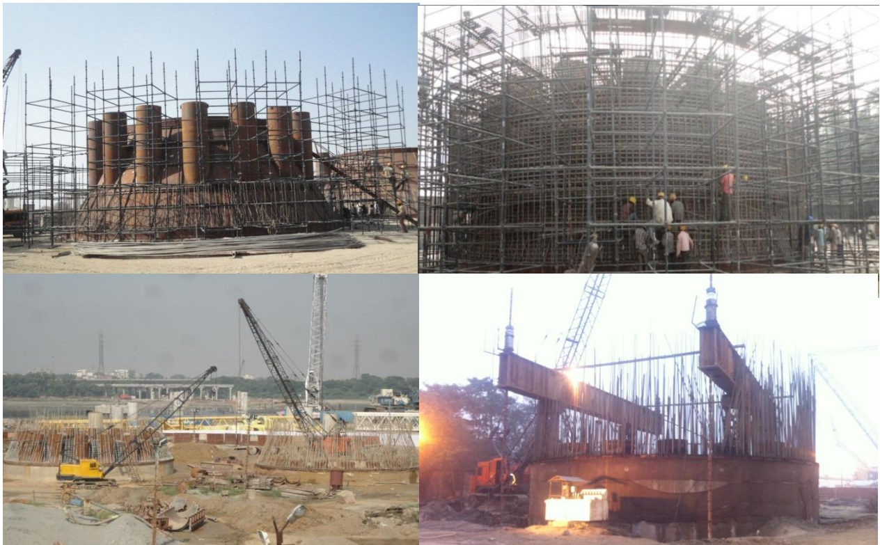
Construction of well foundation at back Stay – P23
