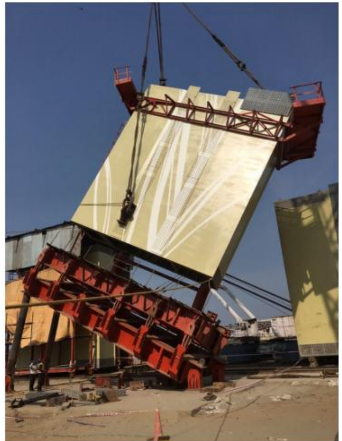
Figure 39: Rigging of a typical leg Segment
