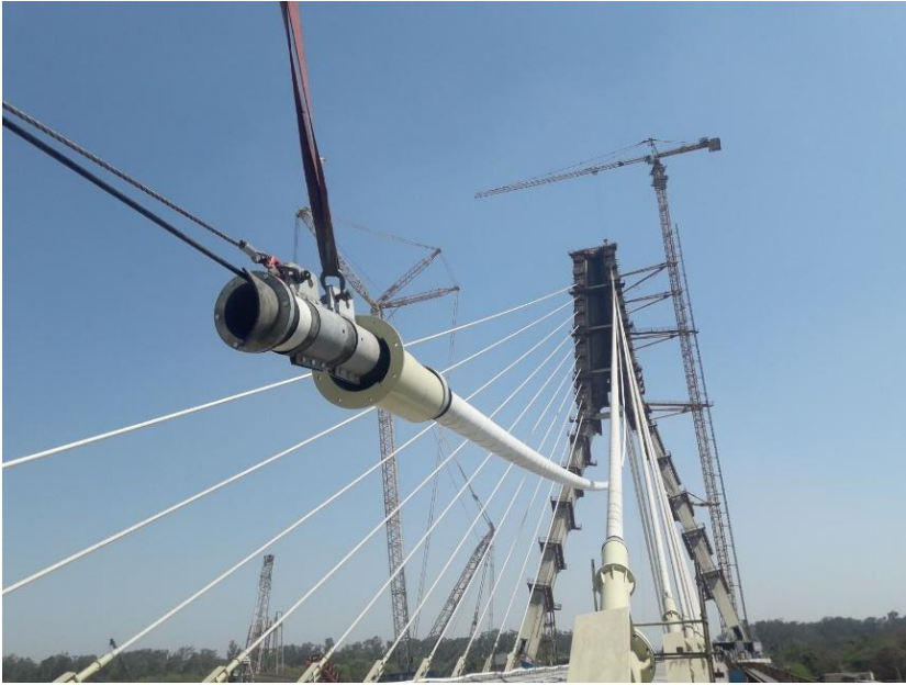
Figure 8: Front stay pipe hoisting
