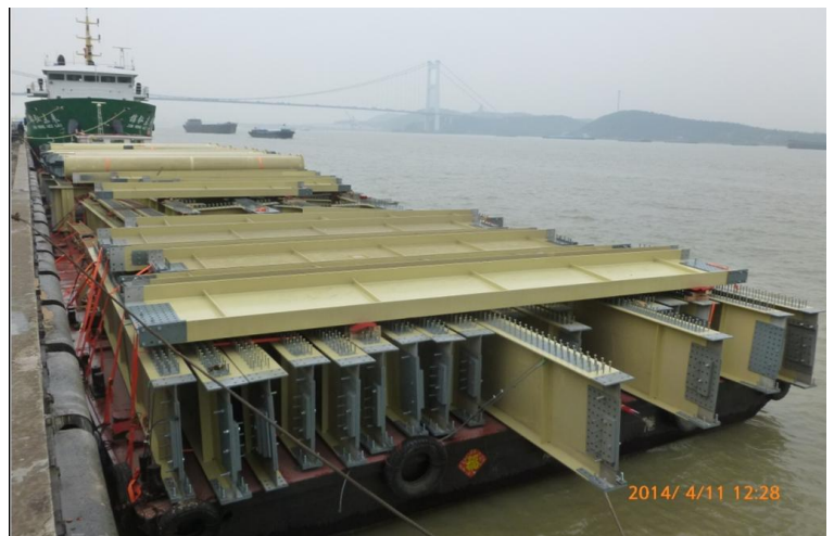
Figure 33: Loading of Segments on Barges at Workshop
