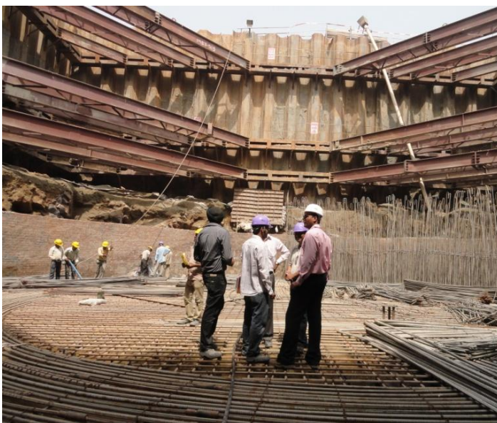
Figures 6 - 8: Sheet Pile cofferdam resting on rock with toe pinning arrangement
