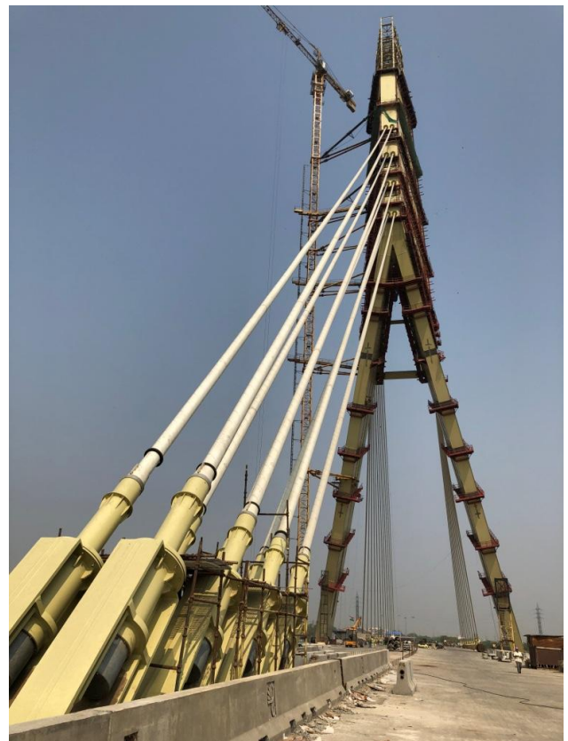
Pendulum Bearing & Back stay cable on completion
