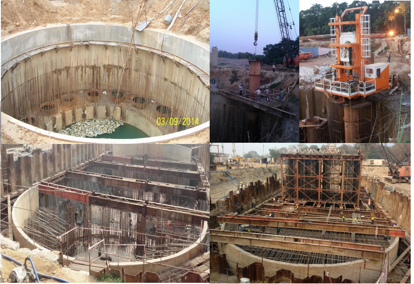
Construction of well foundation at back Stay – P23
