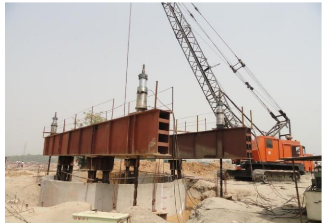
Figures 9 and 10: Well Sinking by Jack Down Method
