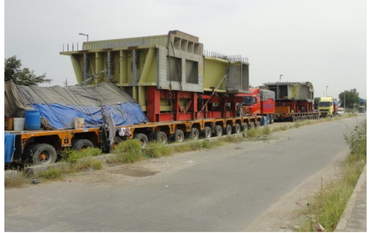
Figure 35: Transportation of Pylon base segments
