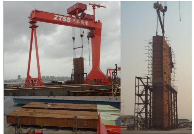
Figure 27: Vertical and Horizontal trial assembly of Pylon leg Segment
