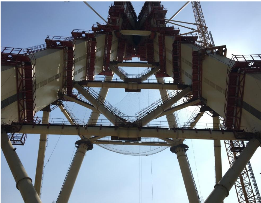
Temporary Structure supporting Pylon
