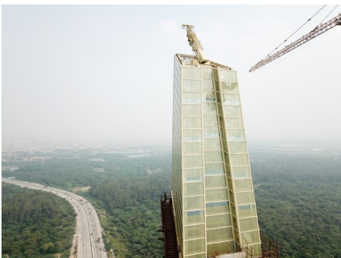
Figure 10: The glass-covered steel structure at the top of the pylon can be illuminated at night
