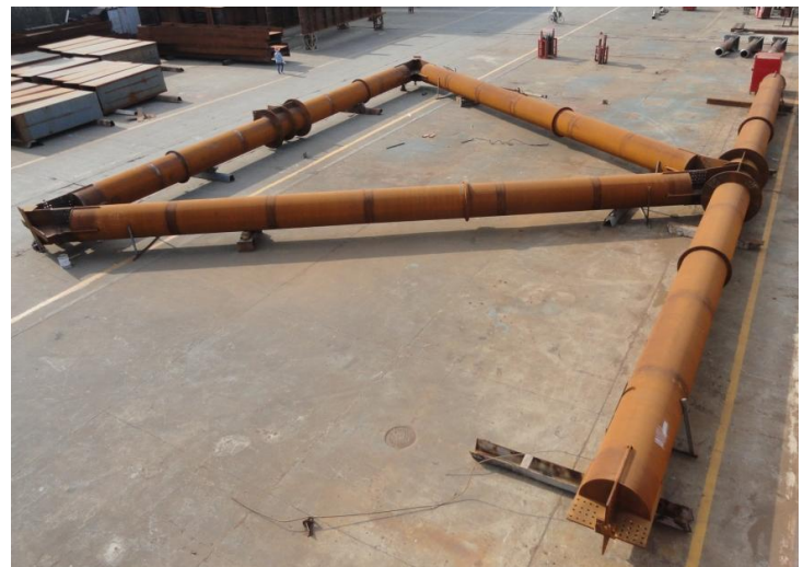
Figure 29: Trial assembly of temporary Pylon supports
