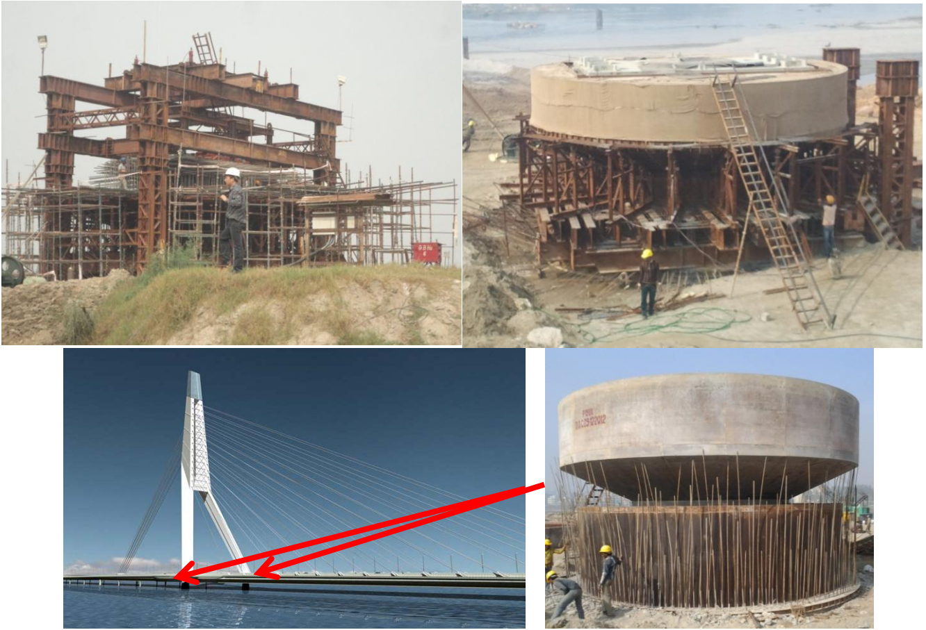
Construction of Open foundation under Pylon – P19
