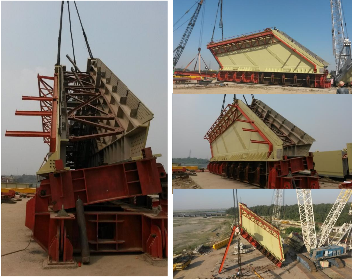
Figure 40: Rigging of a typical Main Body Segment
