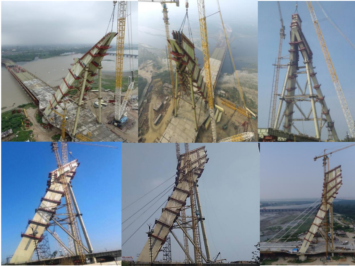
Erection of Pylon at various stages
