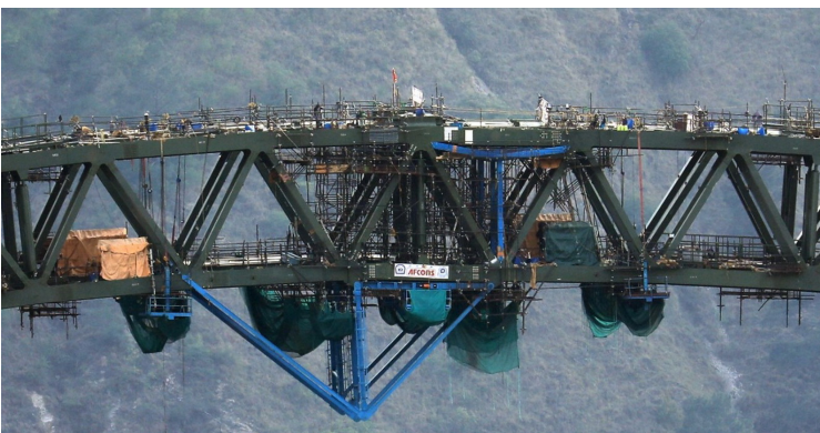
Figure 22: Photo showing Arch closure in the process: Strut C, Tripod B and Strut E (Blue colour)
