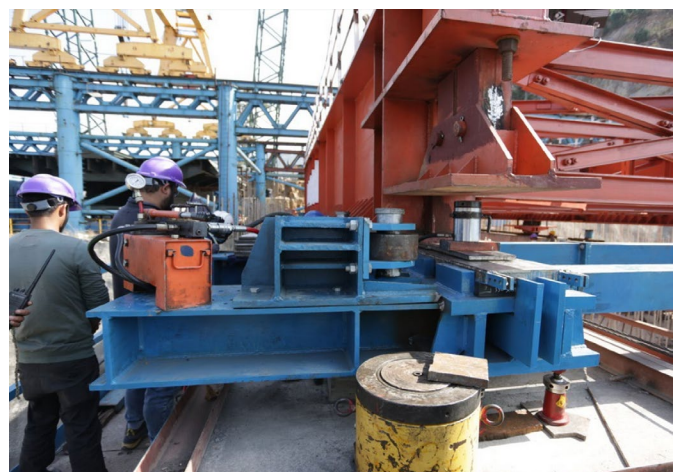
Figure 19: Tandem Bearing
