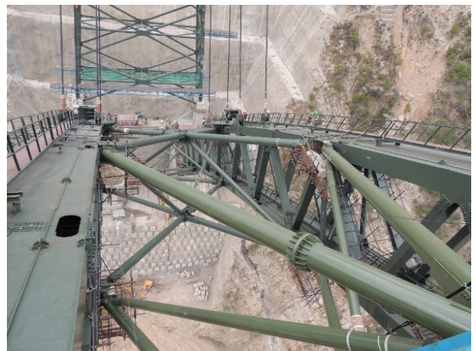
Figures 7 and 8: Arch in erection stage
