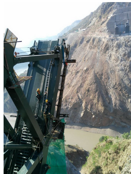
↑ Figure 8: C-Platform connected to bottom chord for longitudinal splice connection
