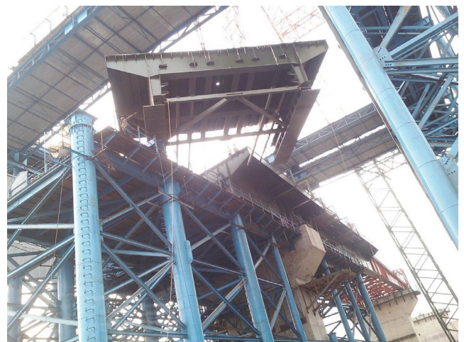
Figure 11: Rotation of segment
