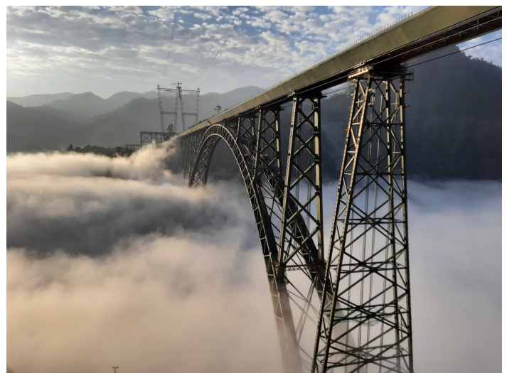
Figure 3: The Arch Bridge fully erected
