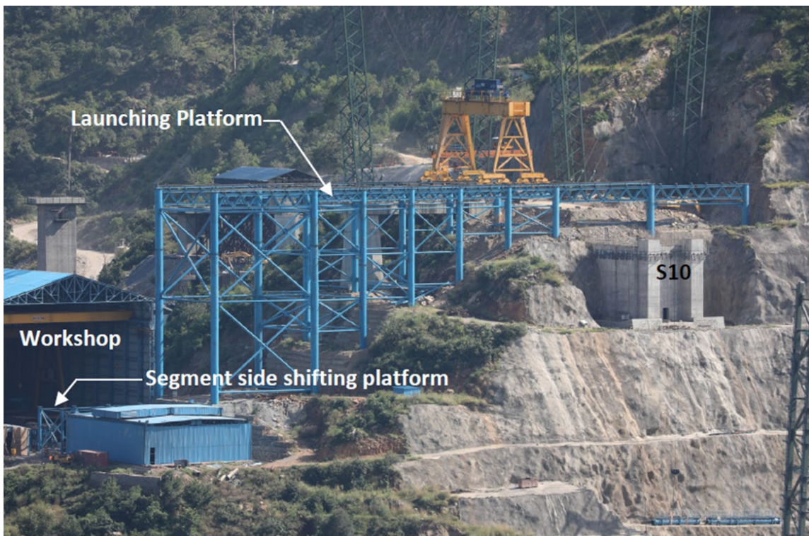
Figure 17: Temporary Platform at S10 Location
