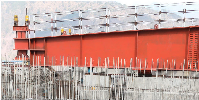
Figure 5: Launching Nose Jack (left) and Curved Launching (right)
