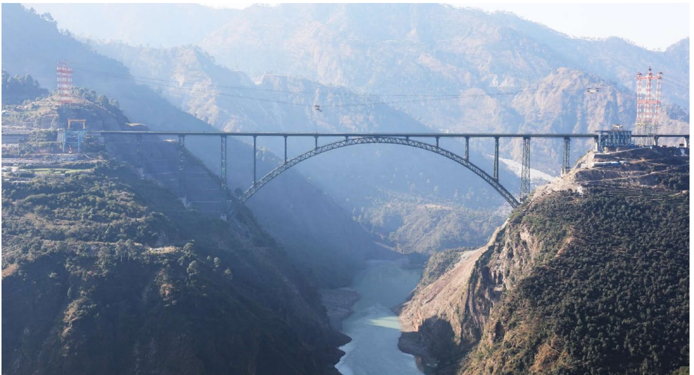
Figure 1: View of the complete Chenab Bridge
