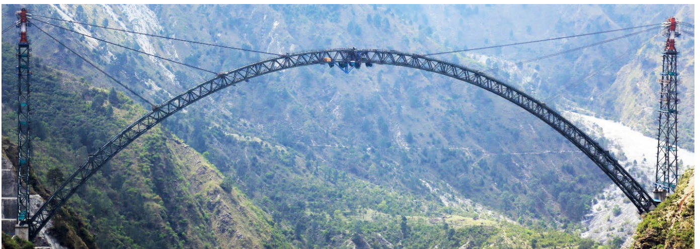
Figure 20: Arch closure in progress
