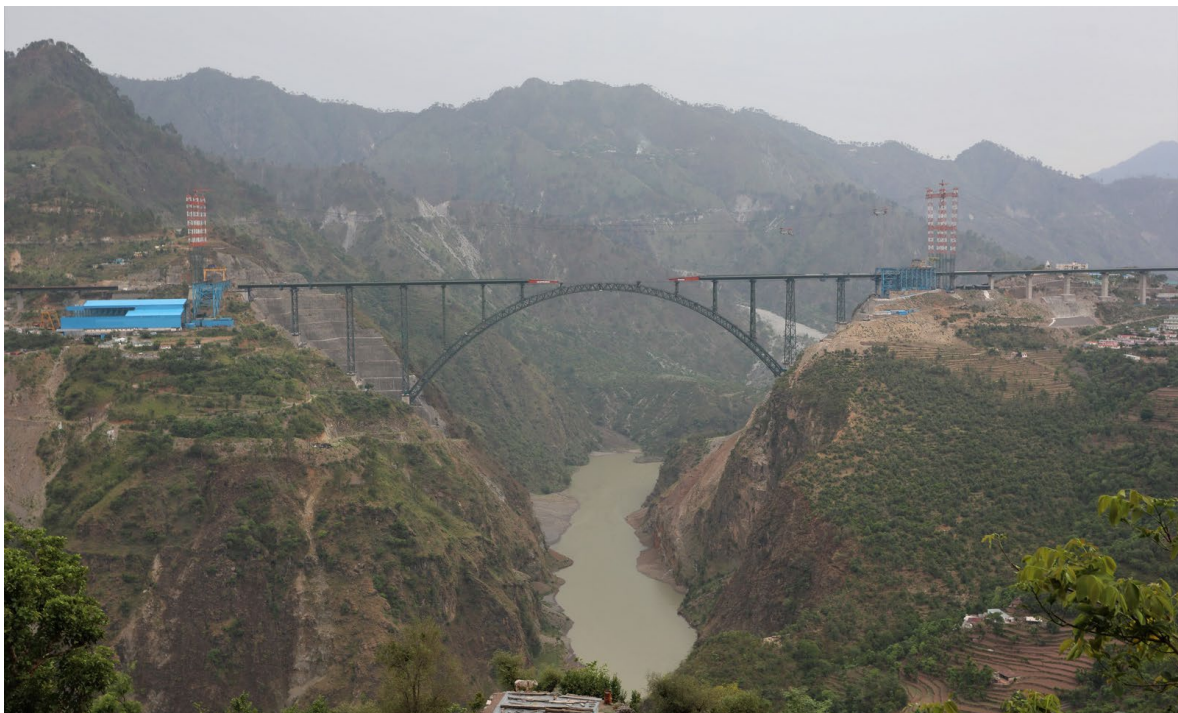
Figure 21: Deck launching over arch span
