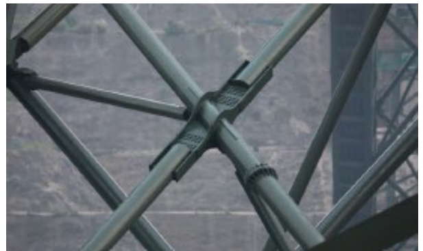
Figure 13: HSFG Bolt
