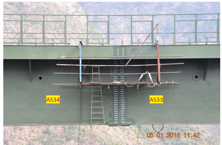
Figure 14: Splicing of segment AS33 - AS34
