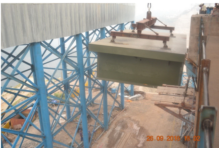
Figure 10: Segment lifting in cross direction
