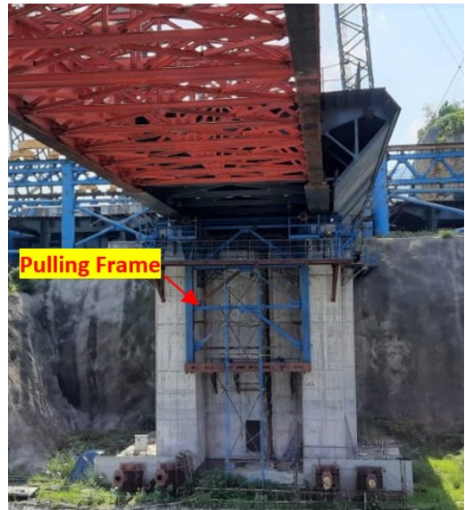
Figure 12: Pulling frame at S90 pier and S10 Abutment
