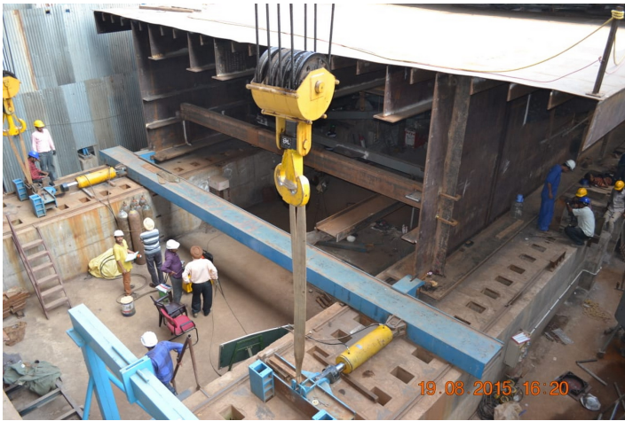
Figure 6: Push Launching arrangement behind the Abutment S180
