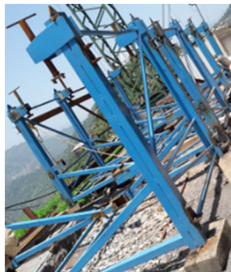
↑ Figure 8: C-Platform connected to bottom chord for longitudinal splice connection
