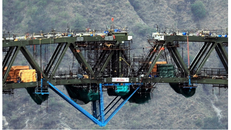
Figure 21: Photo showing Tripod "B" and Strut "C"
