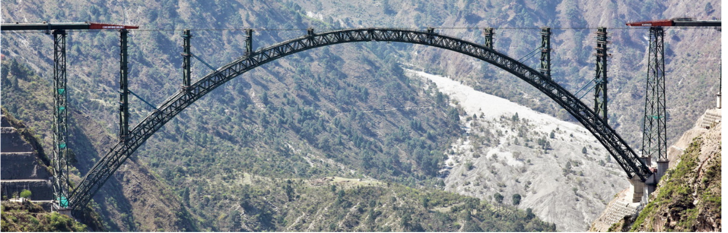
Figure 20: Launching on the arch bridge
