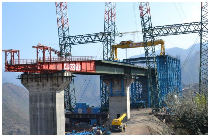
Figure 7: Launching platform at S80 location
