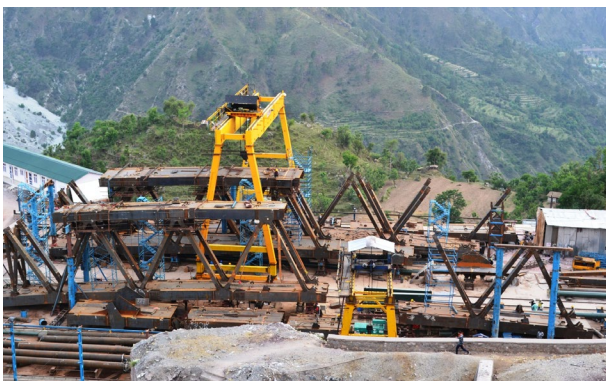
Figure 12: Arch trial assembly progress and completion for one typical span
