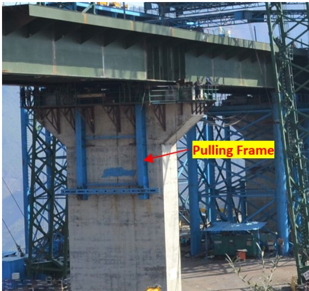
Figure 12: Pulling frame at S90 pier and S10 Abutment
