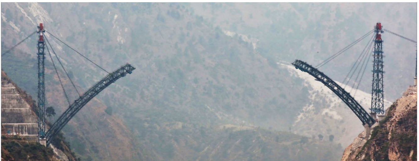
Figure 16: Arch Erection in progress from both sides
