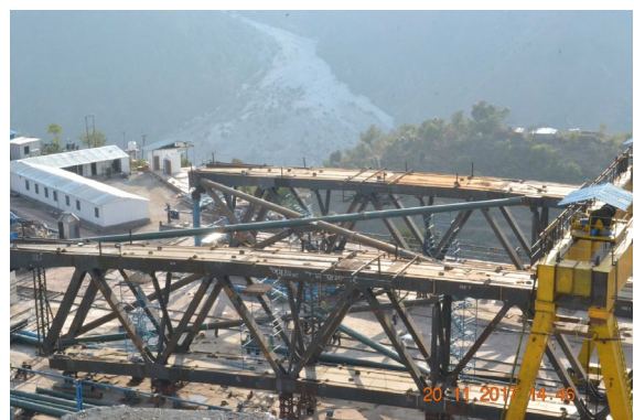
Figure 12: Arch trial assembly progress and completion for one typical span
