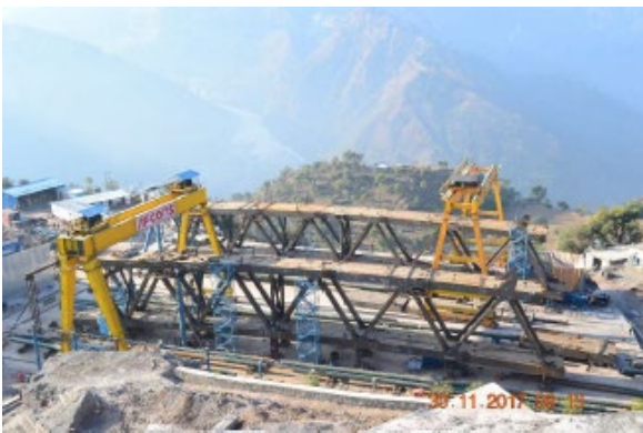
Figure 11: Trial assembly of the arch on the ground
