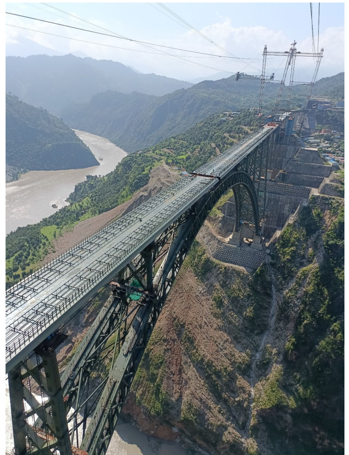
Figure 10: Chenab Bridge, almost completed
