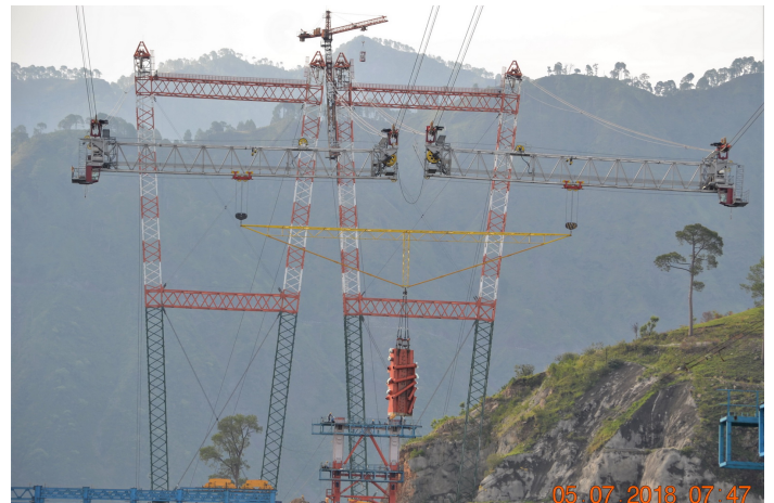
Figure 3: Crossbar cable crane
