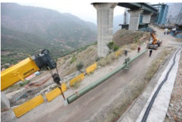
Figure 12: Transportation of wind bracings
