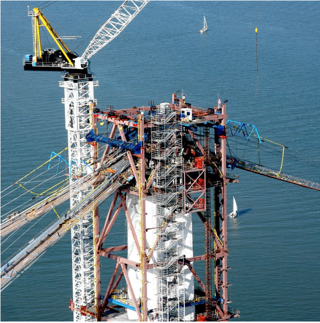
Tower and cable erection
