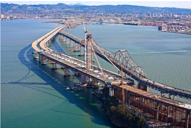
Aerial view of the tower under construction
