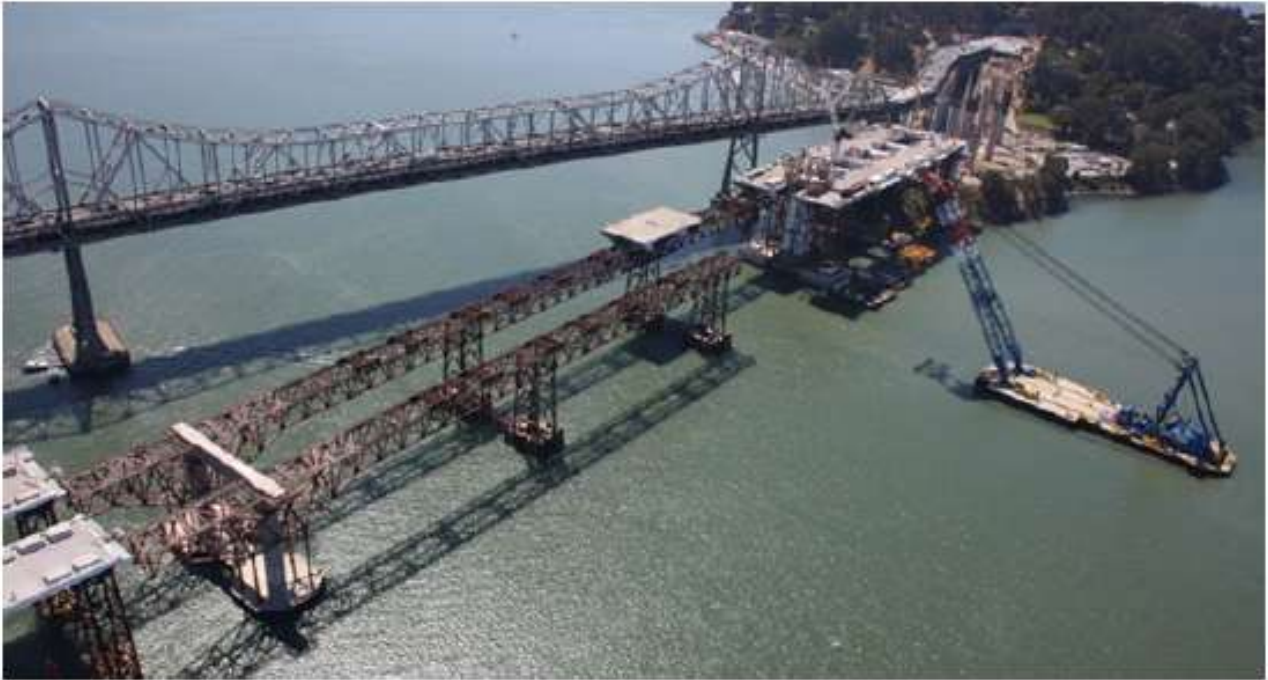
Figure 19: Temporary truss falsework
