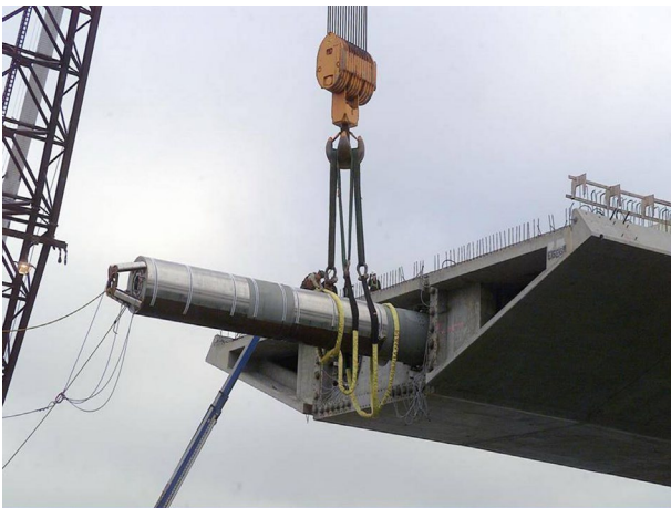
Hinge pipe beam installation
