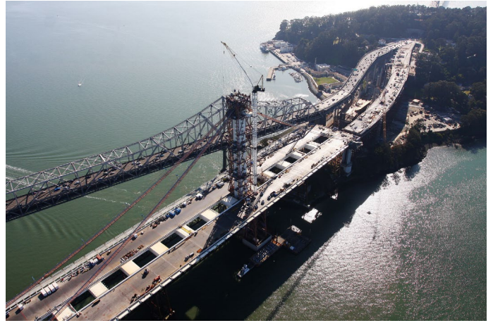
Facing west construction
