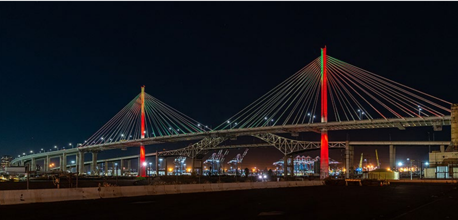
Figure 1: Night View of the complete Bridge
