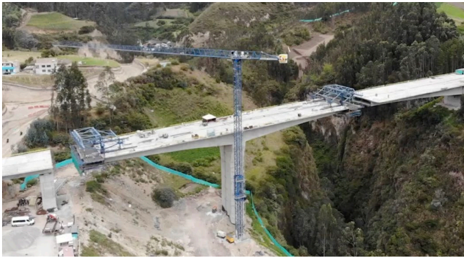
Figures 14 and 15: Formwork travellers on the Boquerón Bridge
