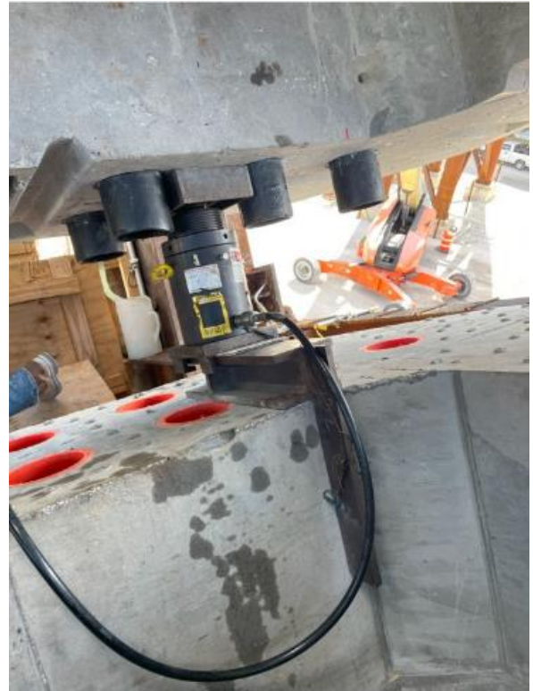
Figure 15: Alignment jacks at the wet-joint between the starter and precast segment
