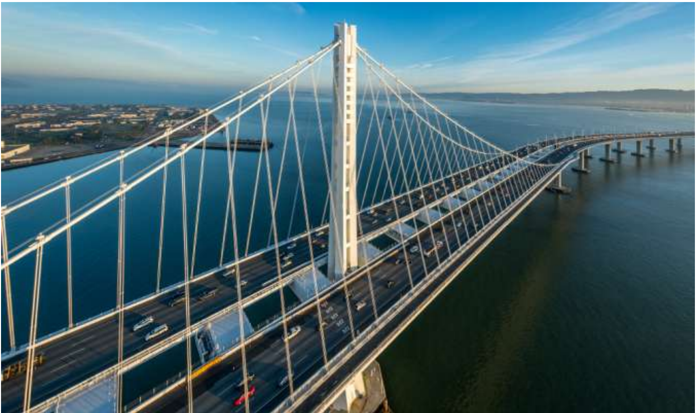
Figure 1: San Francisco-Oakland Bay Bridge over the San Francisco Bay. Source: Sam Burbank
