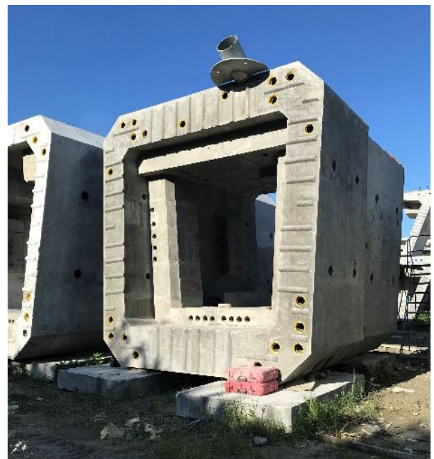
Figure 26: Suspender segment showing suspender pipe. Segments are cast and stored upside-down.
