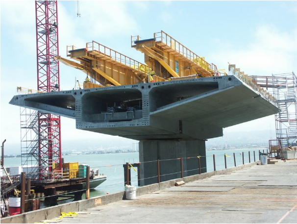
Skyway precast segment at port
