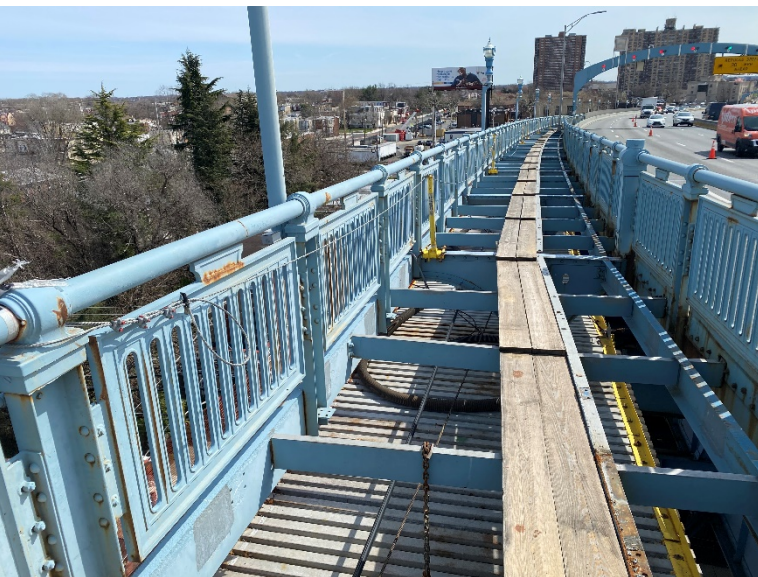
Figure 15: Temporary platform above the PATCO track envelope, existing walkway components demolished
