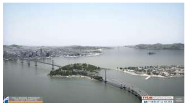
Figure 20: Animation of Load Transfer of San Francisco-Oakland Bay Bridge Self-Anchored Suspension Bridge by TYLin and partners for the Toll Bridge Program Oversight Committee
