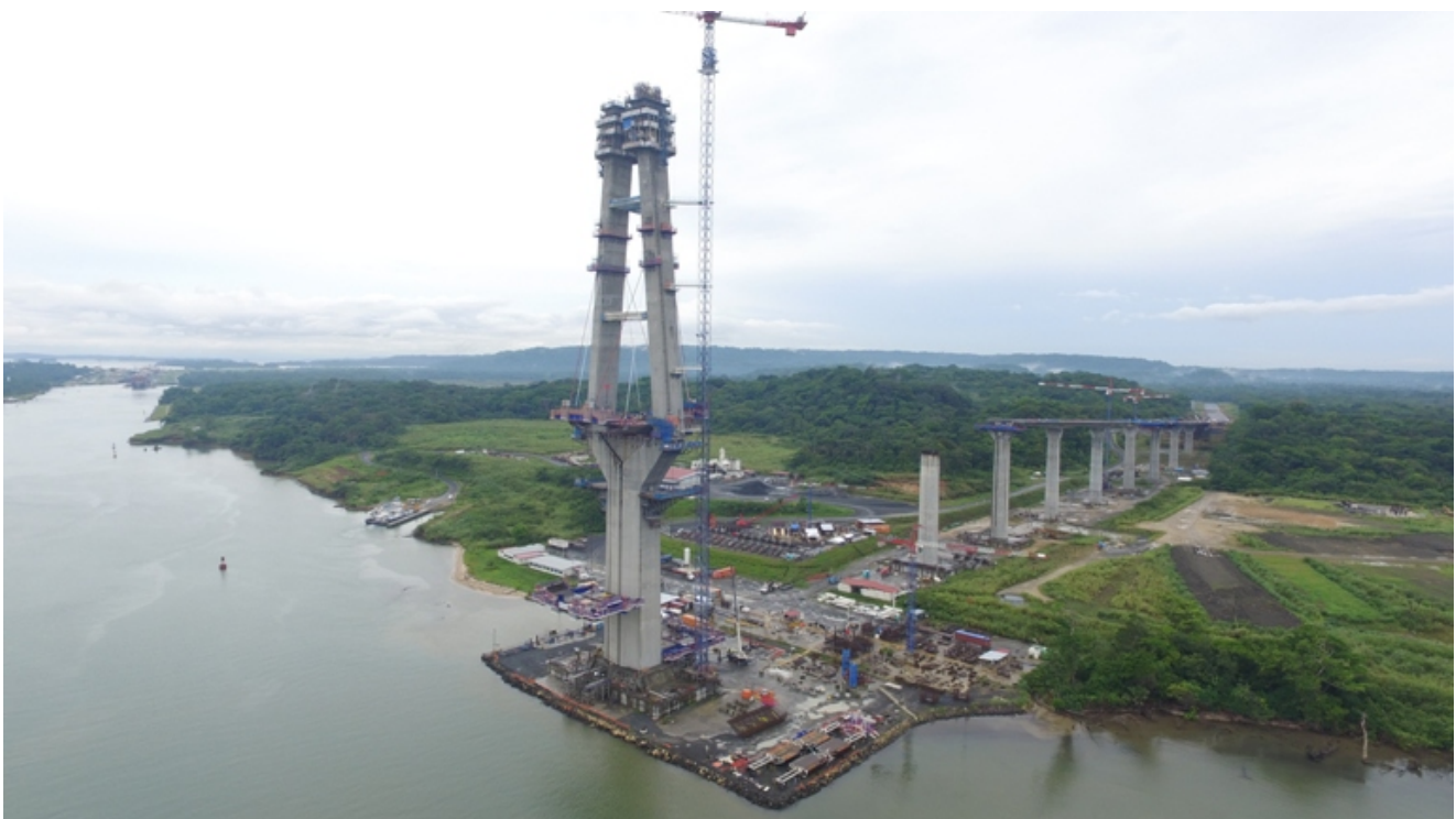
Figures 3: The Bridge during construction
