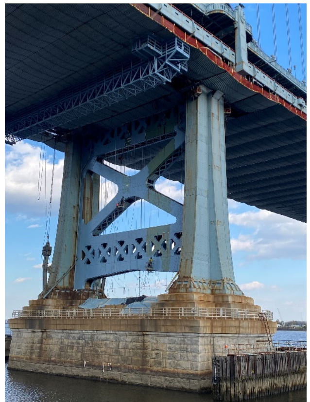
Figure 10: Lower tower strut overcoat painting
