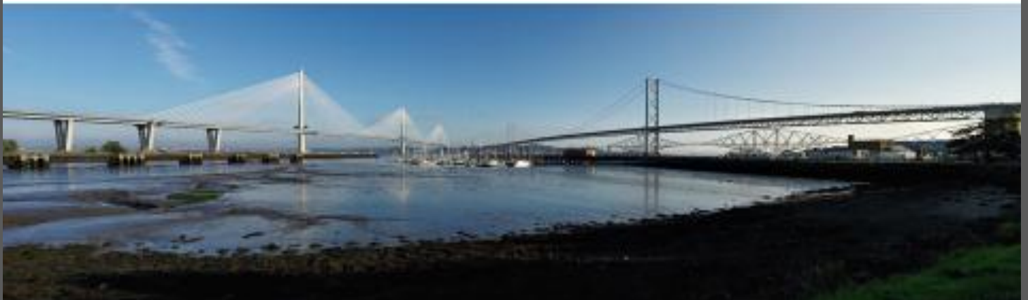
Queensferry Crossing Scotland
