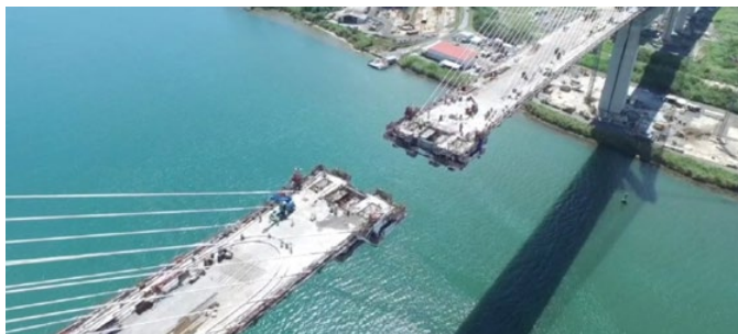
↑ Figure 8: Formwork travellers in full configuration and during typical operation
