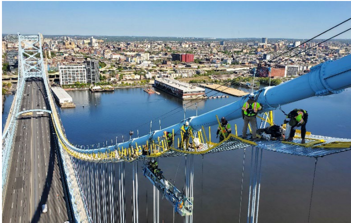
Figure 6: Main cable access platform installation
