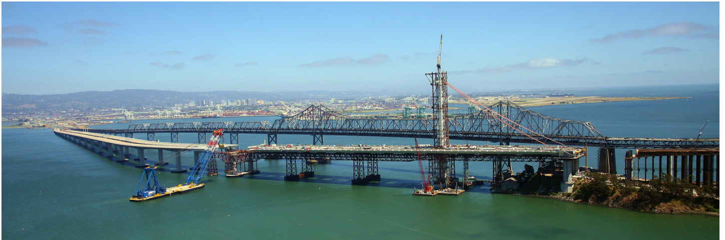
Panoramic view of the SAS bridge under construction
