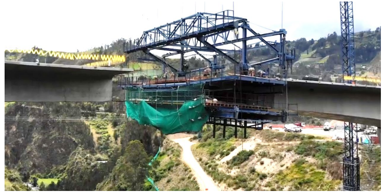
Figures 14 and 15: Formwork travellers on the Boquerón Bridge
