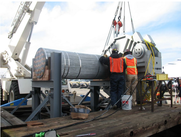
Cable compaction trial
