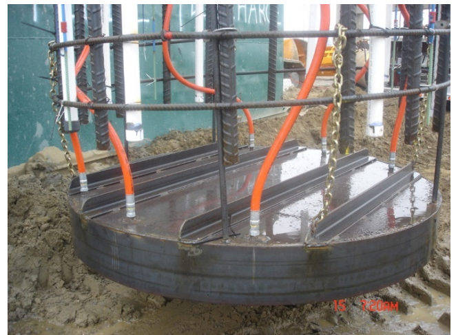
Figure 18: Illustration of the effects of base grouting. Image courtesy of Arup
