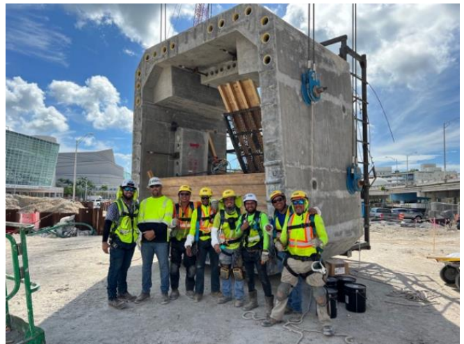
Figure 30: Segment erection crew. Credit: FDOT & I395-Miami.com
