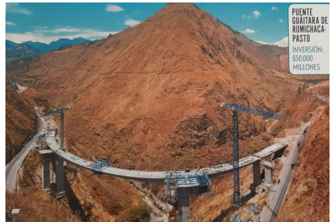
Figure 22: The Guaitara Bridge
