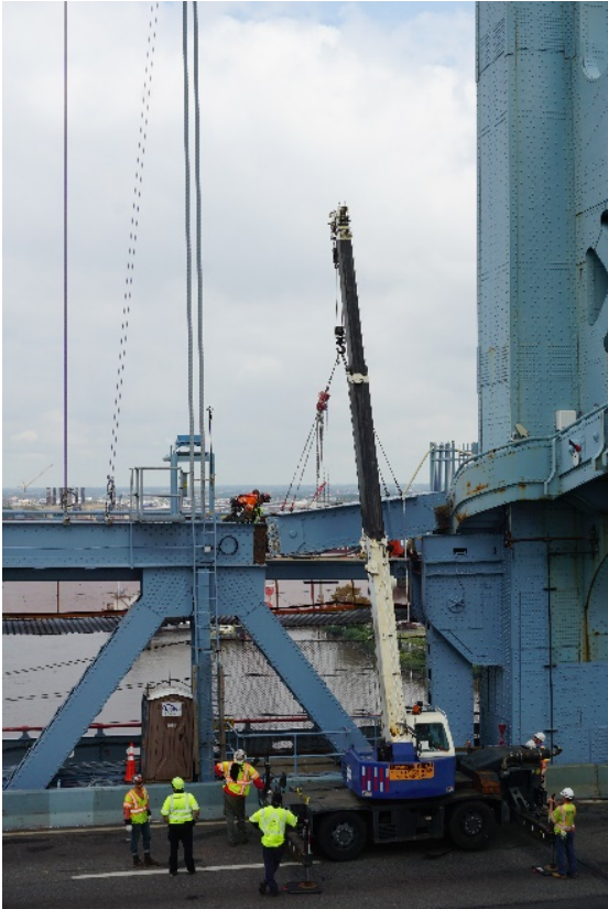
Figure 11: Removal of stiffening truss top chord
