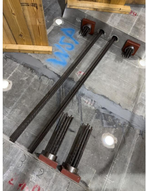
Figures 10 - 12: ↻ Temporary erection tendons at the interior of the top / 'extrados' flange of the arch rib.
