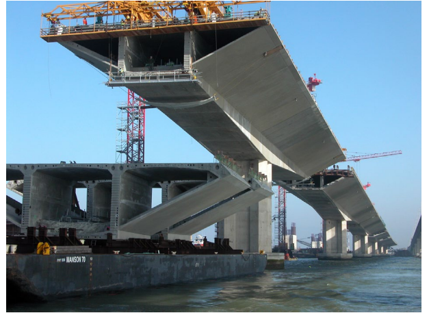
Erection of Skyway superstructure
