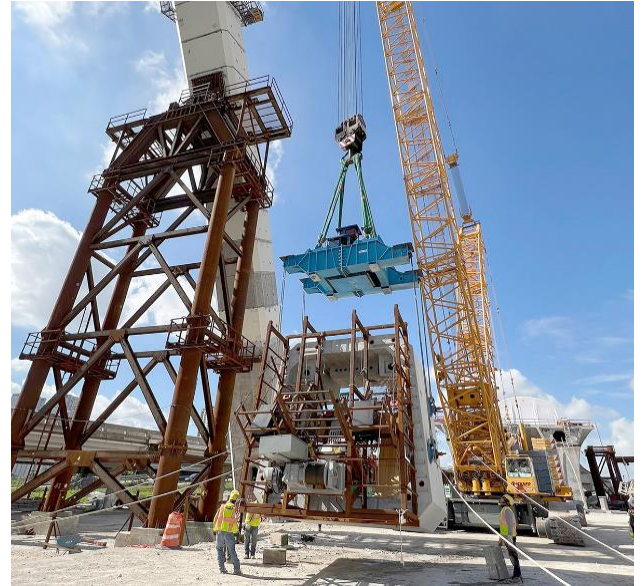
Figure 21: Segments erected in progressive cantilever from tower to tower
