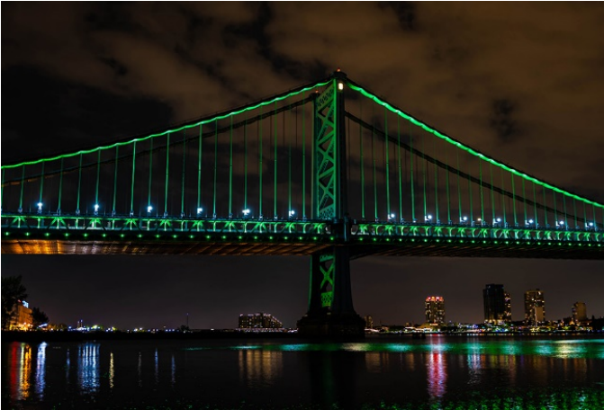
Figure 13: North Cable decorative lighting commissioned in Spring 2023
