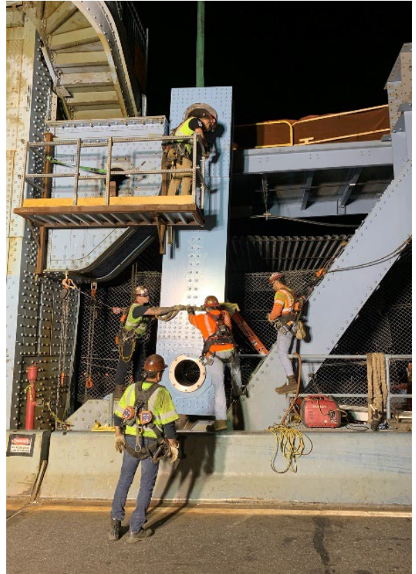
Figure 12: Placement of new stiffening truss end link
