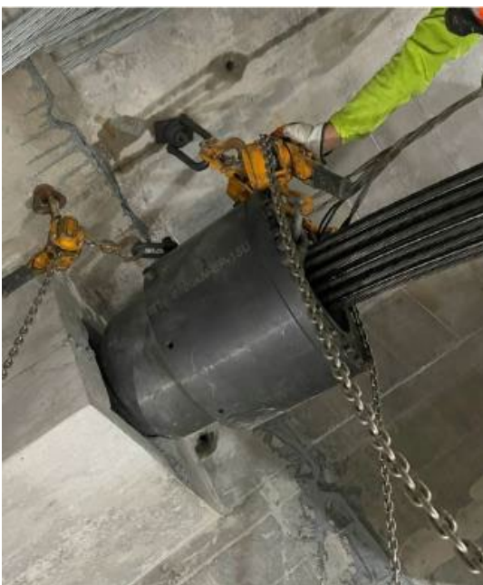
Figures 18 and 19: Permanent post-tensioning installation and stressing
