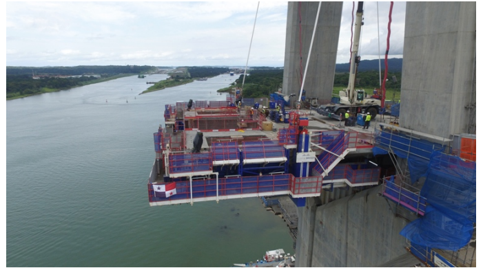
Figures 6 and 7: Casting of the first deck segments
