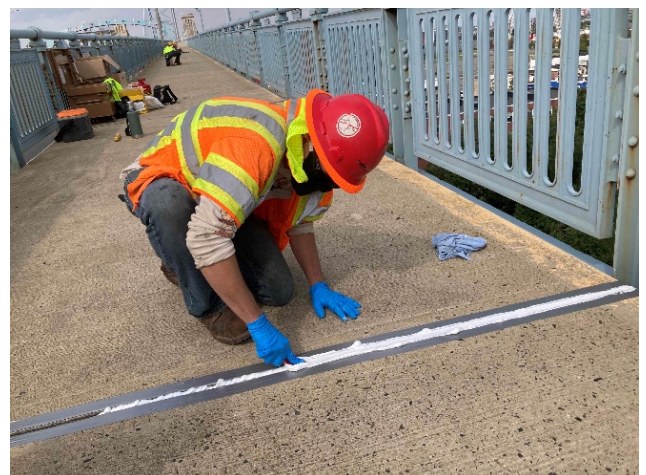
Figure 8: Expansion joint replacement
