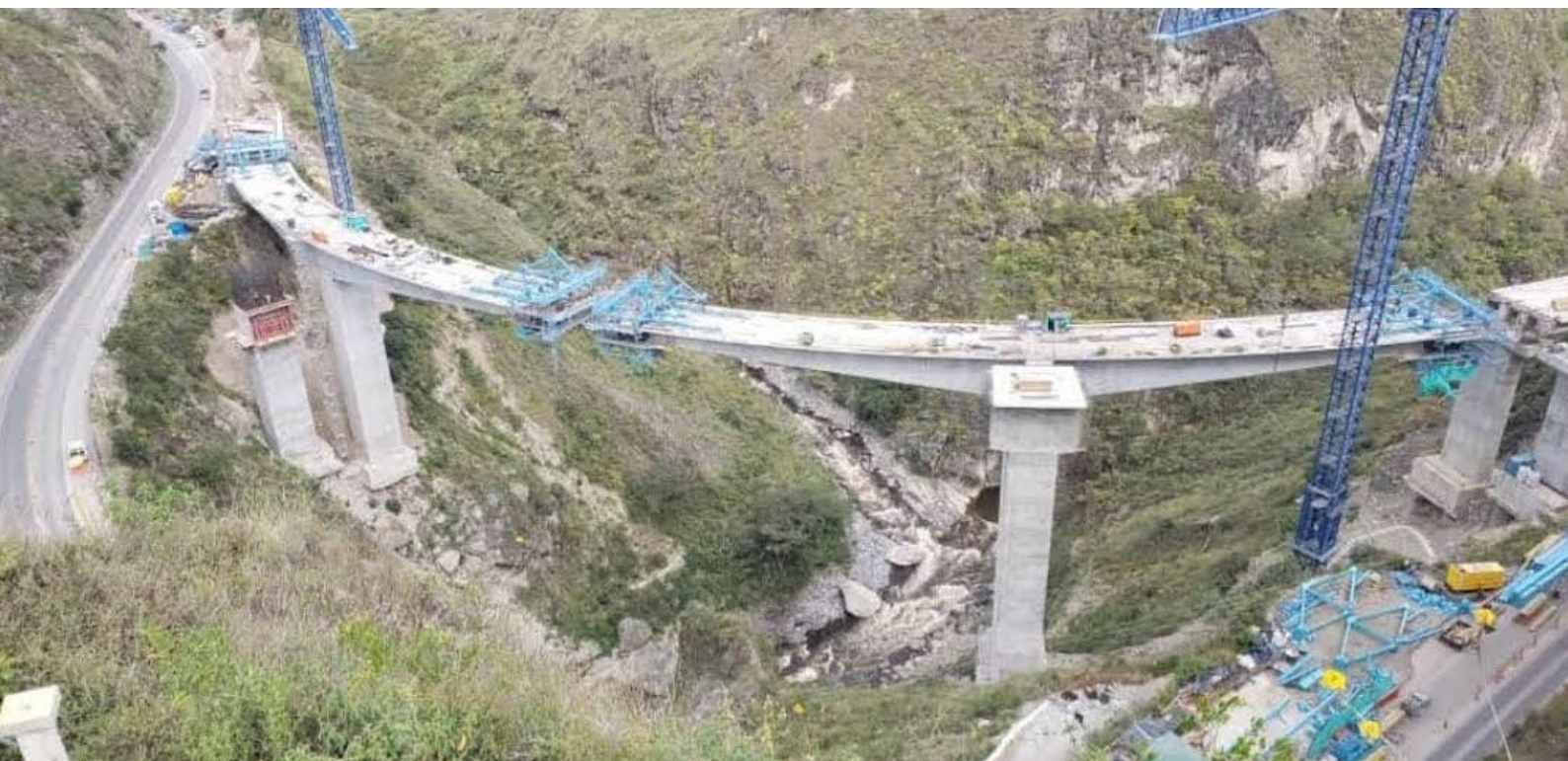
Figure 1: Cantilever overhead formwork system for the Guaitara Bridge, Colombia
