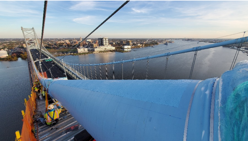
Figure 4: ↑ Elastomeric wrapping material during installation → Installed wrapping with wedge seal detail at each cable band and anti-skid walking surface
