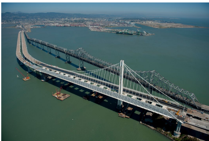
Aerial view of the completed new SAS bridge with the original bridge behind
