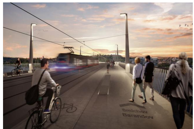
Figure 21: Combined Lighting/Tram Poles and railings
