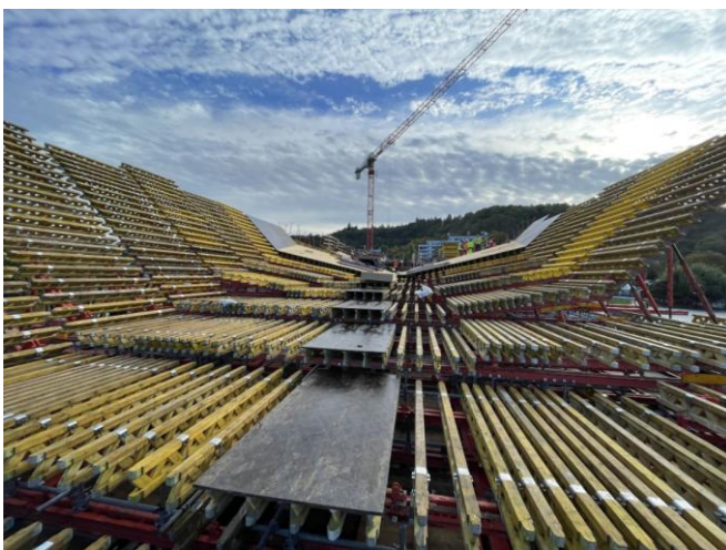
Figure 30: Superstructure formwork of stage 5 (PERI)
