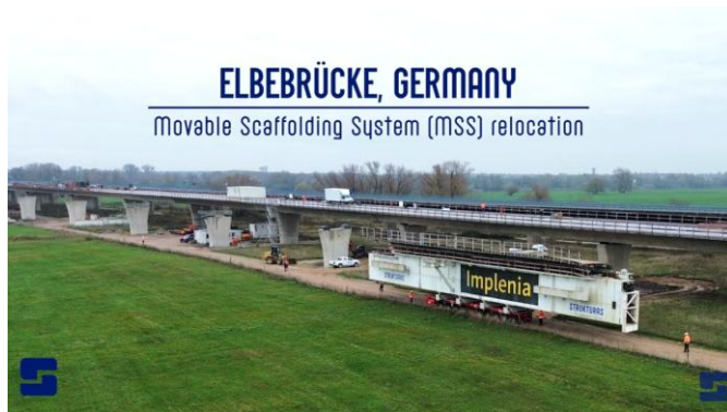
Elbebrücke MSS relocation using underslung MSS with tower crane
