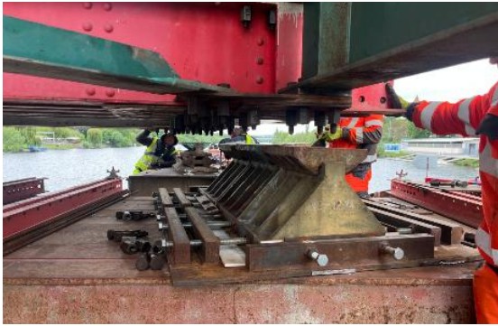
Figure 10: Installation of the temporary structure onto bearings
