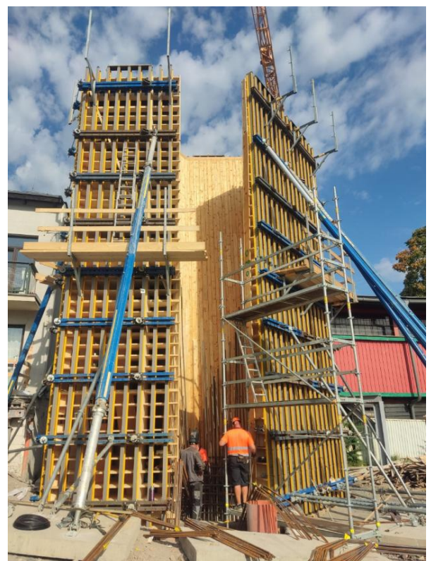
Figure 13: Formwork of pier P3
