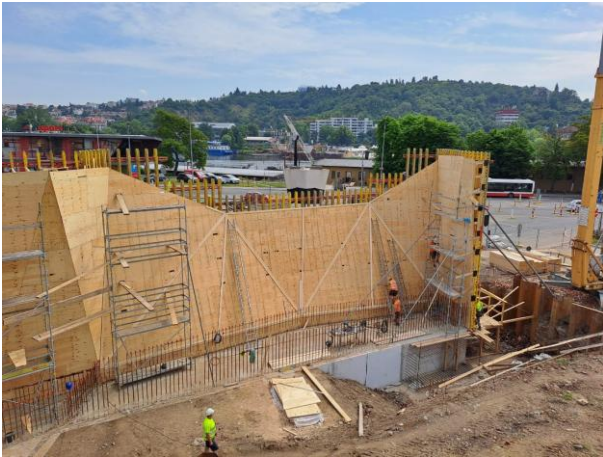
Figure 10: Formwork of abutment O1
