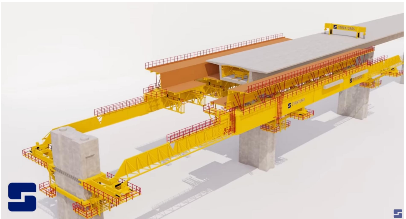
Figure 10: General view of the underslung Movable Scaffolding System during launching
