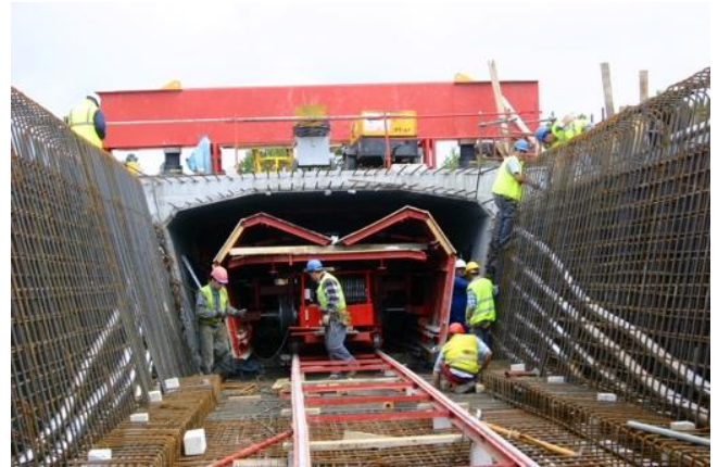
Figure 7: Mechanised transport of the internal formwork in a box girder deck
