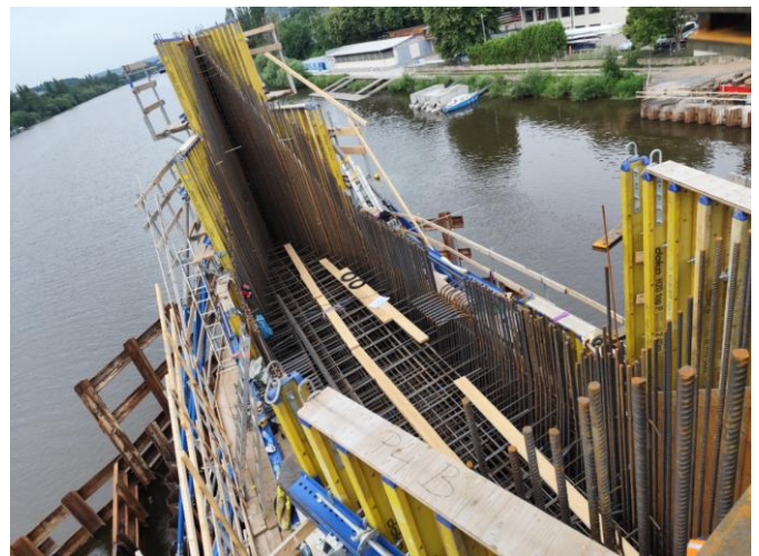
Figure 20: Complex reinforcement of pier P4
