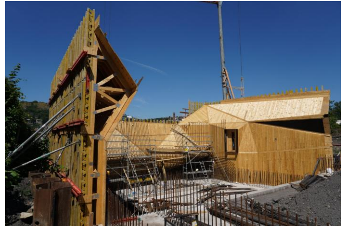
Figure 11: Formwork of abutment O7
