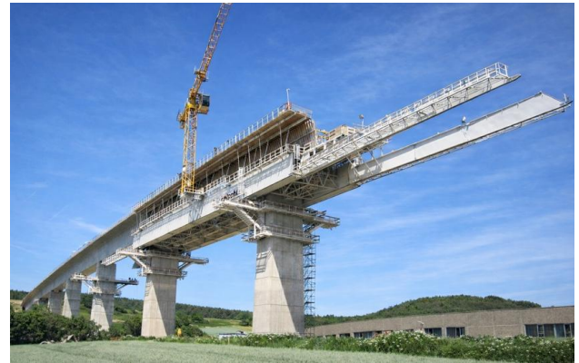
Figure 2: General view of an Underslung Movable Scaffolding System equipped with a tower crane
