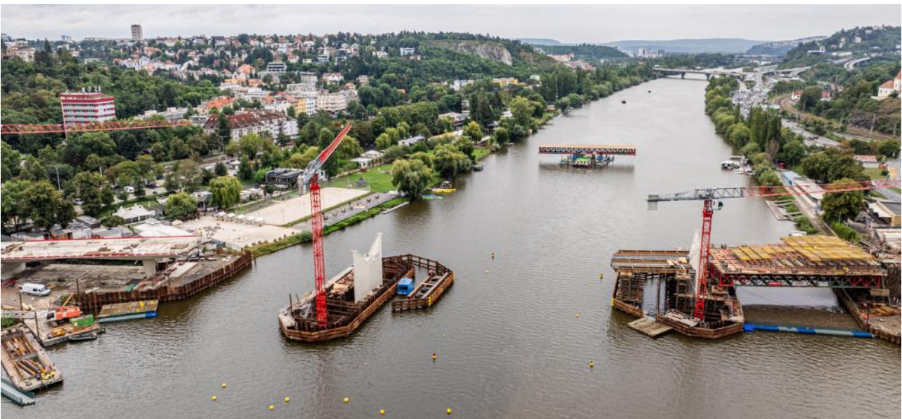
Figure 1: Dvorecký Bridge under construction
