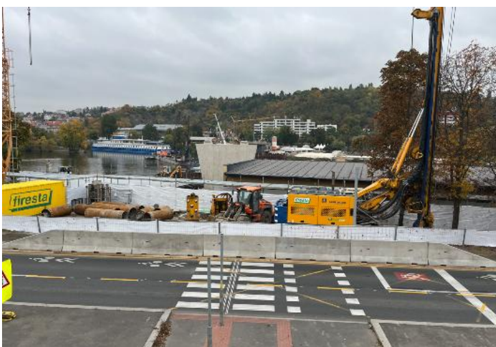
Figure 4: Foundation of temporary trestle Pi2
