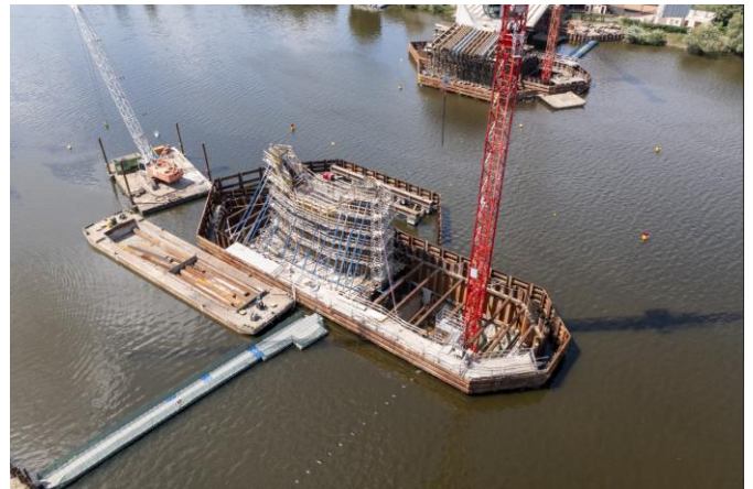
Figure 15: Formwork of pier P5
