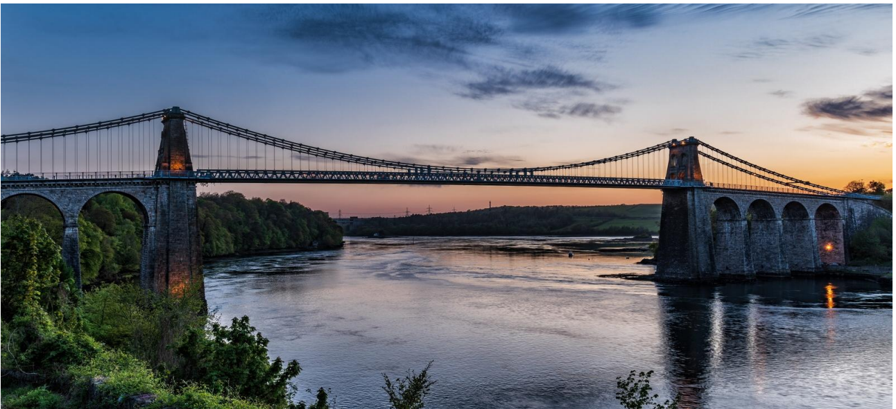
Figure 1: The Menai Suspension Bridge was the first to span the Menai Strait, connecting Anglesey to mainland Wales
