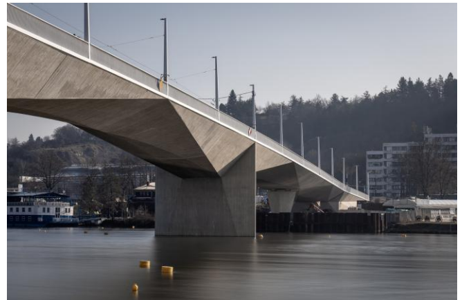
Figure 21: Completed bridge view
