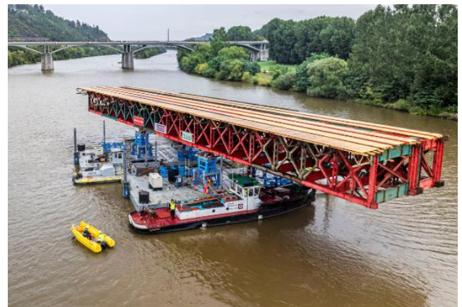
Figure 29: Temporary supports - transport
