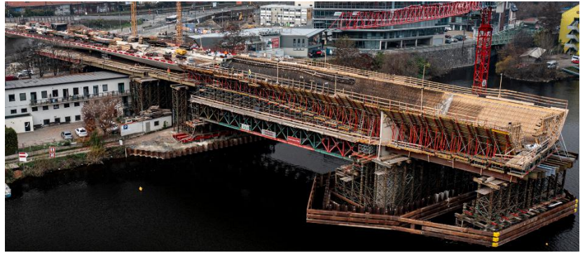
Figure 11: Concreting Stage 4 – temporary structures
