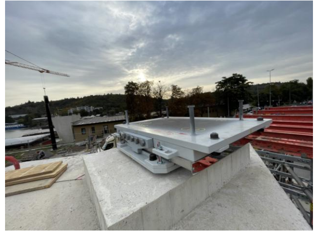
Figure 18: Spherical bearing P2P
