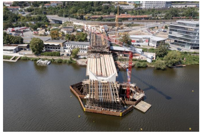
Figure 27: Temporary support structure of stage 4
