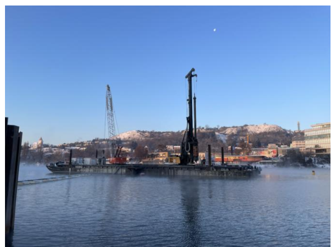
Figure 6: Pile drilling at pier P5
