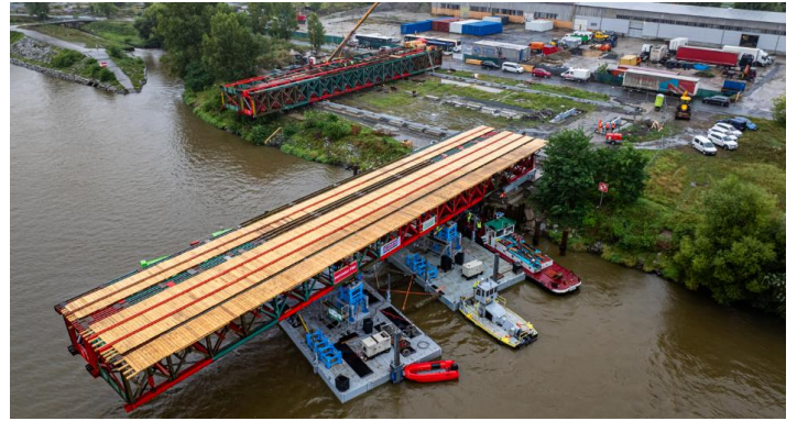
Figure 9: Temporary support structures in Velká Chuchle
