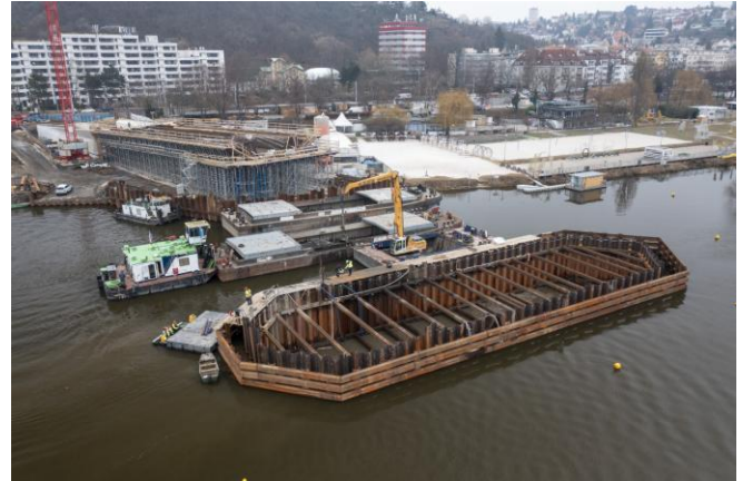
Figure 9: Sealed cofferdam of pier P5
