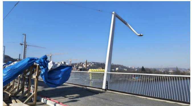
Figure 36: Railing and atypical column no. 133
