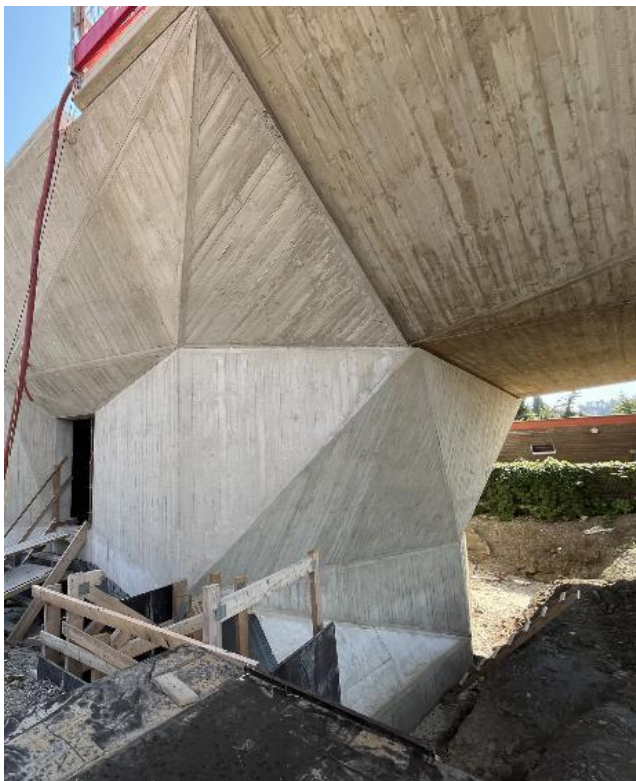
Figure 14: Shaping of abutment O7
