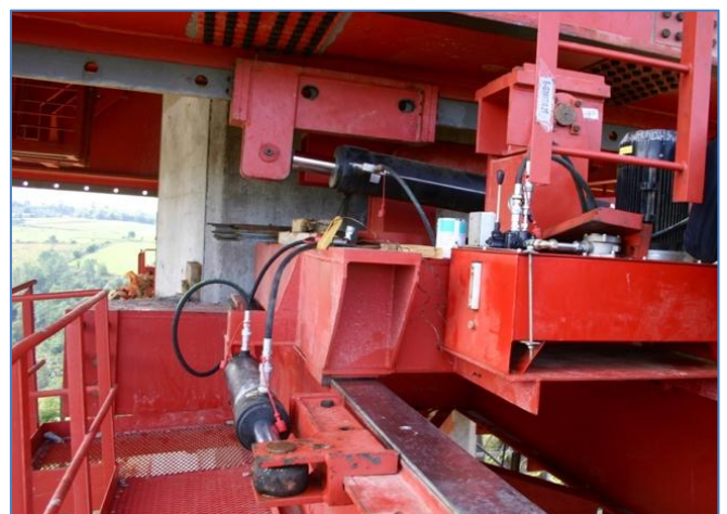
Figure 3: MSS launching subsystem
