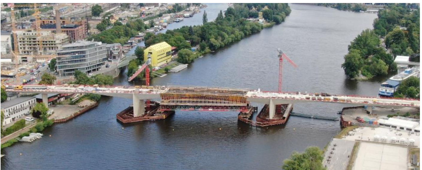
Figure 33: Construction of the central part of the main span
