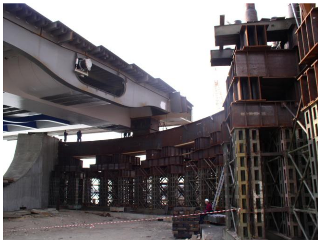
Figure 16: Turning the bridge - a view of the quarter-circle slideway. Photo Credit P. Paulík
