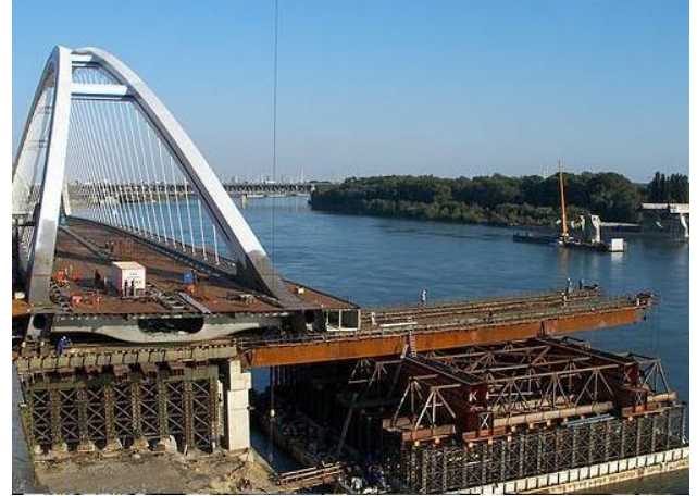
Figure 15: Sliding the bridge from temporary pier onto the vessel – aerial view. Photo Credit: M. Pokorný
