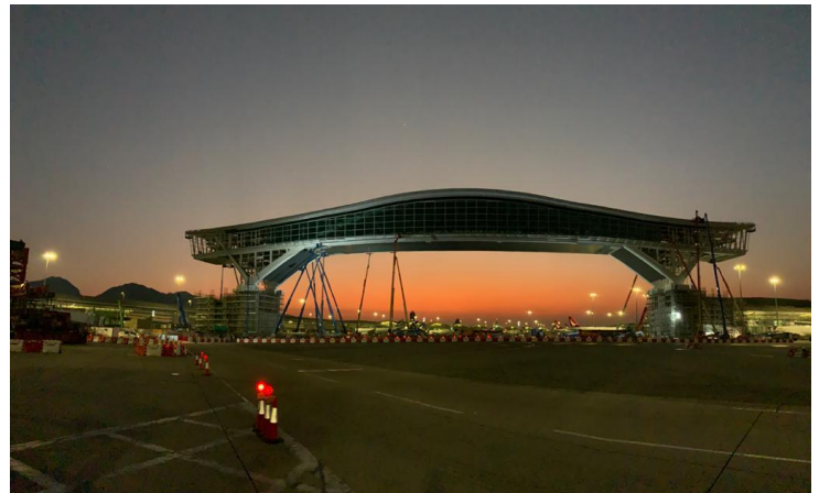
Figure 6: Installation of the bridge in its final position
