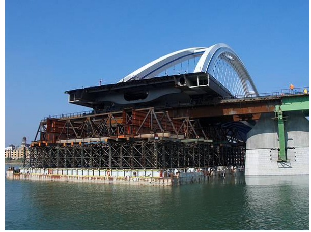
Figure 19: The bridge reached the pier Photo Credit M. Pokorný
