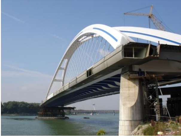
Figure 18: Turning the bridge. Photo Credit P. Paulík
