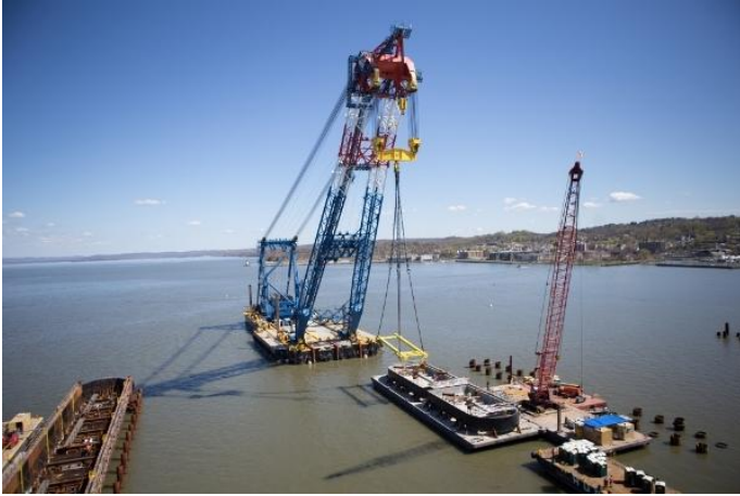
Figure 11: Moments before raising a pair of precast pile caps, each weighing 550 tons
