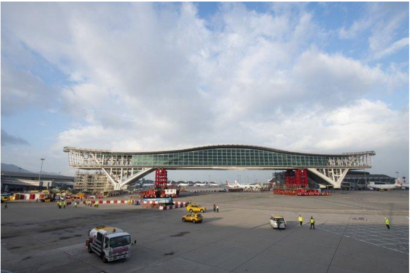
Figure 1: Transportation of the bridge using Mega Jack 5200 system Photo Credit: Hong Kong International Airport (HKIA)
