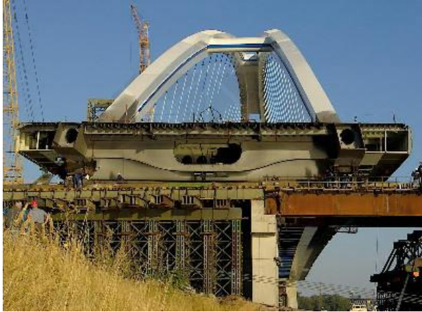
Figure 14: Sliding the bridge from temporary pier onto the vessel – view from the riverbank. Photo Credit M. Pokorný
