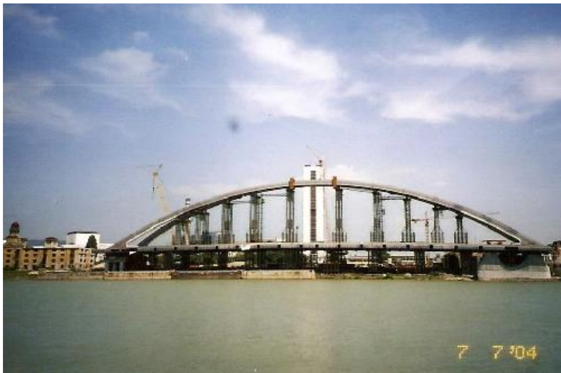
Figure 9: Assembly of the arch with individual parts on steel supports Photo Credit: P. Paulík
