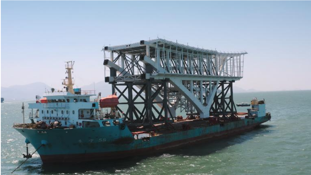
Figure 2: Transportation of the bridge at sea. Photo Credit HKIA
