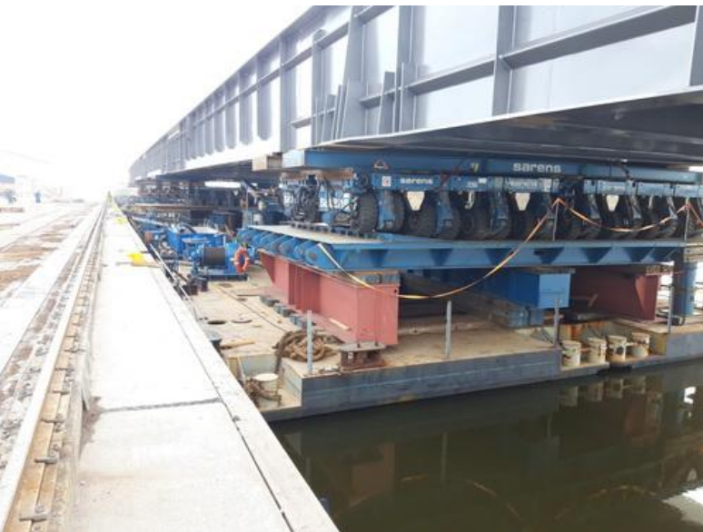
Figure 9: SPMT on a barge during installation of the new bridge
