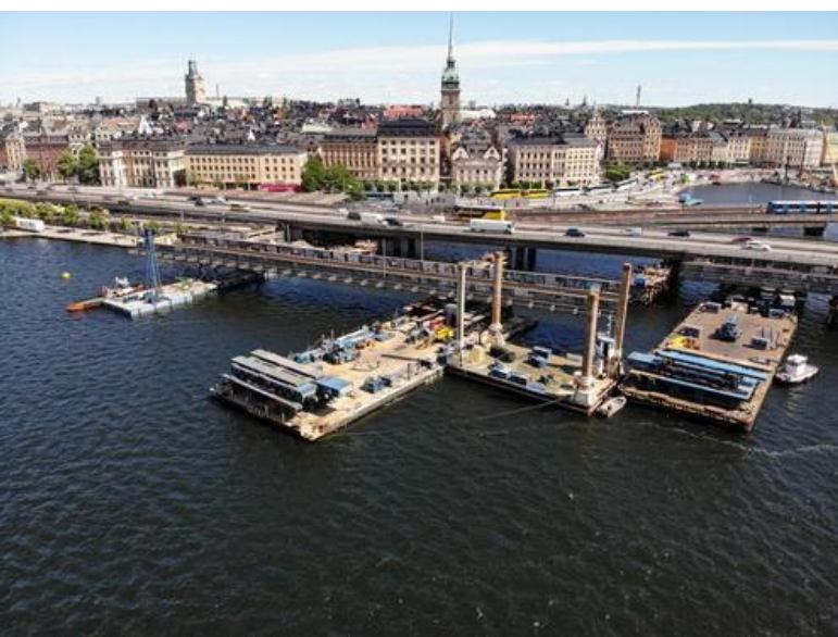
Figure 5: Removal of the old bridge
