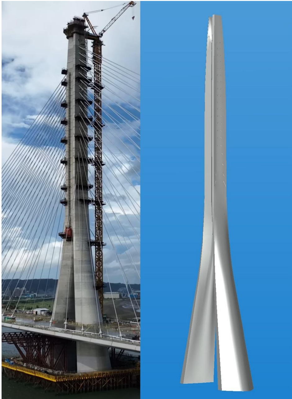
Figure 21: Original rendering and similar view of pylon under construction
