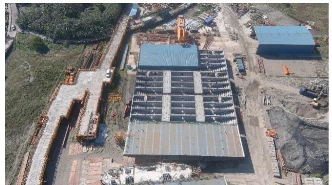
Figure 17: Deck segment assembly on site
