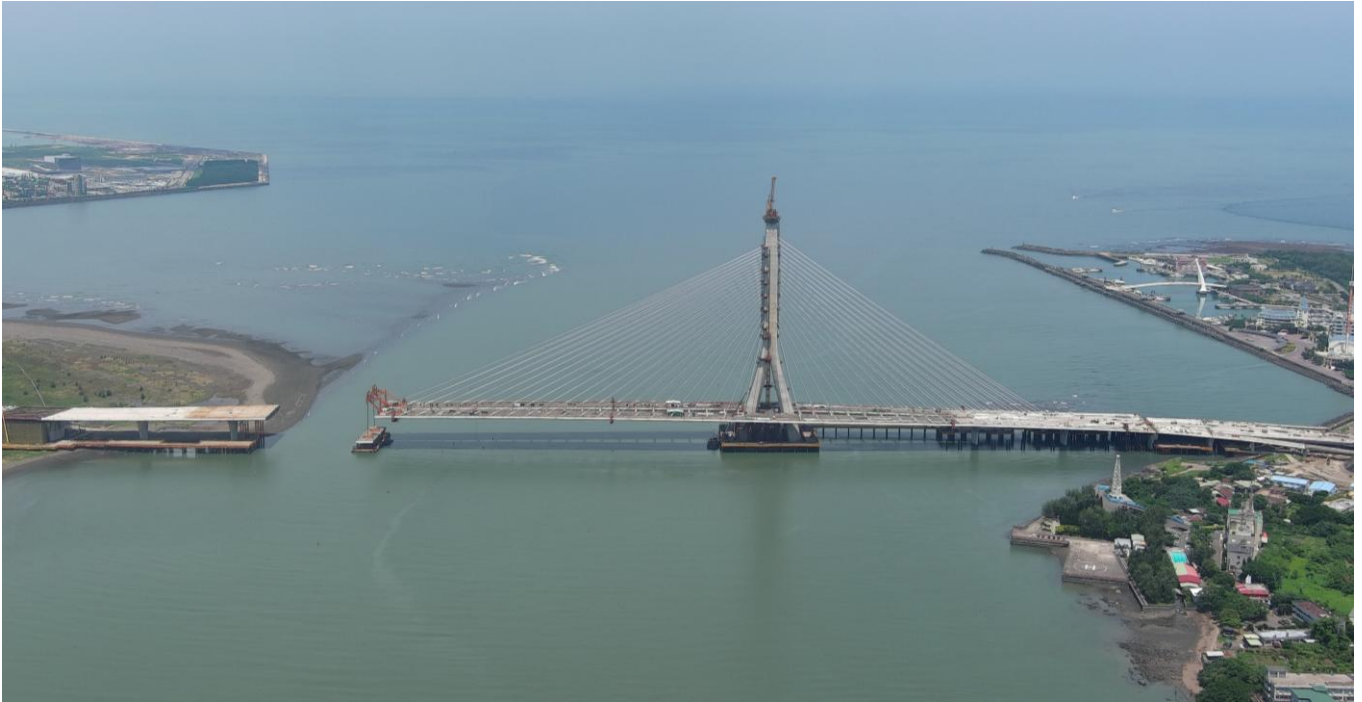
View of the Bridge
