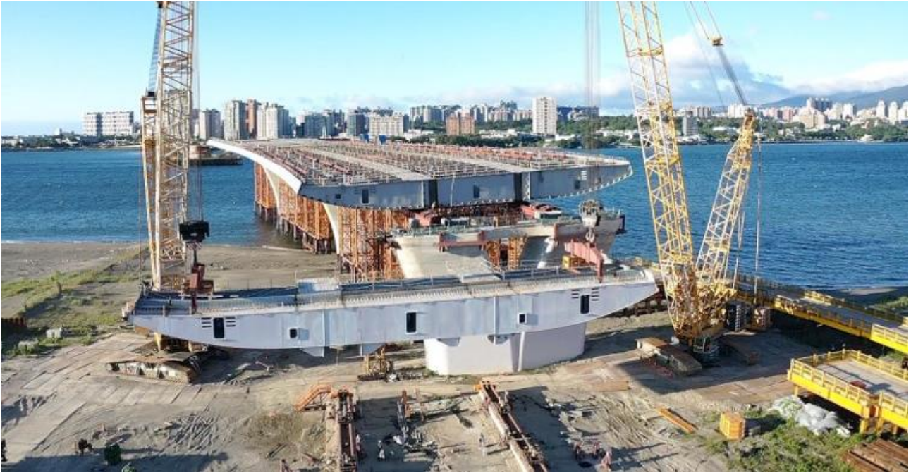
Figure 23: Bali side span installation
