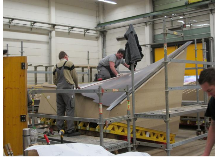
Figure 3: Warped formwork panel prepared at workshop
