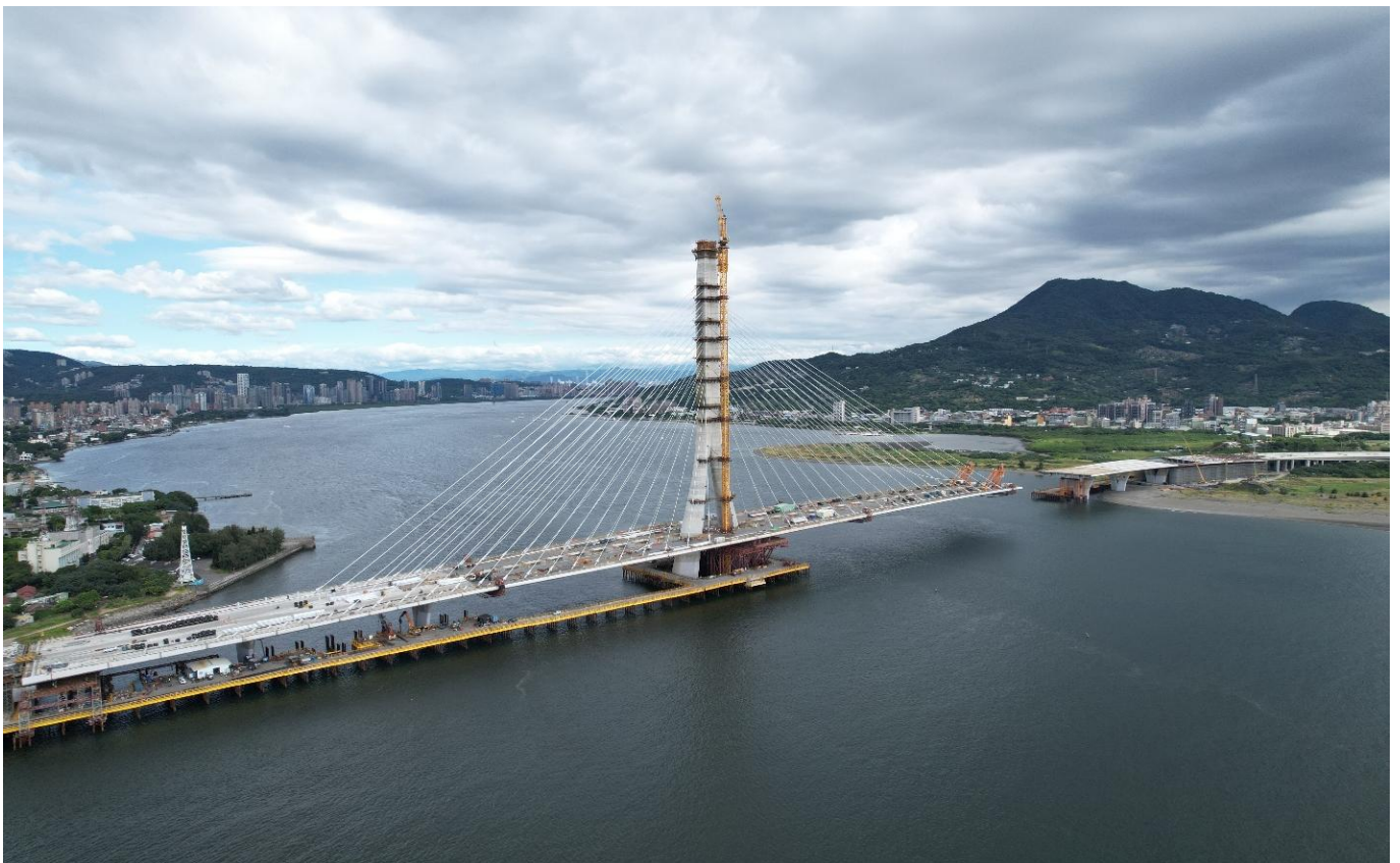
Figure 26: Free cantilever deck erection
