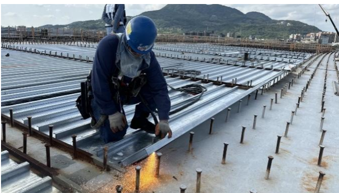
Figure 24: Formwork panels of composite slab
