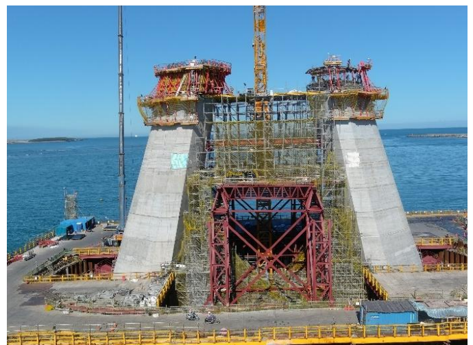
Figure 20: PERI SCS climbing form at pylon legs
