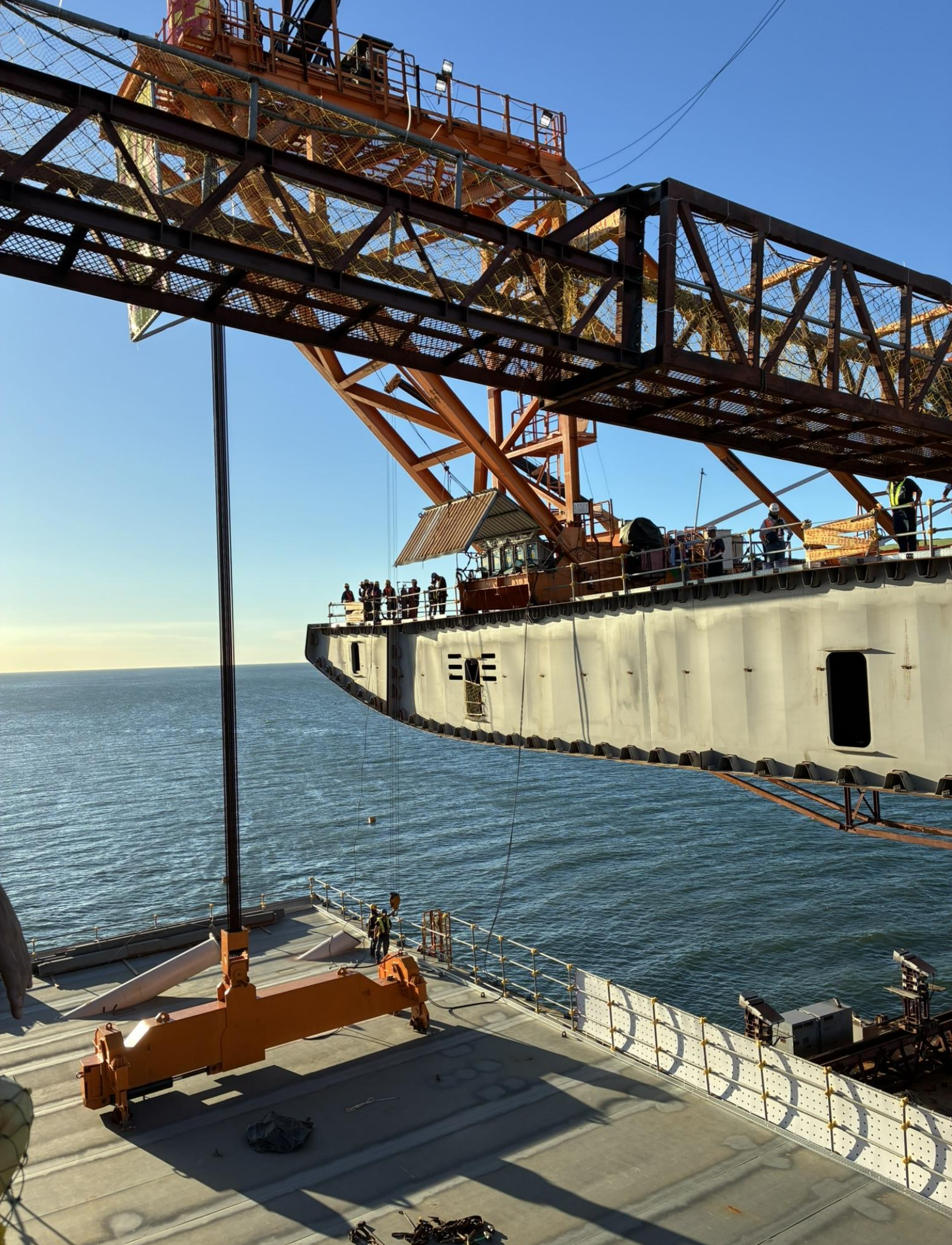
Danjiang Bridge Main Span Closure on 16 th September 2025
