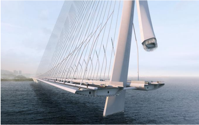
Figure 7: The deck and pylon sections
