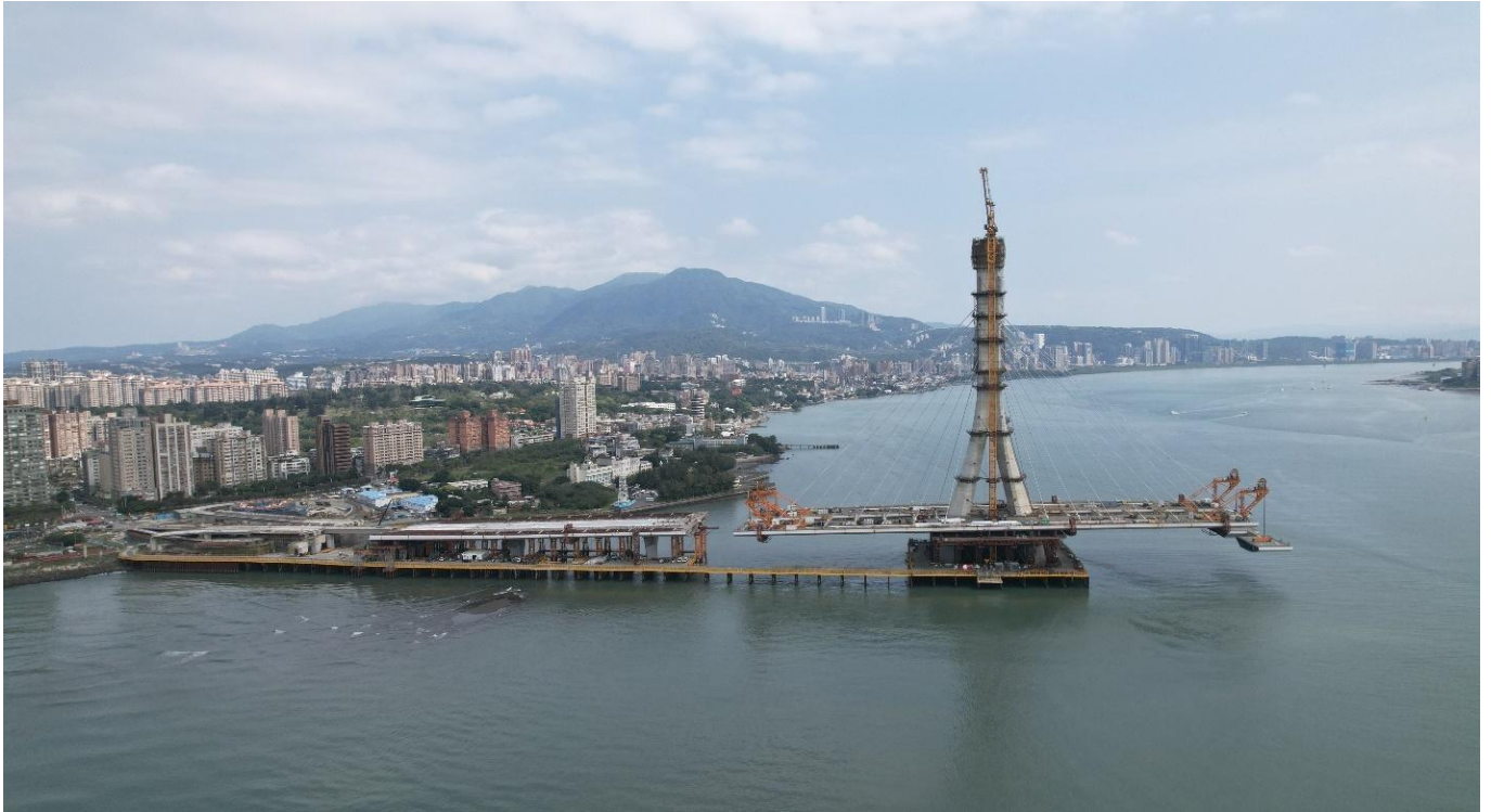
Figure 25: Balanced cantilever deck erection
