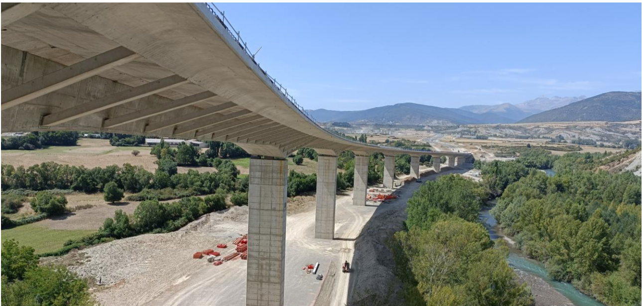
Figure 1: Bottom view of the viaduct with a foreshortened view from pier P1
