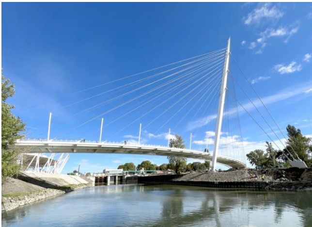
Figure 56: Robinson Bridge from the waterfront
