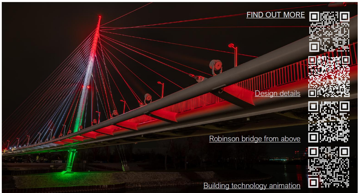
Figure 67: The Robinson Bridge with decorative lighting
