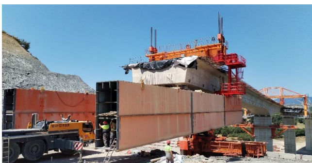
Figure 48: Incremental launching for Main Girders disassembly after completion of last span with MSS – last steps
