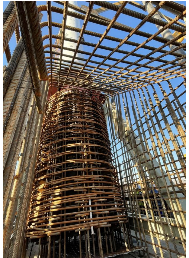
Figure 43: Pylon foundation
