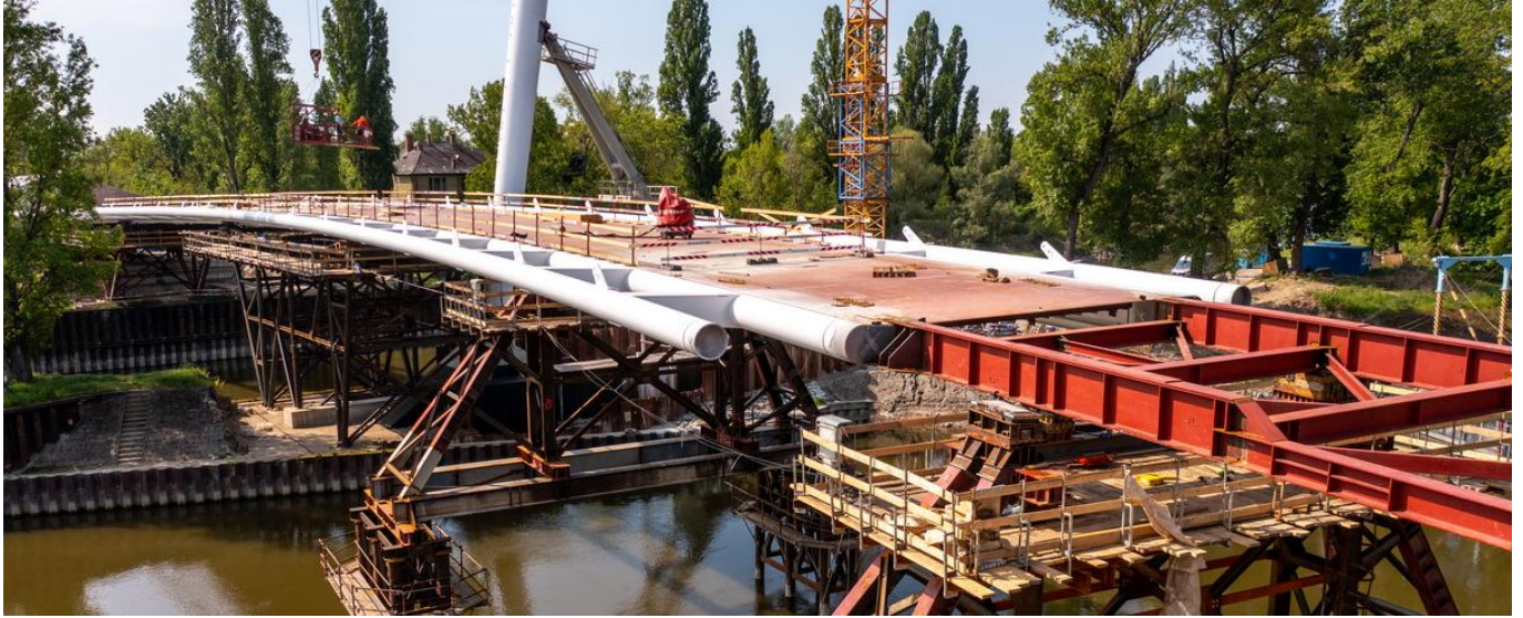
Figure 48: Deck launching on temporary supports
