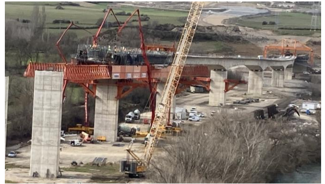
Figure 13: General view of the deck construction, with the MSS and the wing traveller
