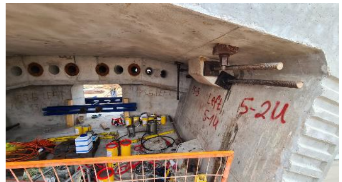
Figure 22: Temporary post-tensioning bars used to fix a newly erected segment to the adjacent segment before permanent stressing
