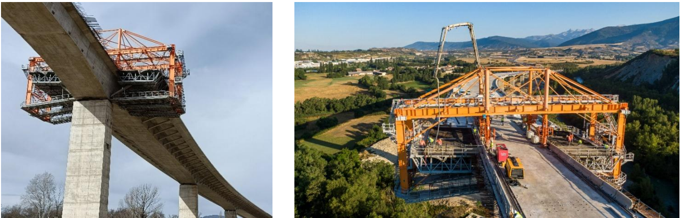
Figure 19: Left: Bottom view of the wing traveller. Right: Upper view of the wing traveller
