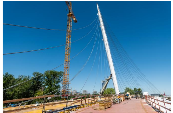
Figure 49: Before cable tensioning
