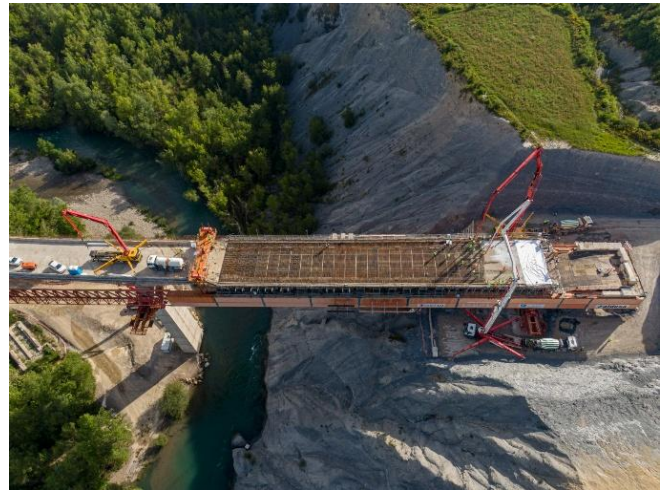
Figure 16: Aerial view of the deck during the execution of the top slab (span 1)
