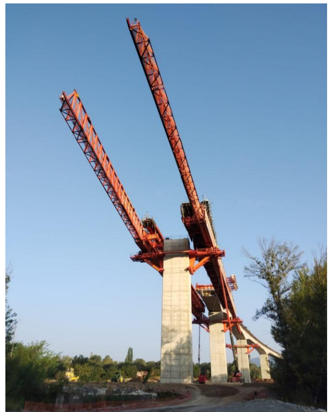
Figure 1: Sabiñánigo Movable Scaffolding in transition between spans
