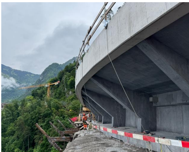
Figure 6: The completed retaining structure follows the curved road alignment through the steep terrain above Lake Lucerne. Copyright: Bänzinger Partner
