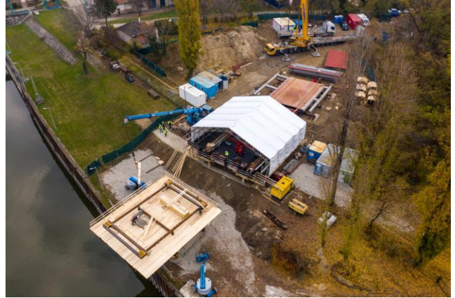
Figure 45: Deck fabrication on site
