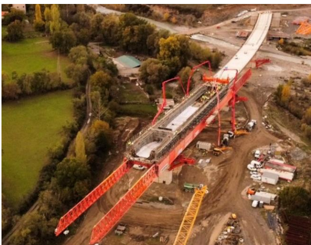
Figures 14 and 15: Views of the deck during the concreting of the U-shaped partial section
