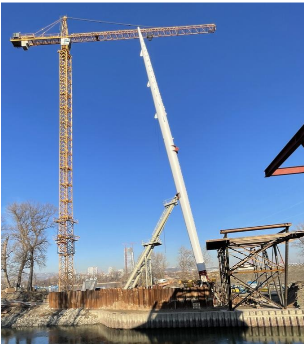
Figure 42: Pylon in temporary support
