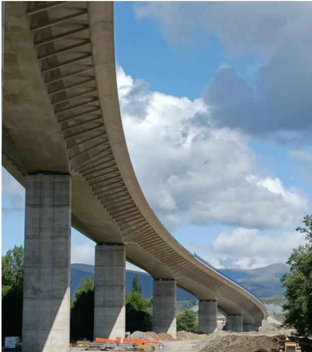
Figure 7: Bottom left and right: Bottom views of the deck that show the warping of the prefabricated strut's plane. Top right: prefabricated strut assembled on site
