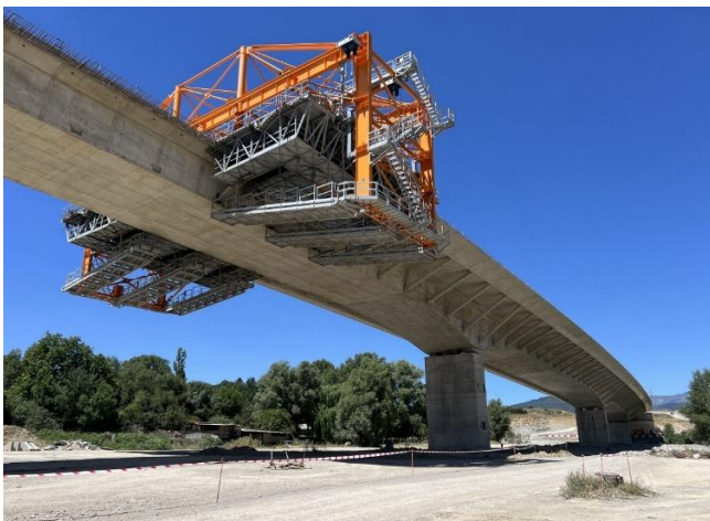
Figure 14: Wing traveller for cantilever slab execution
