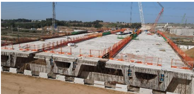
Figure 23: A view of the abutment of the bridge during construction
