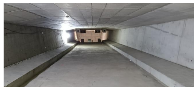
Figure 22: Interior view of the deck including the enlarged corners
