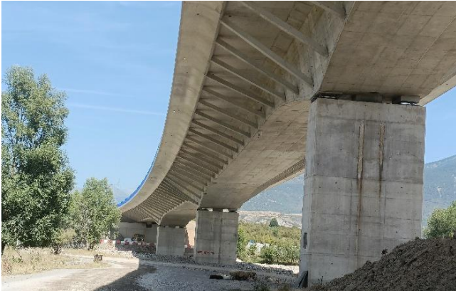
Figure 5: Left: Bottom view of the depth variation. Right: MSS during concreting of the upper slab of a typical span of 90 m
