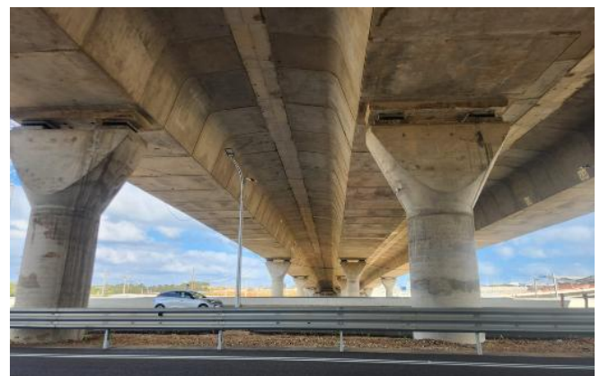
Figure 24: Completed BR-541 bridge viewed from below after opening to traffic. The final structure presents a continuous segmental deck supported by slender piers, combining structural efficiency, constructability and a clean architectural expression
