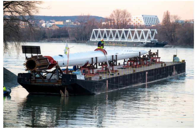
Figure 36: Pylon transport on barge
