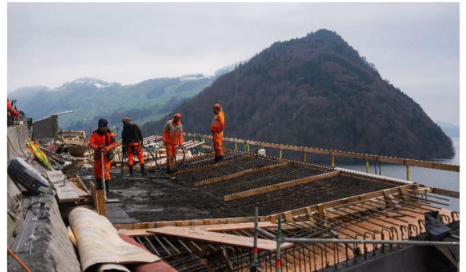
Figure 5: Construction of the reinforced concrete road deck in the challenging terrain above Lake Lucerne. Copyright: Bänzinger Partner
