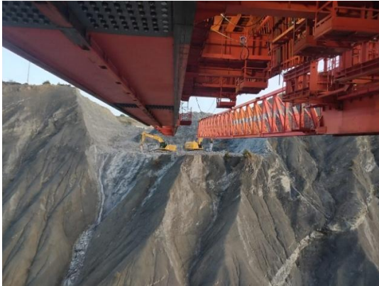
↑ ↗ Figures 45 and 46: Launching to Stage 10
