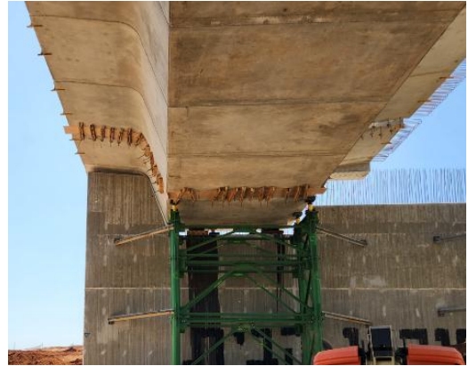
Figure 21: Closure pour at the end segment, showing the interface between precast segmental units and in-situ closure concrete
