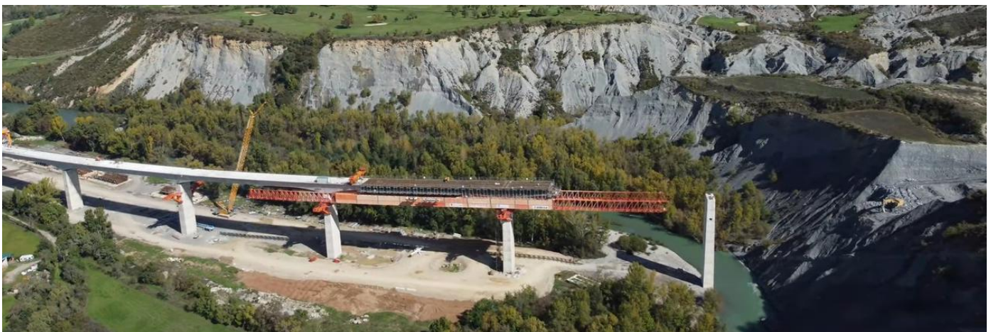
Figure 18: Aerial image during the reinforcement of the top slab
