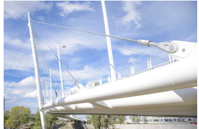
Figure 21: Stay cable joint
