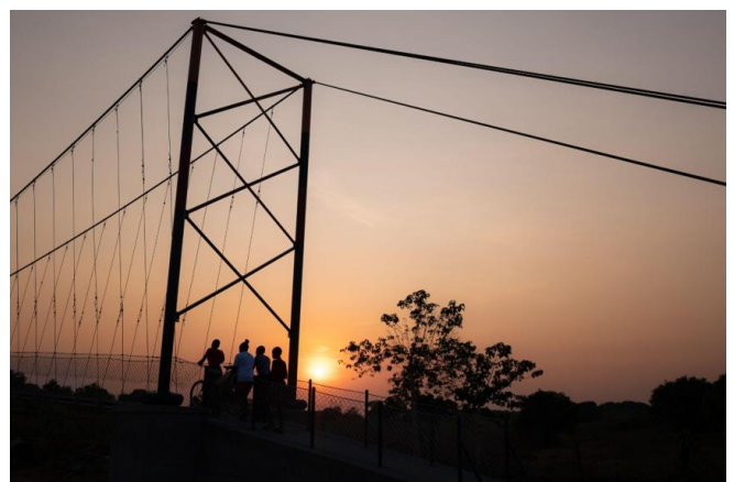
Figure 3: Kasenga Bridge – Zambia Photo Credit: Robb Hohmann
