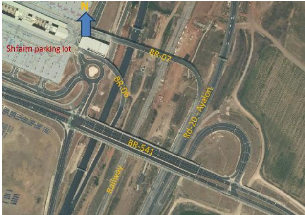
Figure 2: Aerial view of the BR-541 crossing within the Fast Lanes Shfaim corridor. The bridge crosses a dense transport zone containing Ayalon Road, existing railway tracks, planned railway facilities and major utility infrastructure.
