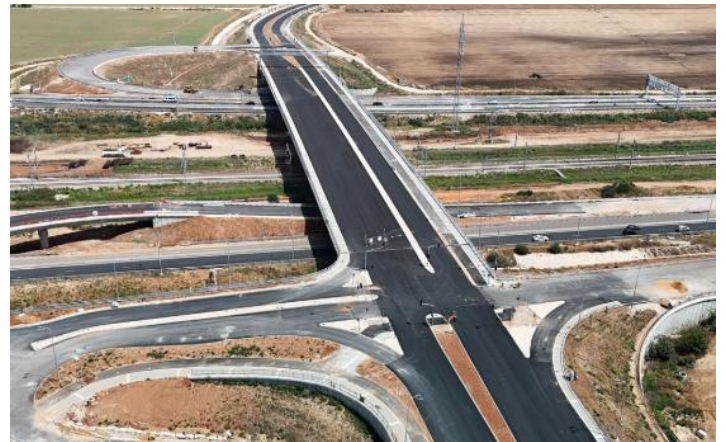
Figure 3: Plan view of the completed BR-541 bridge after opening to traffic
