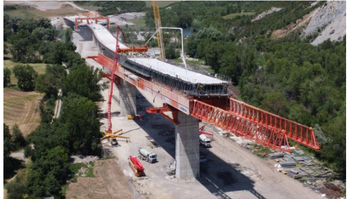
Figure 5: Left: Bottom view of the depth variation. Right: MSS during concreting of the upper slab of a typical span of 90 m
