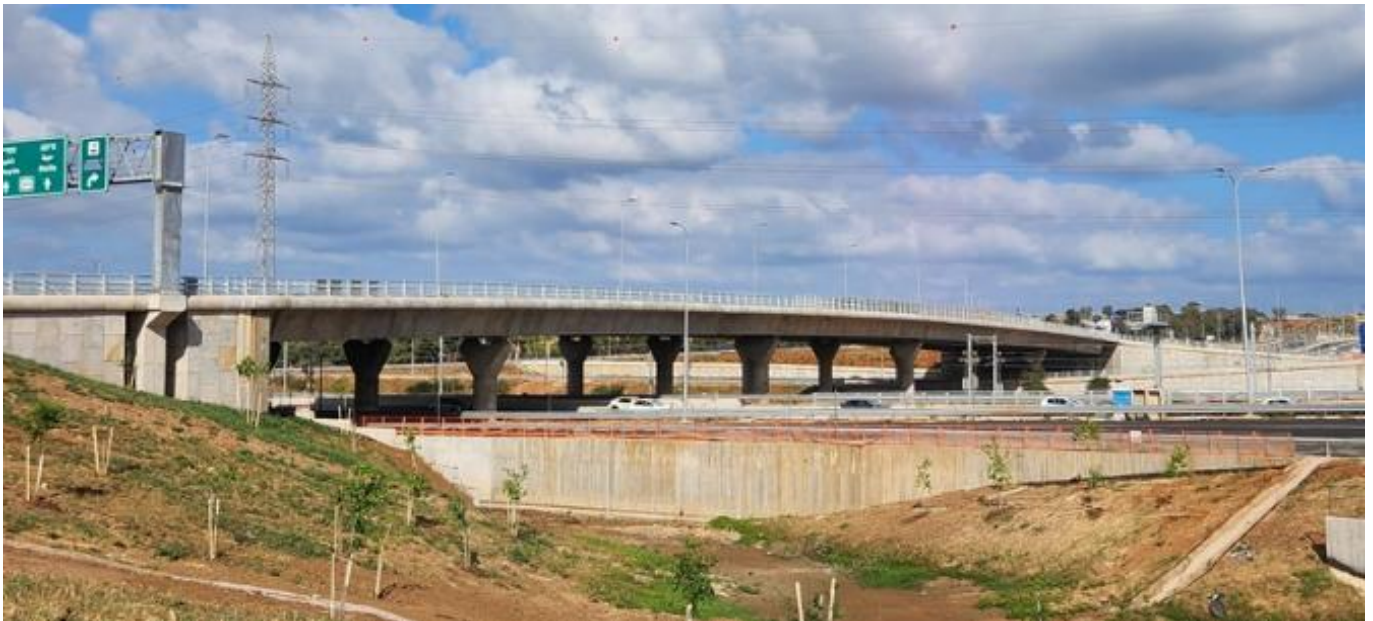
Figure 1: General view of the completed BR-541 bridge after opening to traffic
