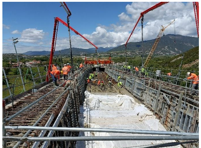
Figures 14 and 15: Views of the deck during the concreting of the U-shaped partial section
