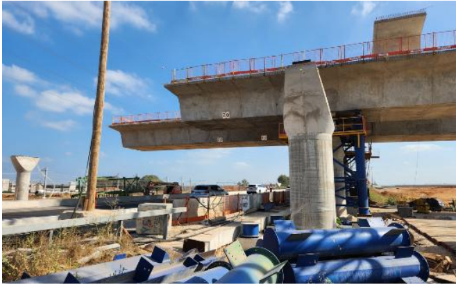
Figure 20: Construction view at a pier segment during balanced cantilever erection. The photograph shows the scale of the precast segmental units and the close relationship between the superstructure, substructure and restricted working area
