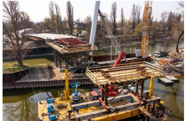
Figure 46: Deck launching on temporary supports
