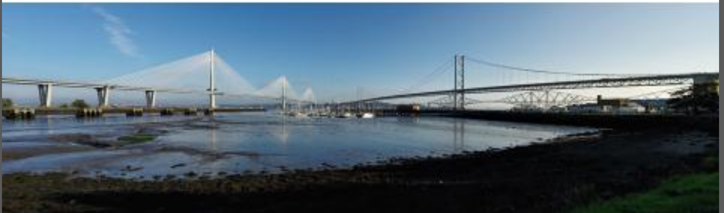
Queensferry Crossing Scotland
