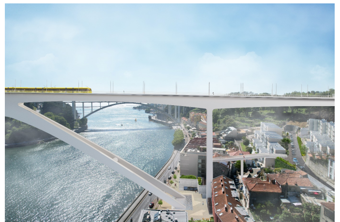
Figures 18 and 19: The Bridge is located in an inhabited area of Porto. View of the abutments on both sides of the Douro River
