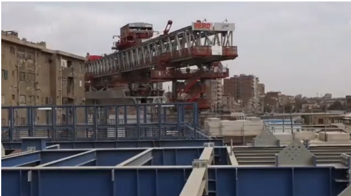
Video: BERD’s LG 36 at Phase 3 of Line 3 of the Greater Cairo Metro. Credit: National Authority for Tunnels, Egypt
