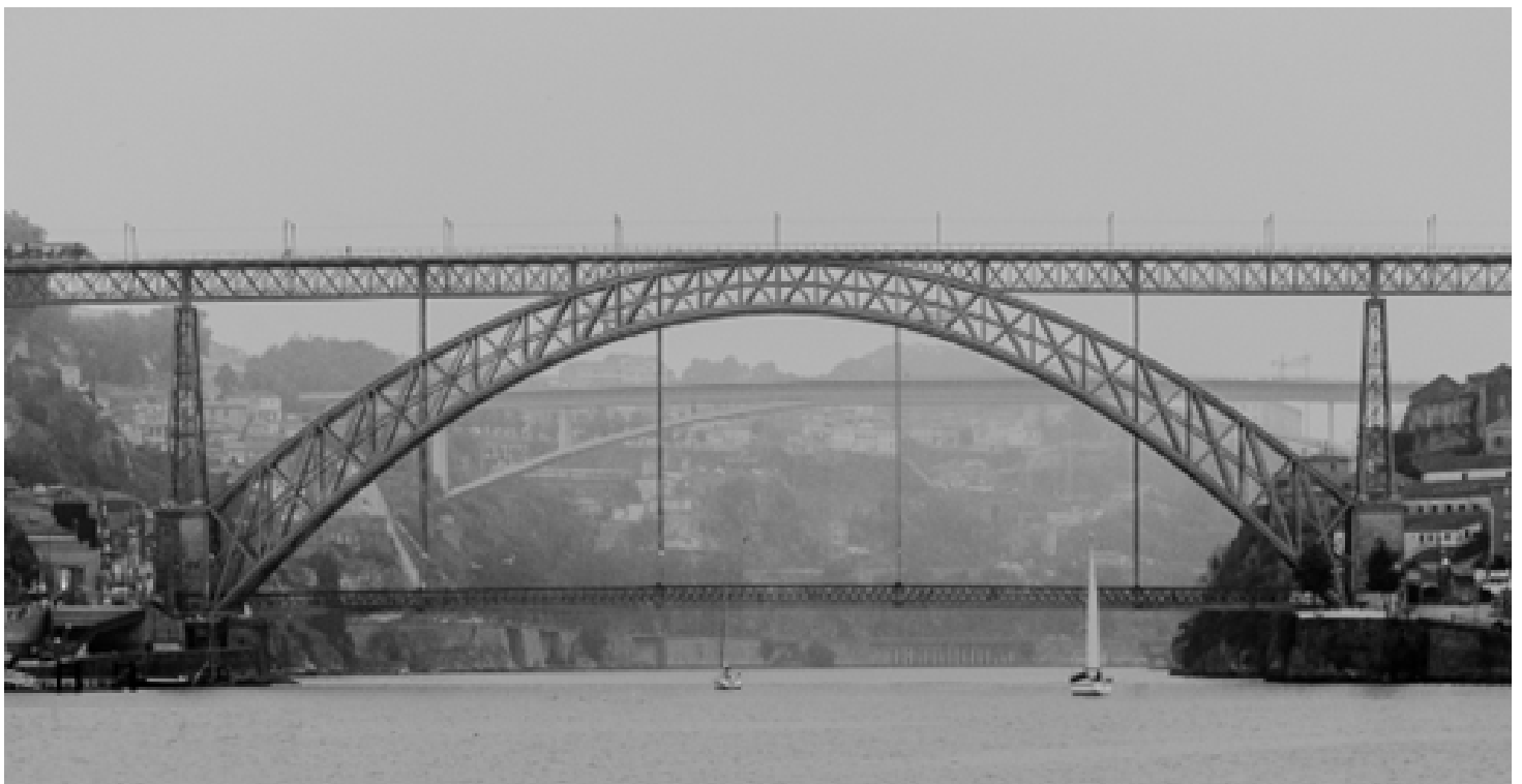
Figure 4: Luis I. Bridge
