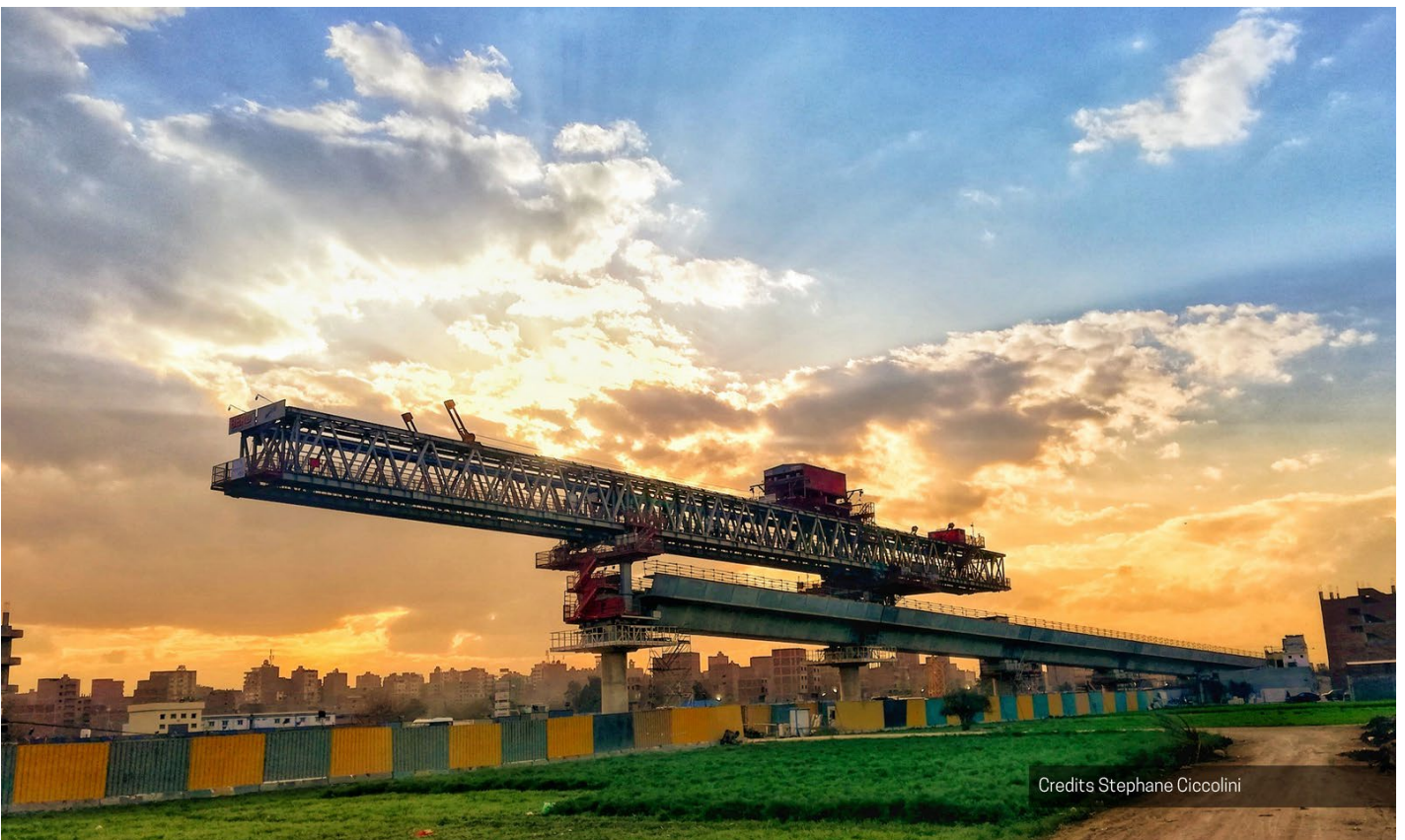
Figure 1: Launching Gantry in operation
