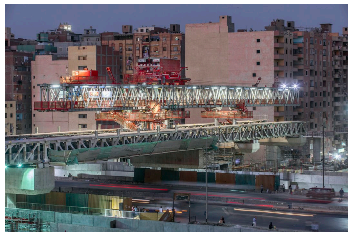
Figure 9: LG special operation crossing over the Ring Road
