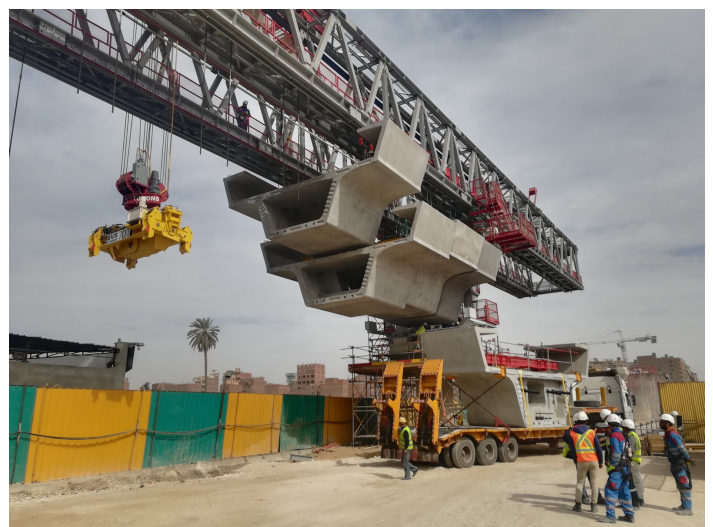
Figure 11: Transportation of segments from a truck
