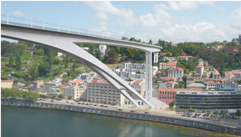
Figure 8: The new bridge will be 75 m high
