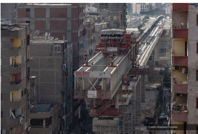
Figure 8: The construction site in the close vicinity to buildings
